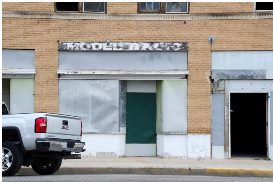
Photo 7: West elevation, storefront, looking east
