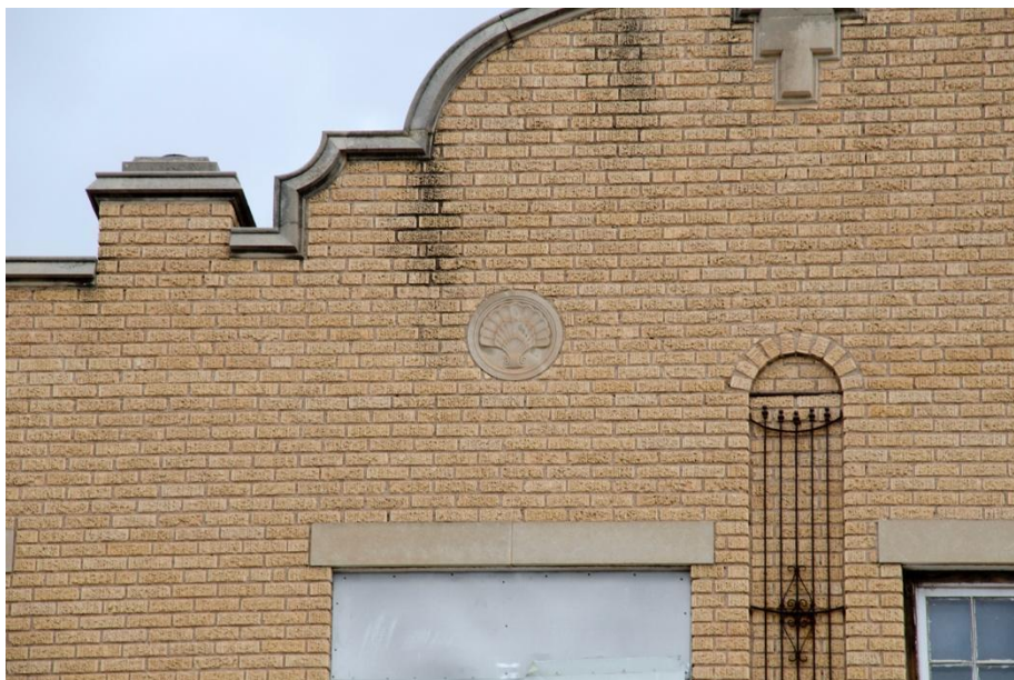
Photo 9: Masonry detail, west elevation, looking east
