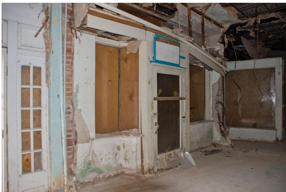
Photo 10: Interior storefront entrance, looking west
