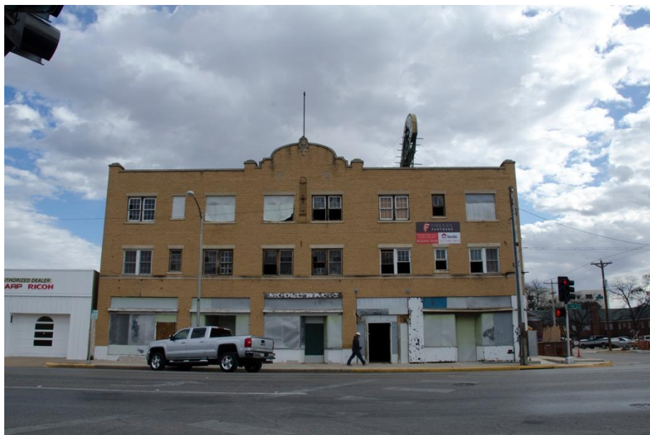
Photo 1: West elevation, looking east
