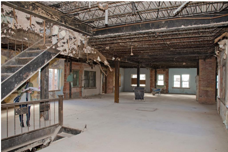
Photo 14: Interior, second floor, looking southeast
