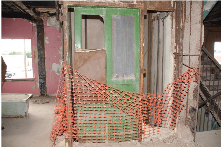
Photo 13: Elevator, second floor, looking south
