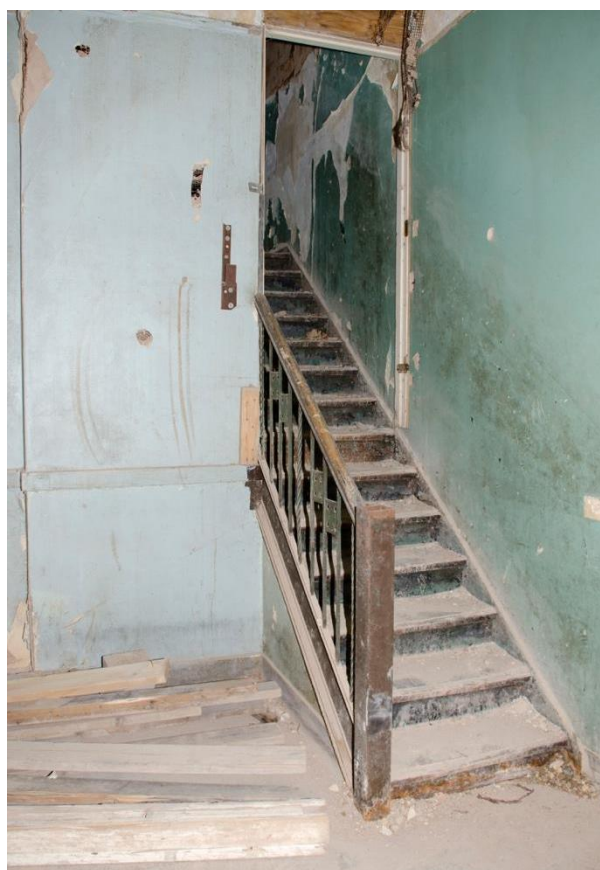
Photo 12: Central stair, first floor, view southwest
