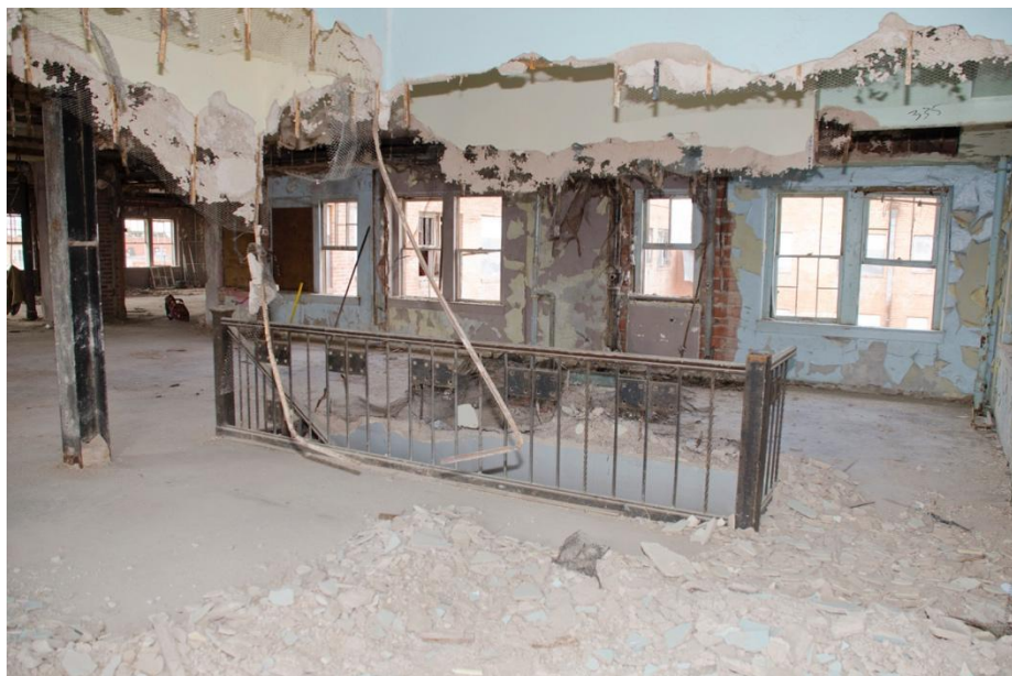
Photo 15: East stair, third floor, looking southwest
