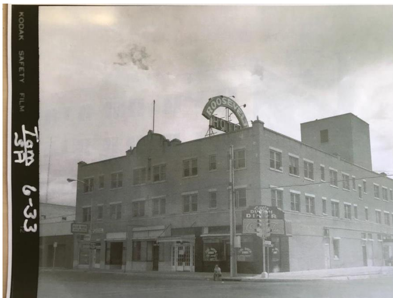
Figure 8: Roosevelt Hotel, looking northeast, Historic Photo – Undated
