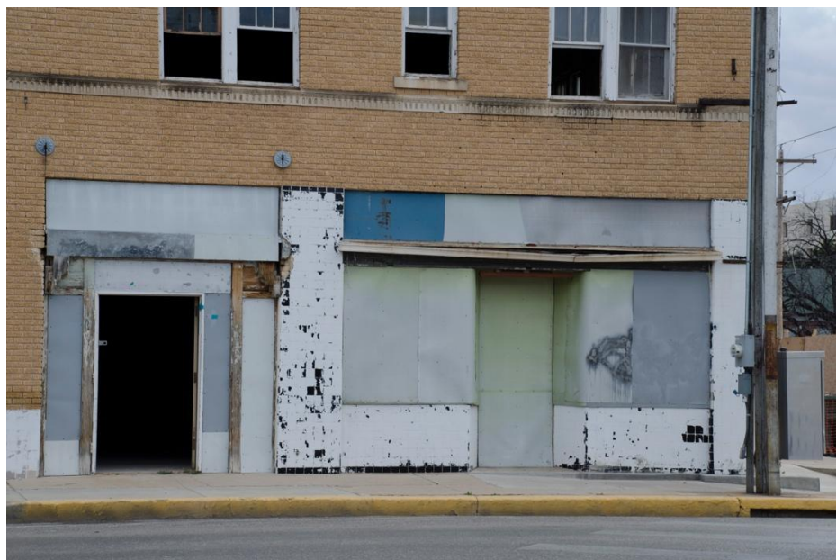
Photo 8: West elevation, storefront, looking east
