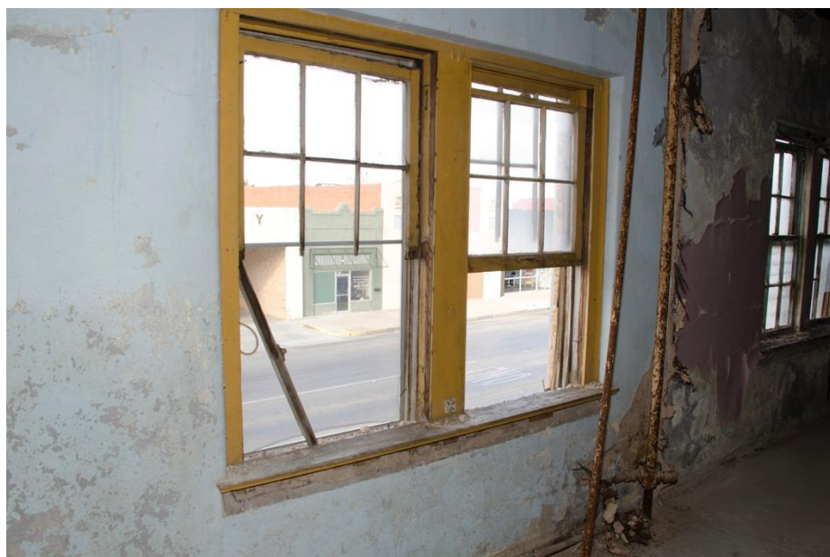
Photo 16: Window detail, second floor, looking northwest
