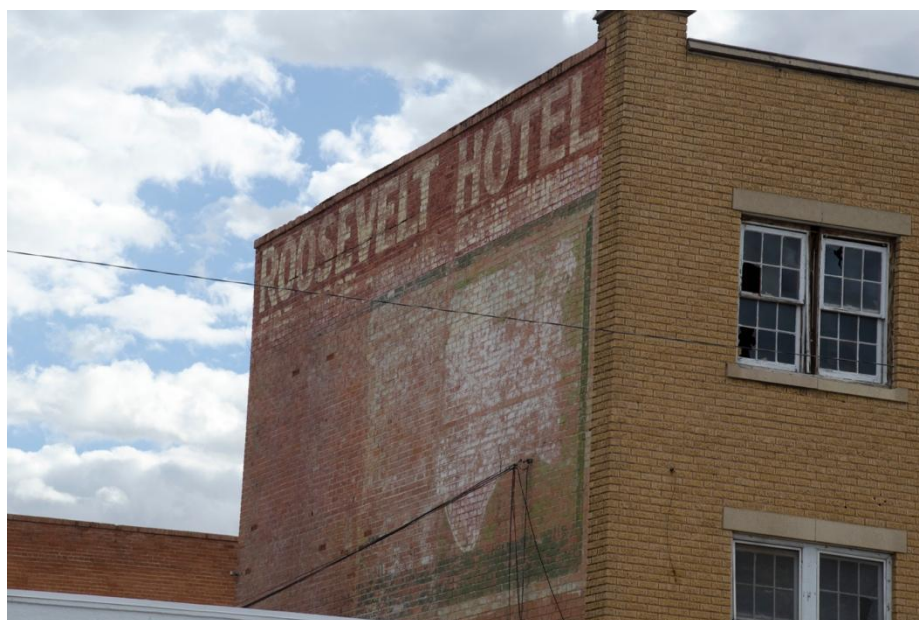
Photo 6: North elevation with ghost sign, looking southeast
