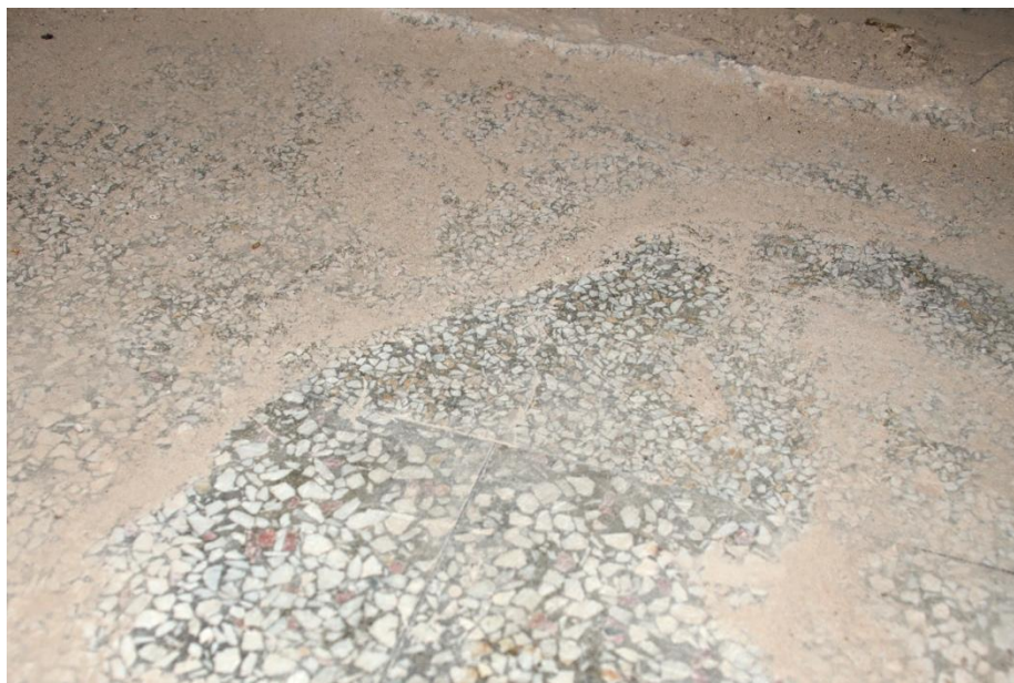
Photo 11: First floor, detail of terrazzo flooring
