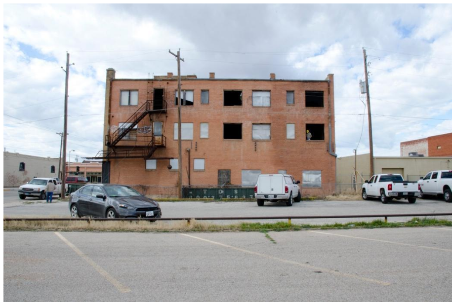
Photo 4: East elevation, looking west
