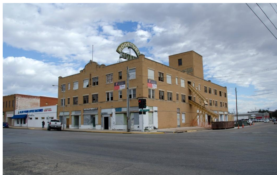
Photo 2: West and south elevations, looking northeast
