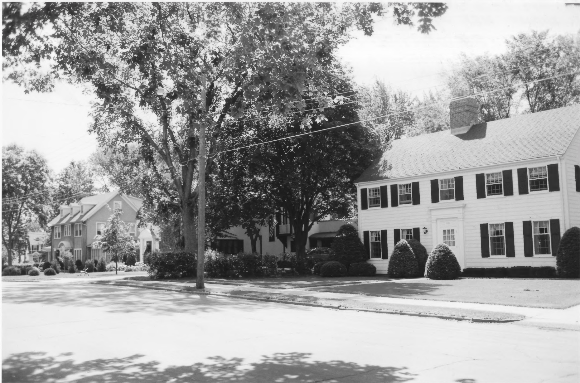
LEFT: 1014-7 TH ST. SW, CENTER: 1104-7 TH ST. SW, RIGHT: 1120-7 TH ST. SW (CNC) PILL HILL RESIDENTIAL HISTORIC DISTRICT ROCHESTER, OLNSTED CO., MINNESOTA
