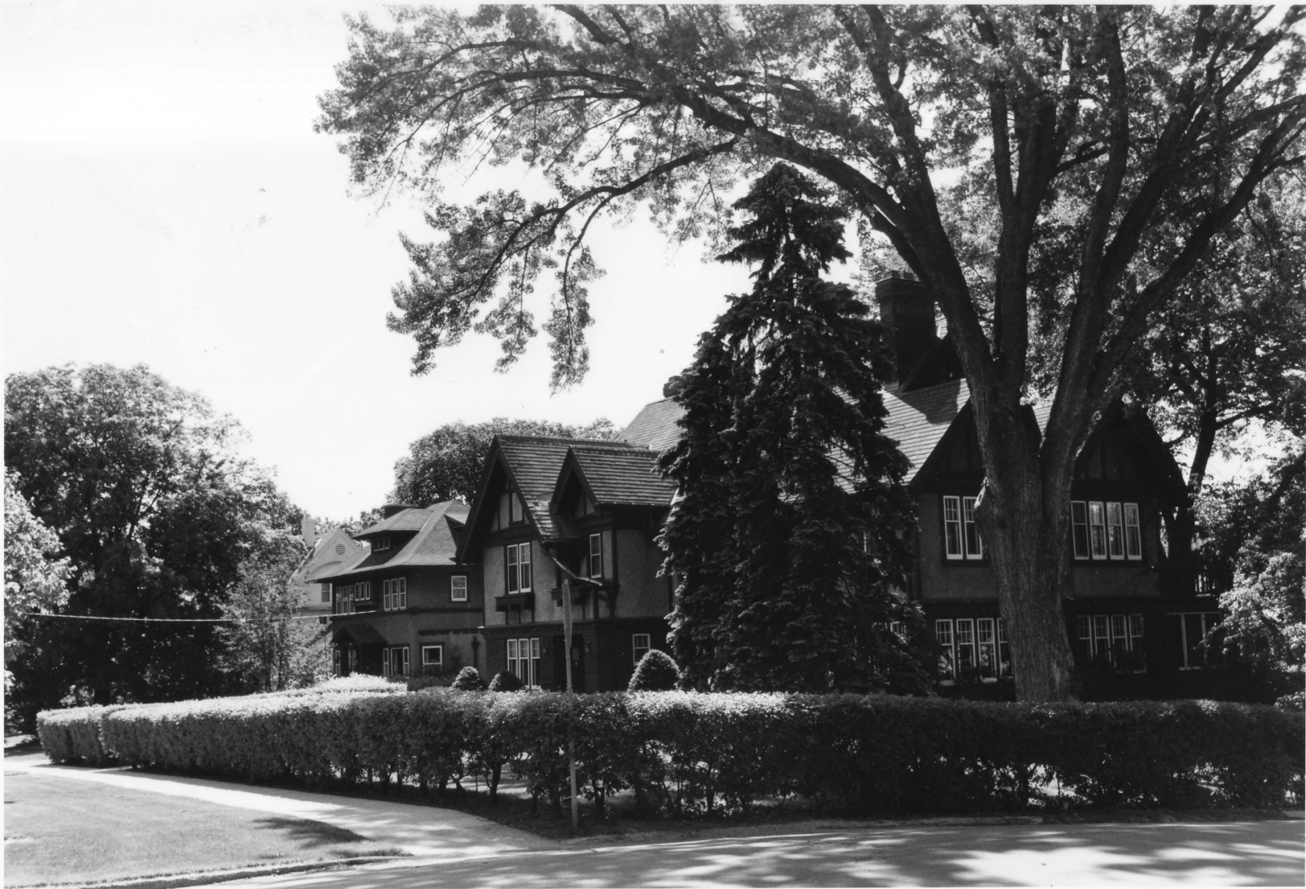
Pill Hill Historic District streetscape along 4 th St / FAR LEFT: 716 4 th St. SW, CENTER: 720 4 th St. SW, Rochester, MN RIGHT: 724 4 th St. SW 07824-6
