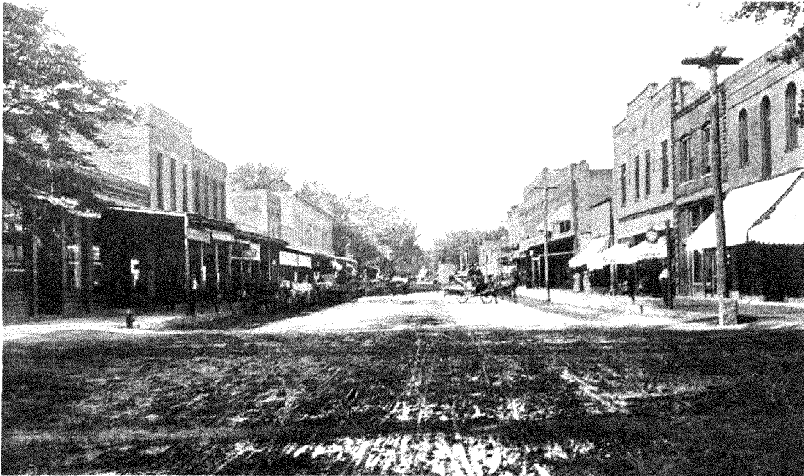
Figure 7 – Looking south on Douglas Avenue from 2 nd Street, c.1905
