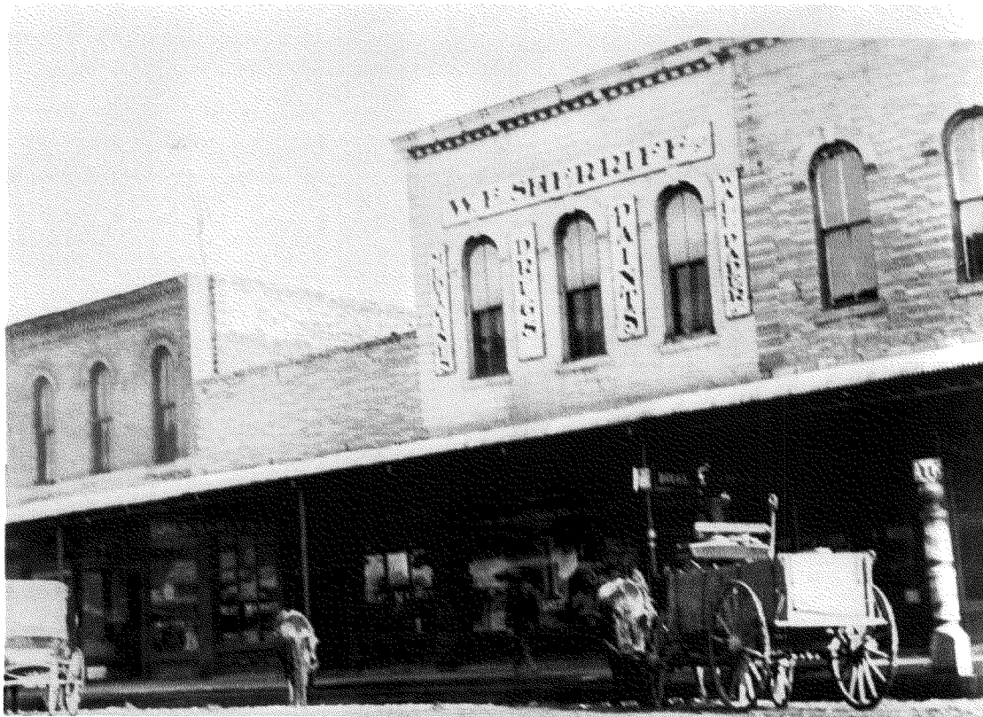
Figure 9 – East side of 200 block N. Douglas Avenue mid-block c.1900
