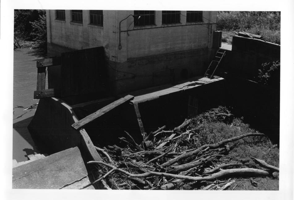
Photo #13 DEC 2 7 1978 DeWitt Flour Mills and King Iron Bridge Gage County, Nebraska Photo by D. Murphy, Nebraska State Historical Society, July 1978 DEC 6 1978 NSHS # 7807/3:23 DEC 6 1978 View of the base of the electric power house showing inlet and outlet flumes; looking southeast. 7807/3:23
