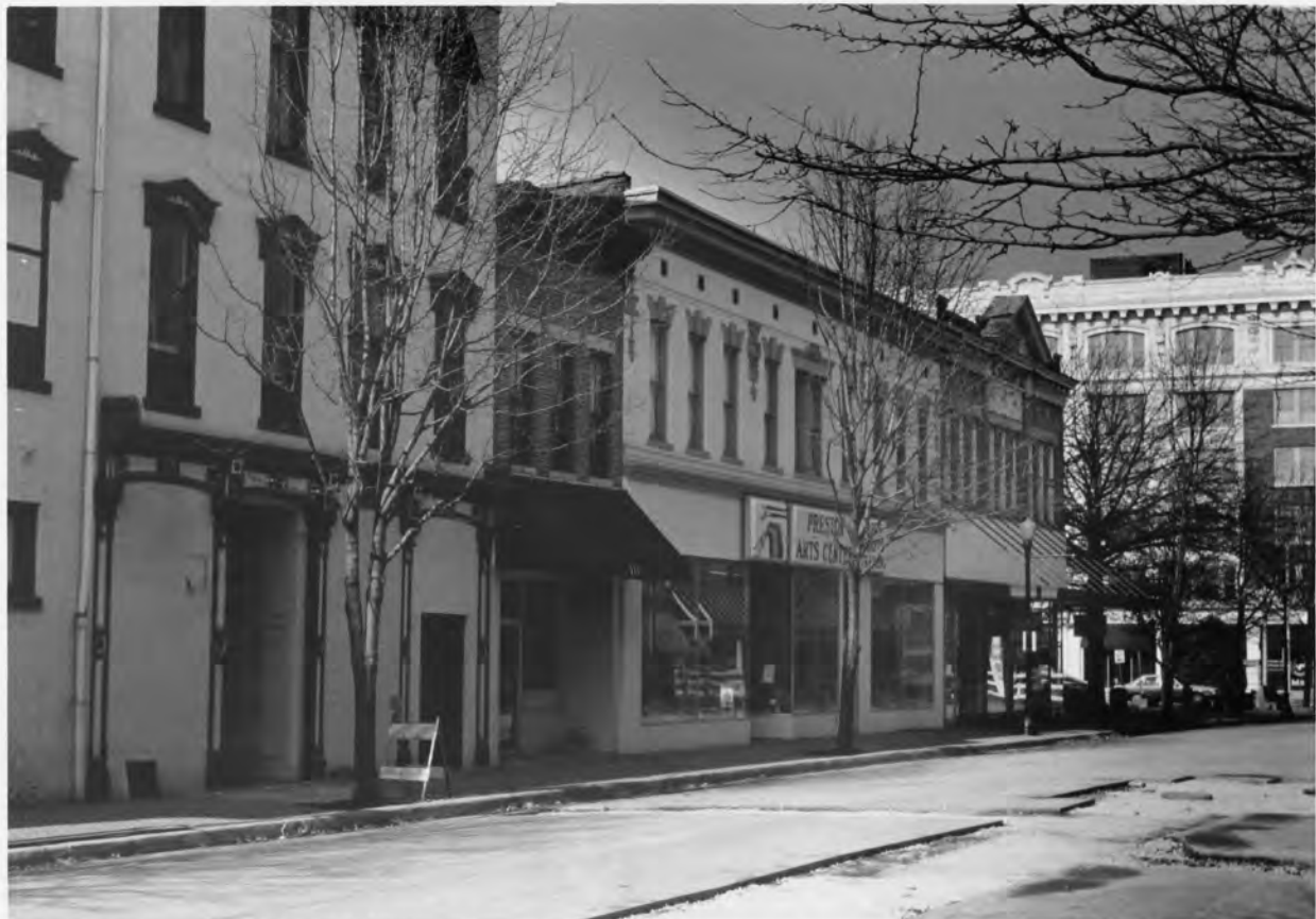
W. SIDE PEARL ST., NEW ALBANY DOWNTOWN HIST. DIST., FLOYD CO., IN, PHOTO NO. 10
