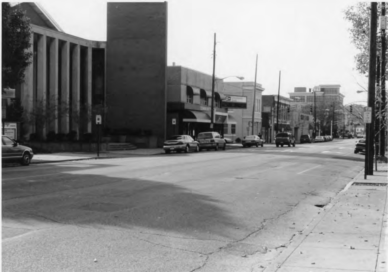
222 E. SPRING ST., NEW ALBANY DOWNTOWN HIST. DIST., FLOYD CO., IN, PHOTO NO. 2
