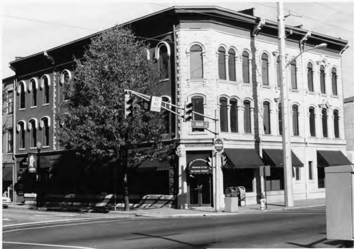
202-204 PEARL ST., NEW ALBANY DOWNTOWN HIST. DIST. ROYDCO., IN, PHOTO No. 28
