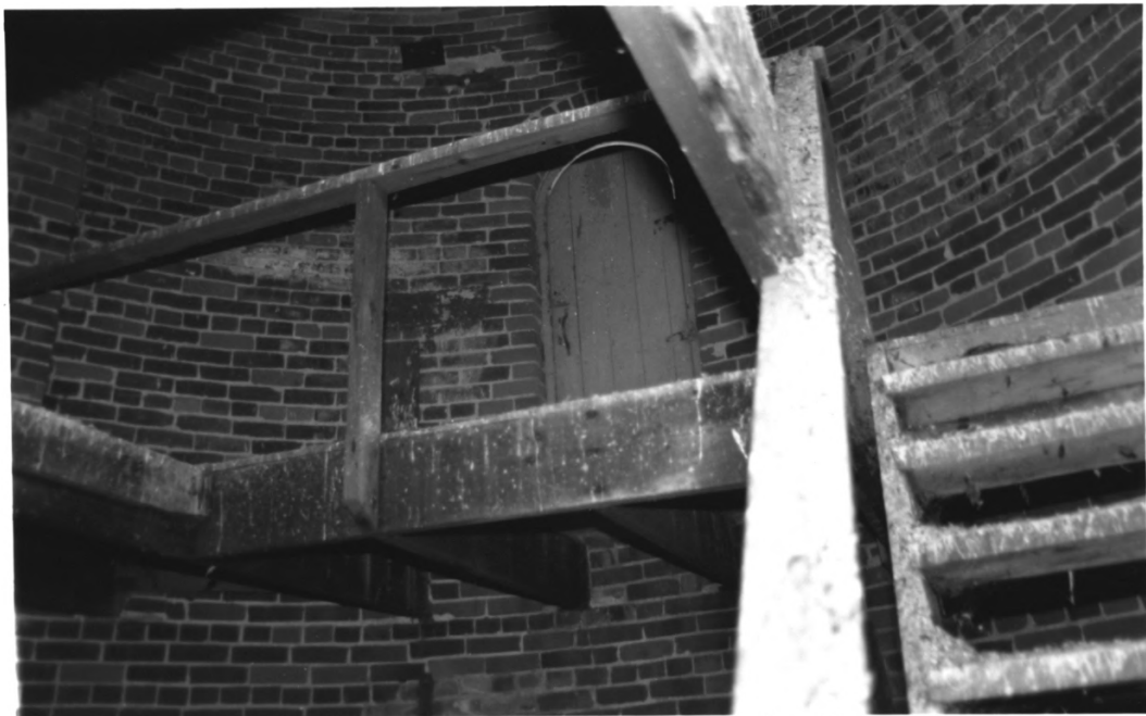
Remington Water Tower, Jasper Co, IN
