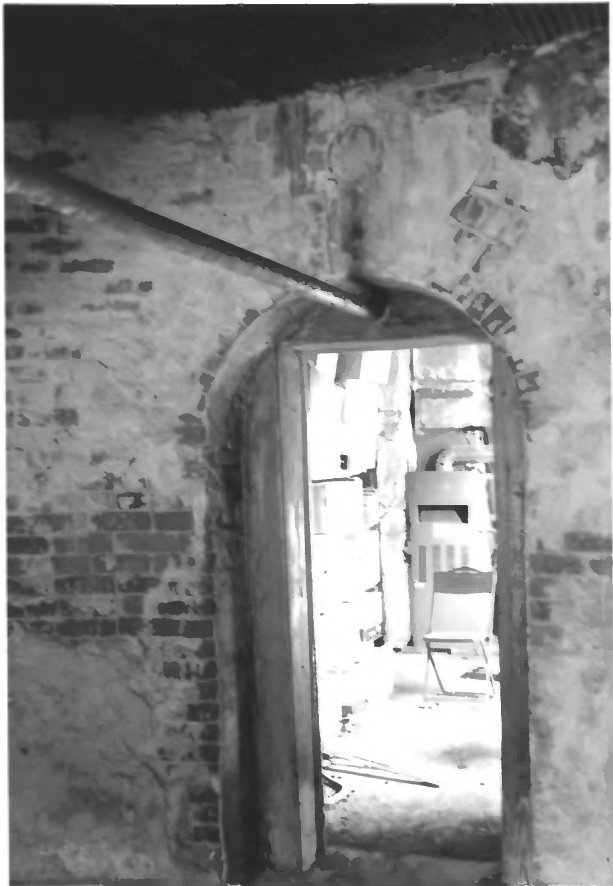
Remington Water Tower, Jasper Co, IN, #17
