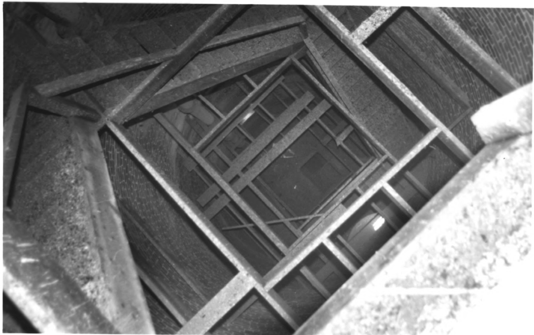
Remington Water Tower, Jasper Co, IN
