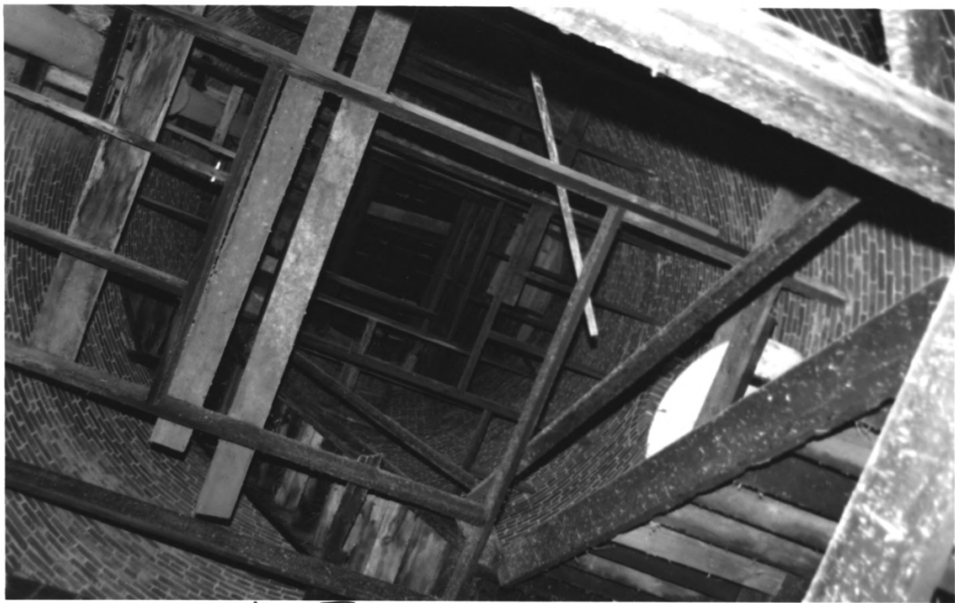
Remington Water Tower, Jasper Co, IN
