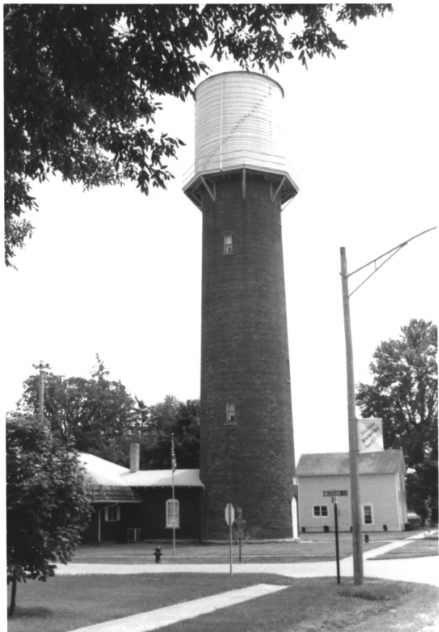
Remington Water Tower, Jasper Co, IN #1
