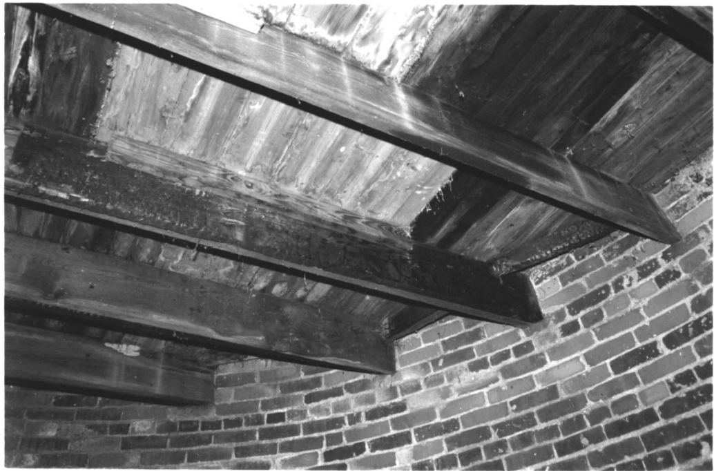
Remington Water Tower, Jasper Co, IN
