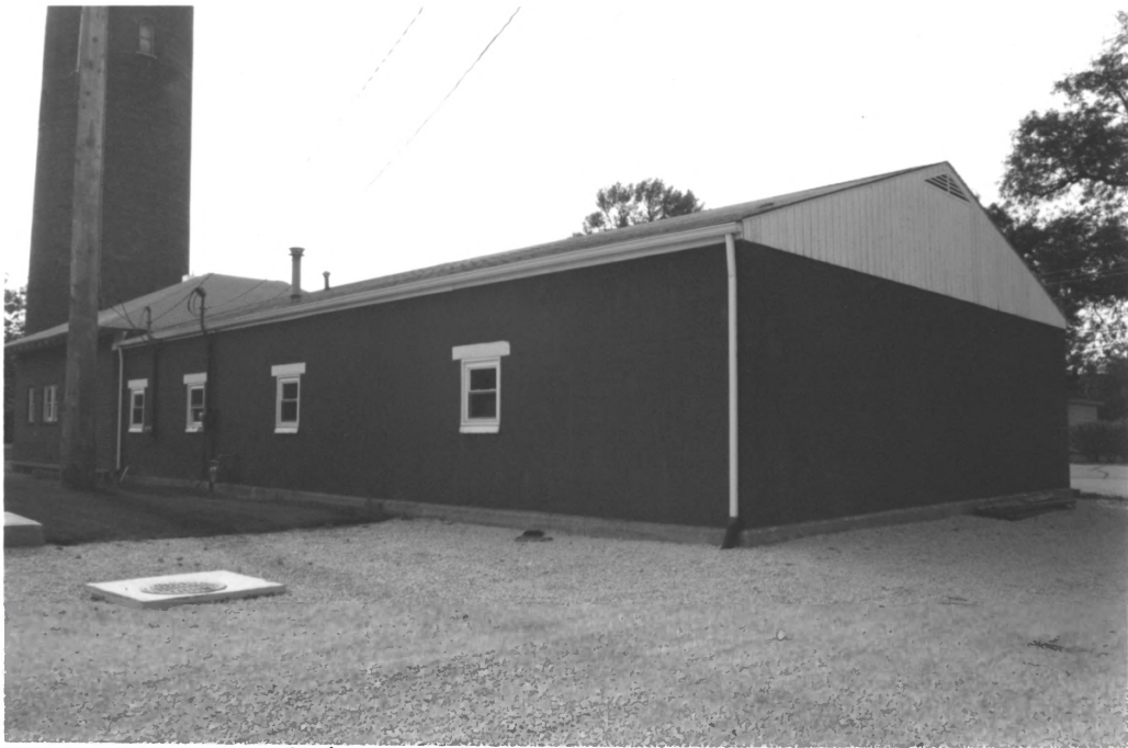
Remington Water Tower, Jasper Co, IN
