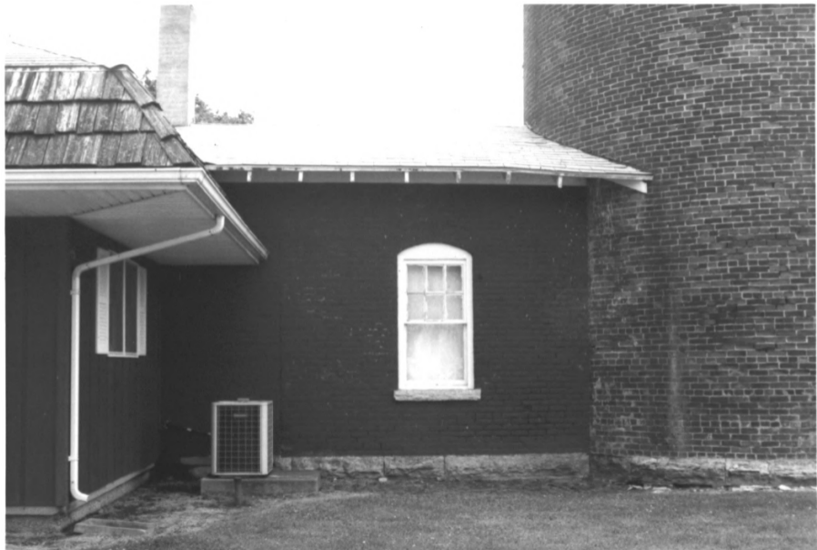
Remington Water Tower, Jasper Co, IN #9
