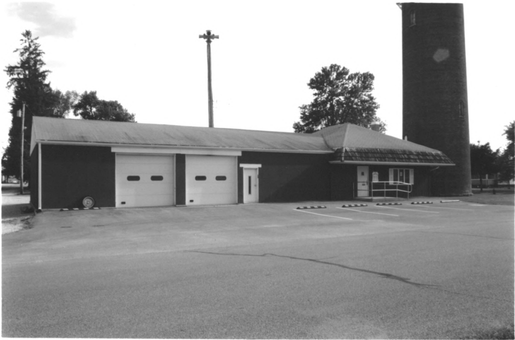
Remington Water Tower, Jasper Co, IN
