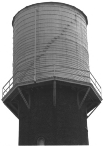
Remington Water Tower, Jasper Co, IN
