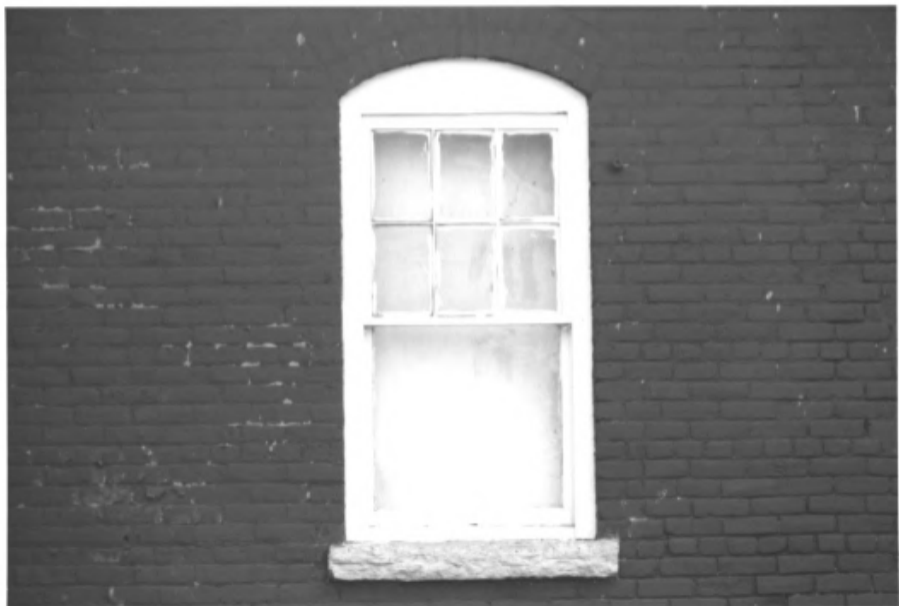
Remington Water Tower, Jasper Co, IN
