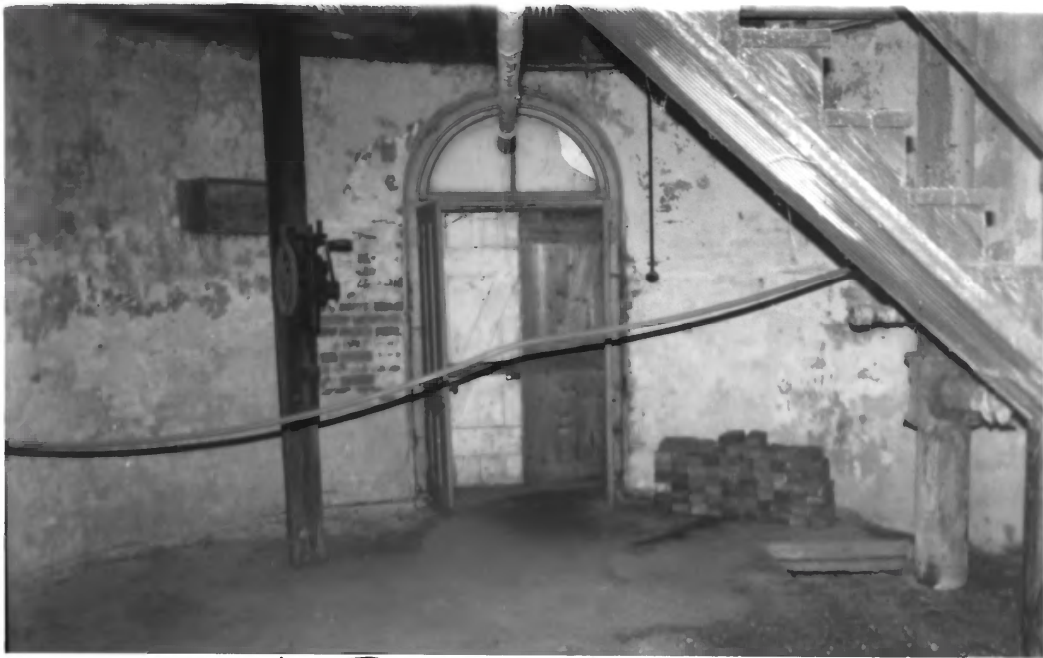
Remington Water Tower, Jasper Co, IN
