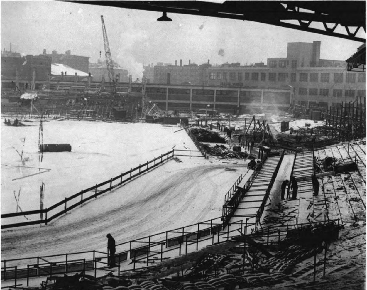
Figure 6. Rebuilding of Fenway Park, December 6, 1933. Boston Globe
