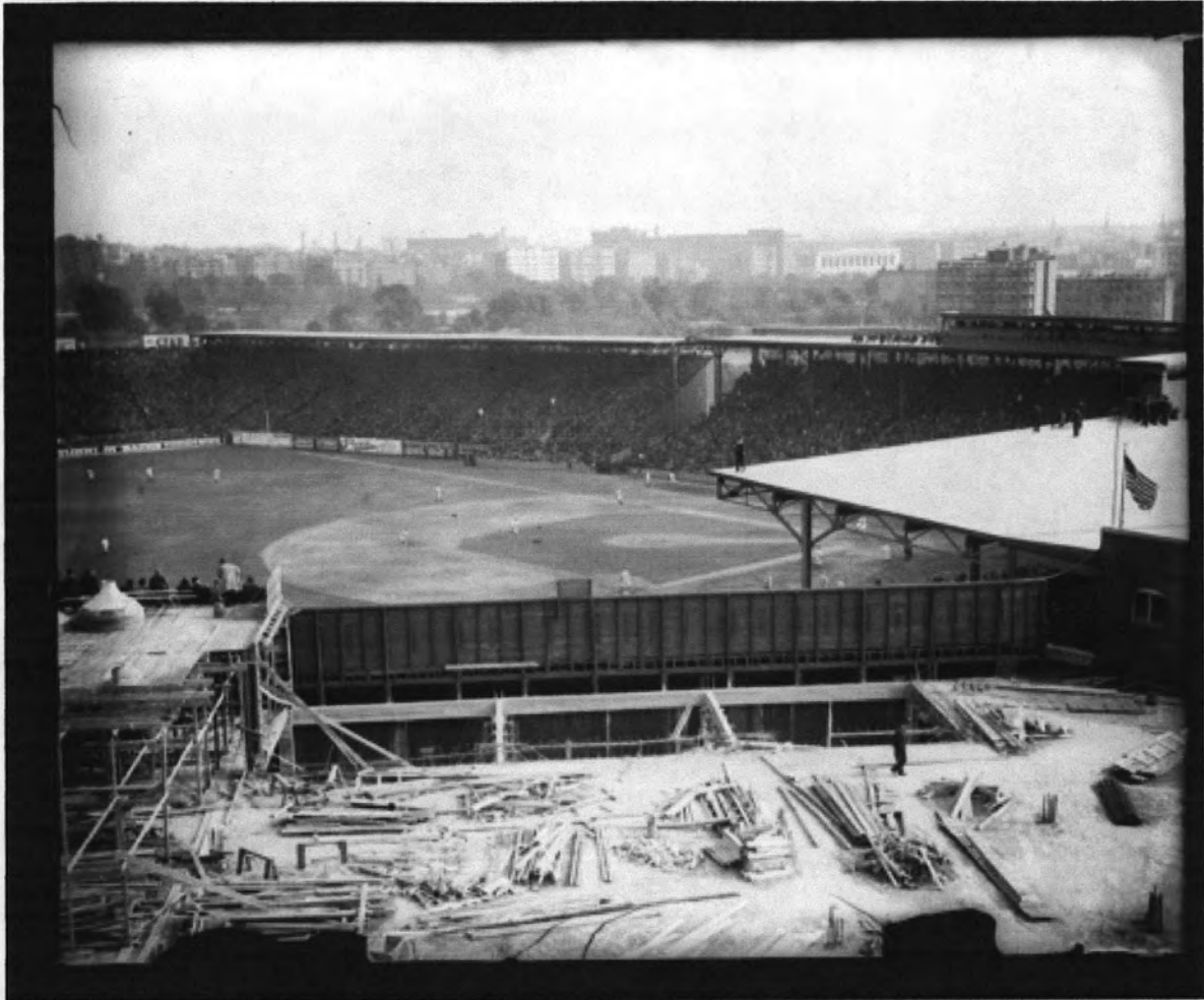
Figure 10. John B. Smith Building under construction in foreground, looking east, 1914. Braves vs. Philadelphia at Fenway, World Series, 1914.
