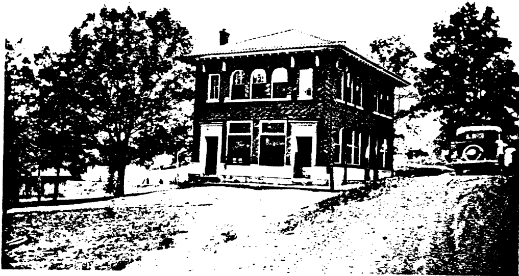
This photograph was taken shortly after the completion of the building.
