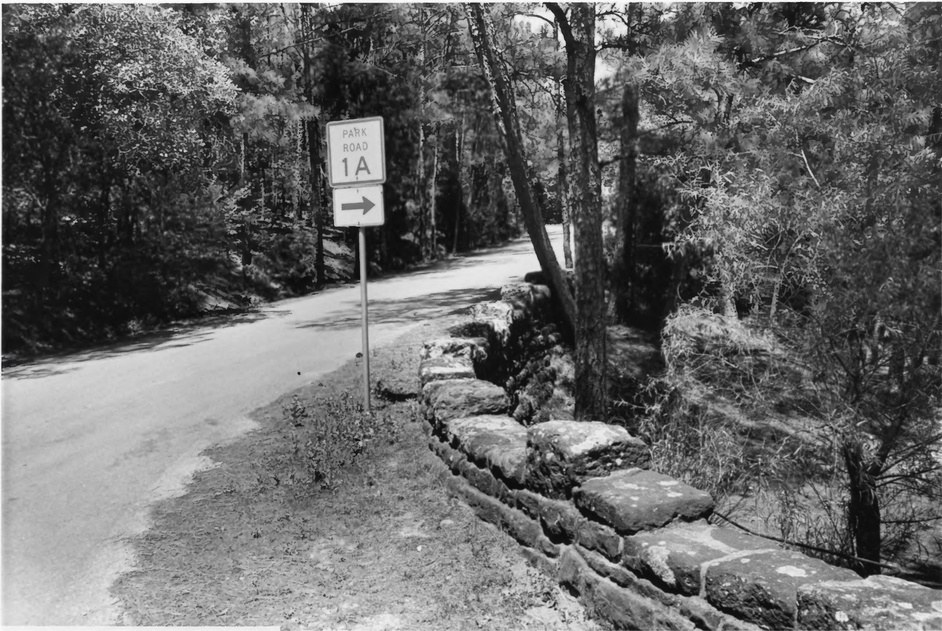
BASTROP STATE PARK Bastrop vic., Bastrop County, Texas Entrance to Cabin Area Spur Road Photo: Ethan Carr, 1995
