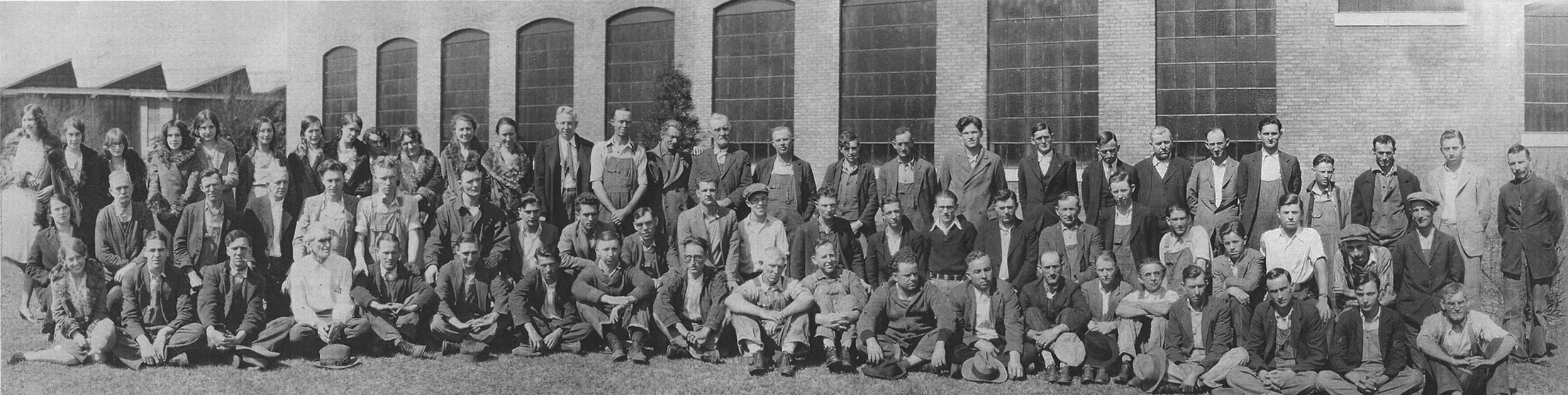
DUNEAN MILL GARDING ROOM, GREENVILLE, S. C. MAR. 1931
