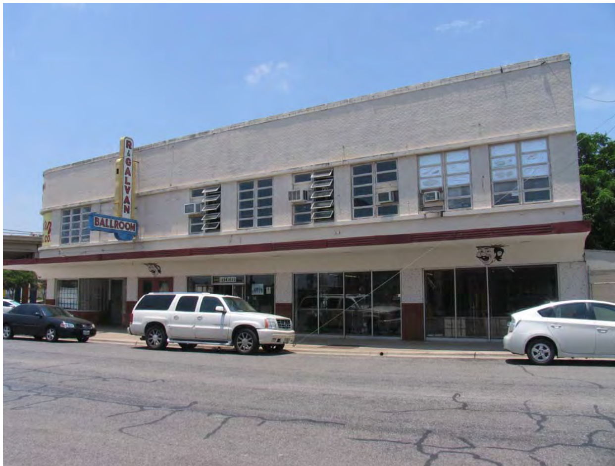
Photo 5 South elevation Camera facing north
