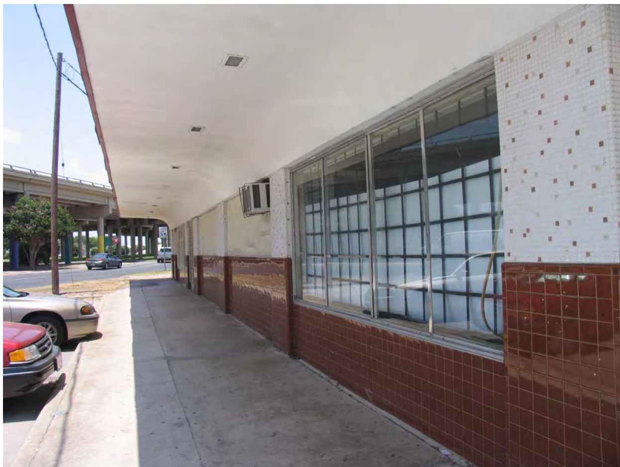
Photo 4 West side storefront windows Camera facing north
