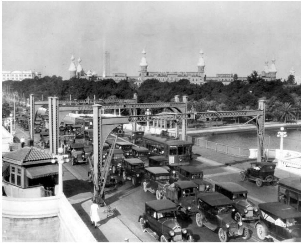
View of Third Lafayette Bridge, circa 1920.
