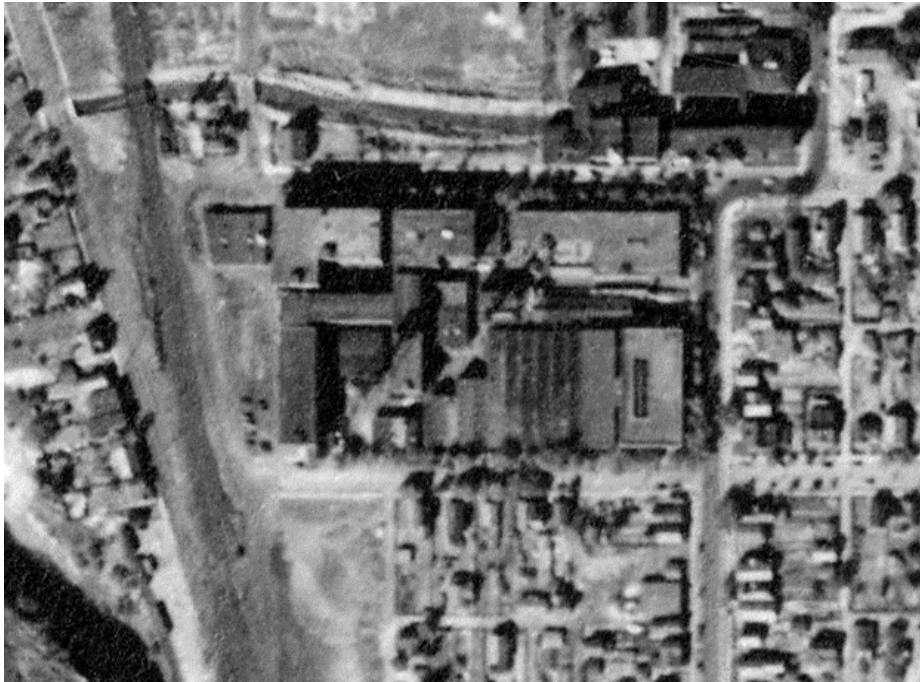
Figure 10: Aerial view, 1939. Shows all existing buildings except C-2, C-3, and M-1. (Courtesy http://www.pennpilot.psu.edu/ )
