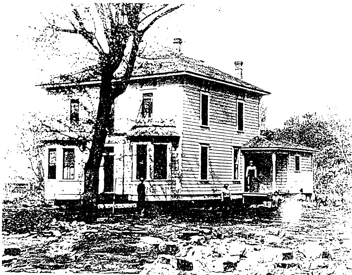
The Frazier home being moved to accommodate a street, 1913.
