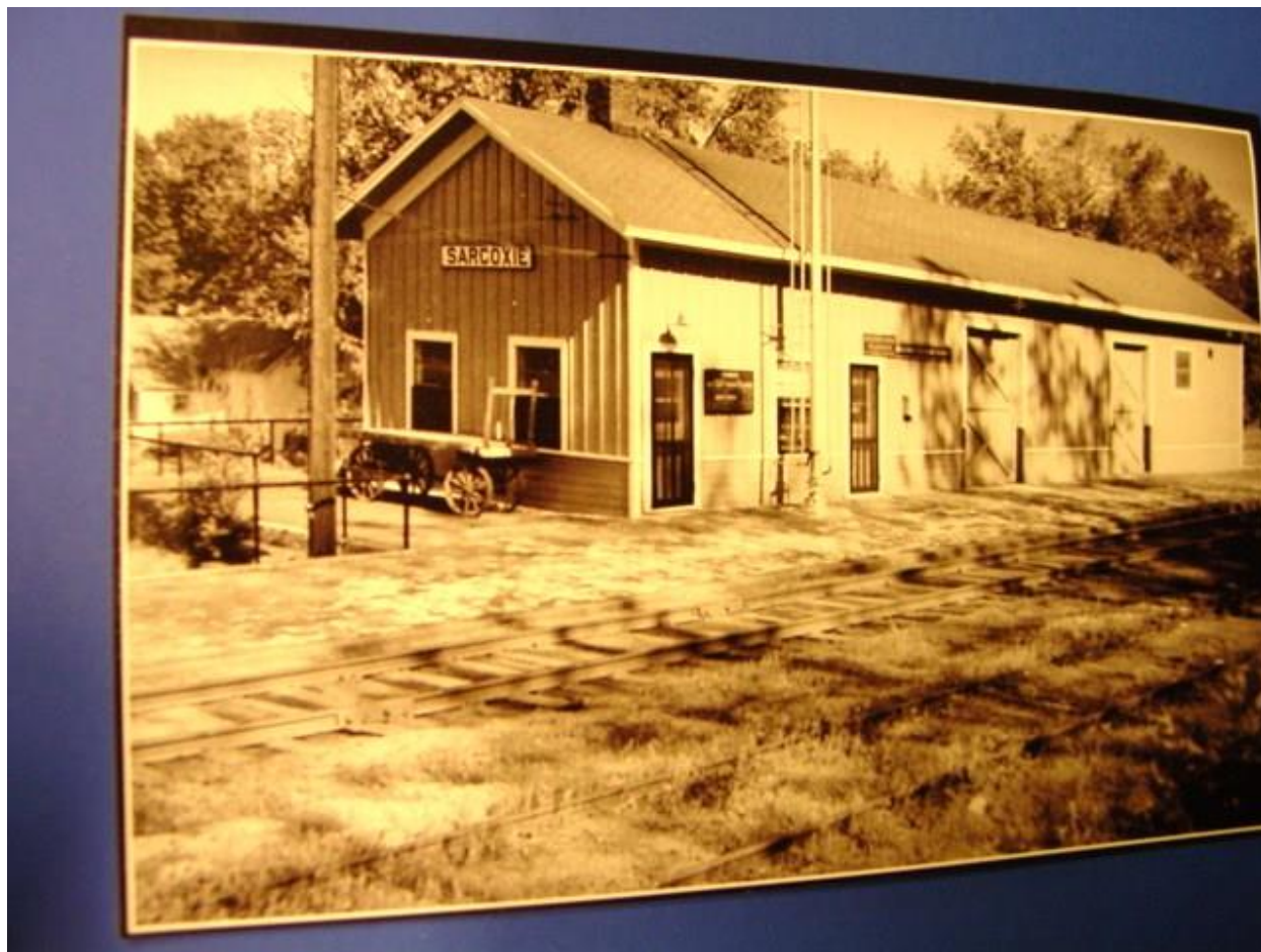
Figure 2: The Frisco Depot located west of the Sarcoxie Historic District on S. 7 th Street was torn down in c.1970. In October of 1960 the Frisco railroad abandoned its two last passenger trains between Monett and the Kansas-Missouri line. The railroad first began running its trains into Sarcoxie around c.1872. At one time the railroad operated four passenger trains through Sarcoxie each day. The depot was still serving Sarcoxie in 1968. Photo provided by Larry Myers, Sarcoxie resident. May 19, 2014.
