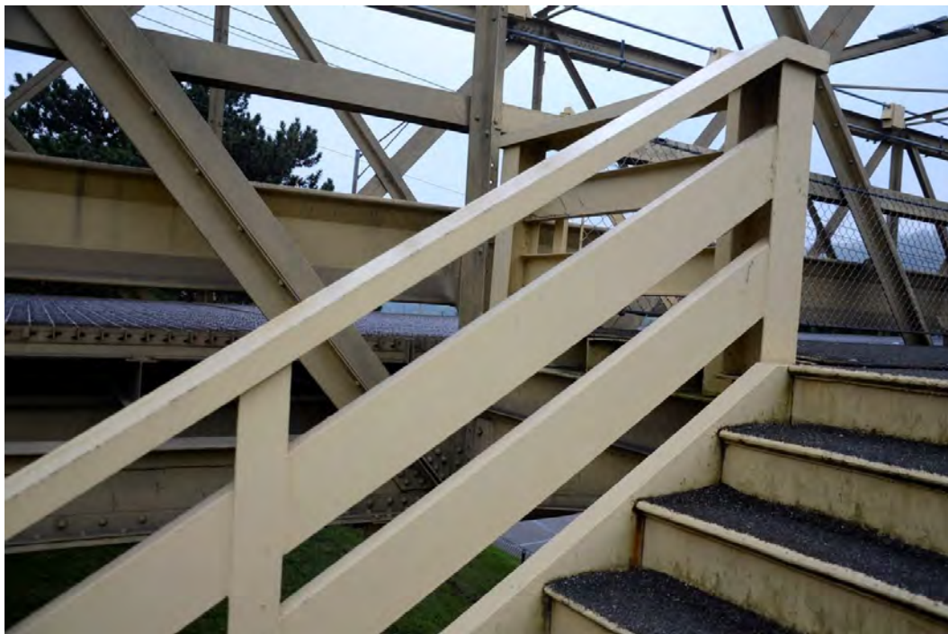
Photo 6: Market Street Bridge, Handrail leading to Pedestrian Walk, facing NE
