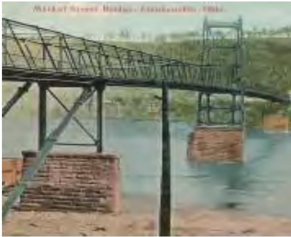
Figure 8: In October 1903, stone masons began working on the cut stone piers. (Courtesy of Jefferson County Historical Society)
