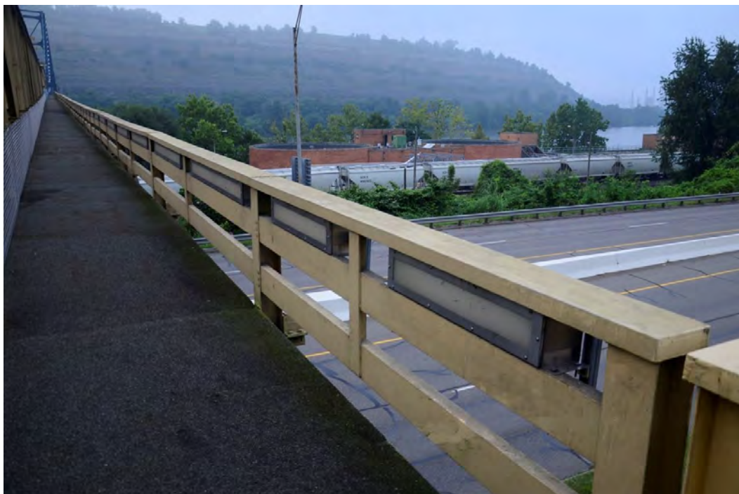
Photo 8: Market Street Bridge, Pedestrian Walk on Downstream side, Note lighting under Handrail Cap, facing East
