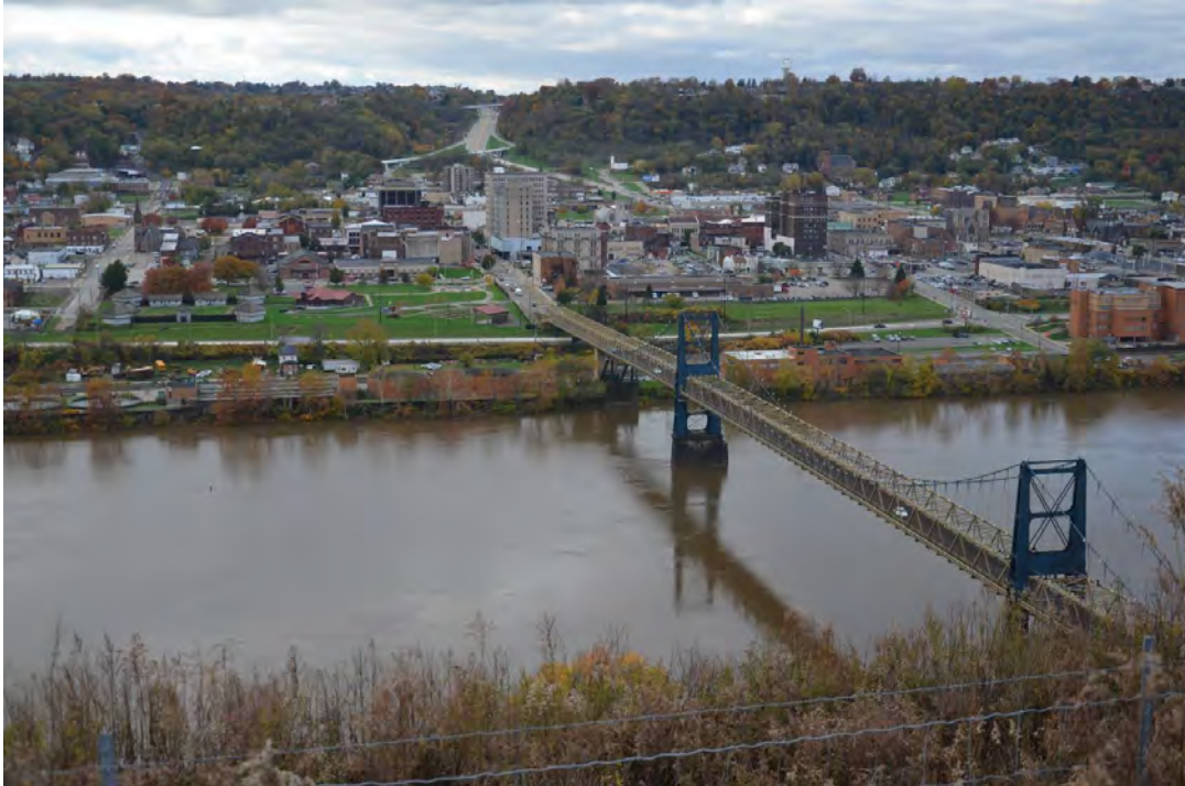
Photo 1: Market Street Bridge, Facing NW, standing on WV side of Ohio River
