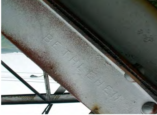
Figure 7: Original steel purchased from Bethlehem Steel Corporation for the Market Street Bridge is stamped with the foundry's name.
