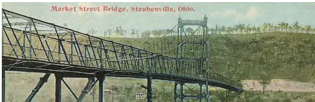
Figure 1: Early depiction of Market Street Bridge illustrating tower finials and cresting. Note the lack of steel plates on the tower. (Courtesy of the Jefferson County Historical Society).
