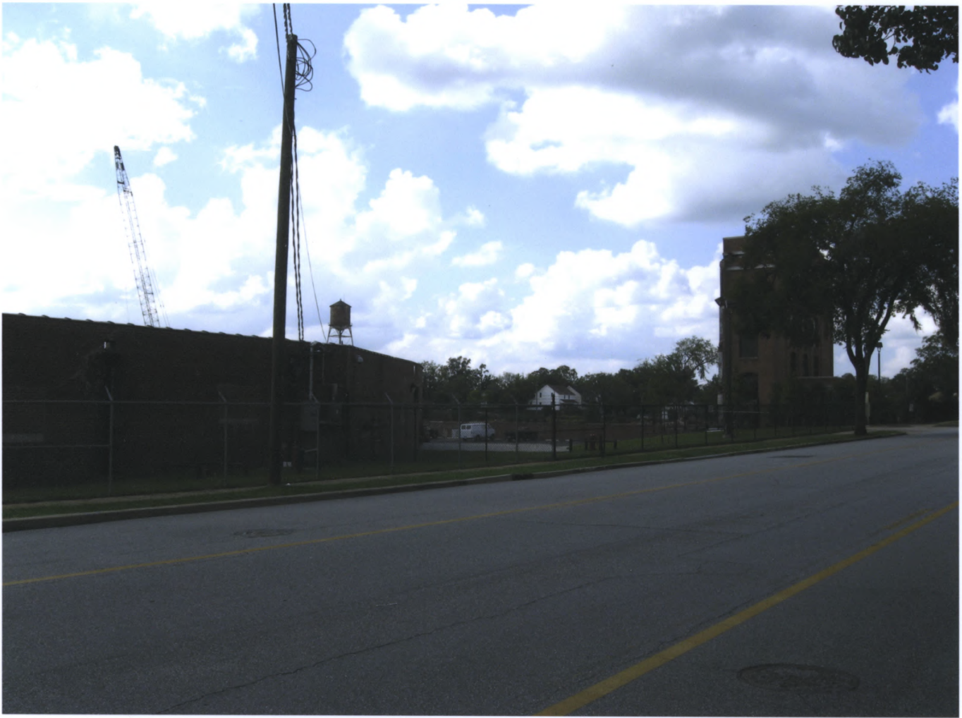
BIBB CITY HISTORIC DISTRICT, MUSCOGEE COUNTY, GEORGIA ATTACHMENT 7: WAREHOUSE AND FRONT BAY OF BIBB MILL AUGUST 19, 2009 PHOTO BY LYNN SPENO, HPD
