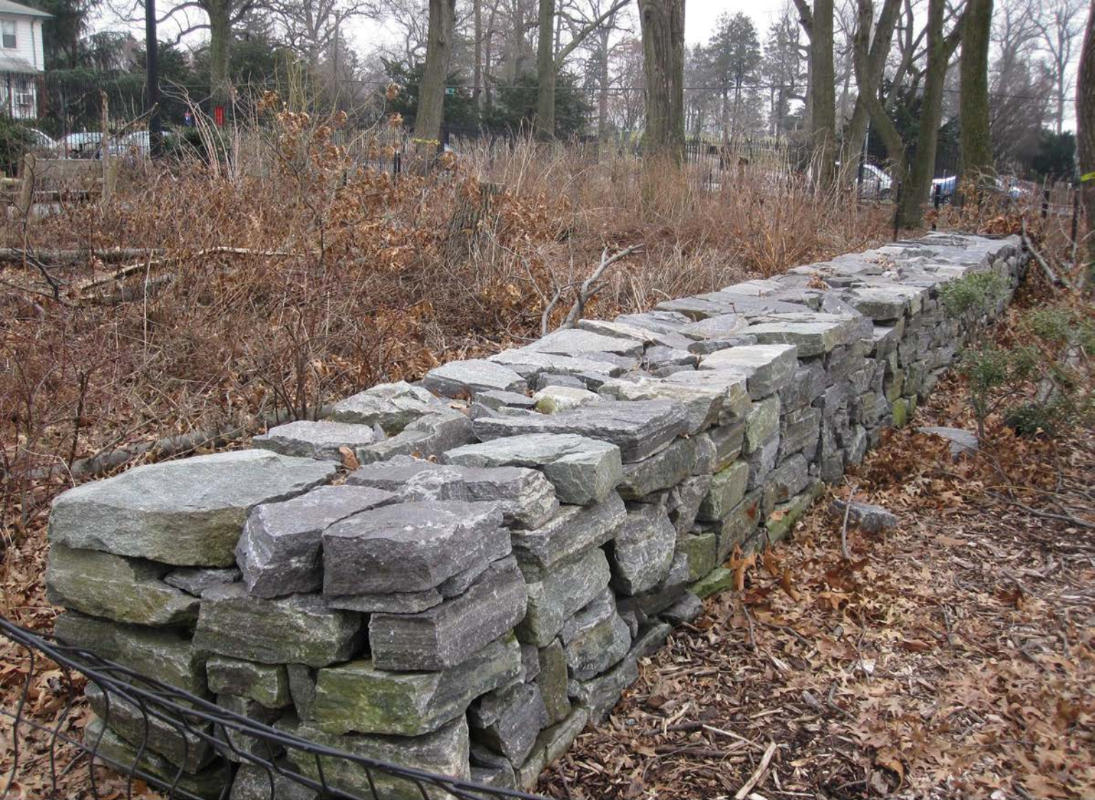
Olde Towne of Flushing Burial Ground, Queens, NY. Photo 10 of 17
