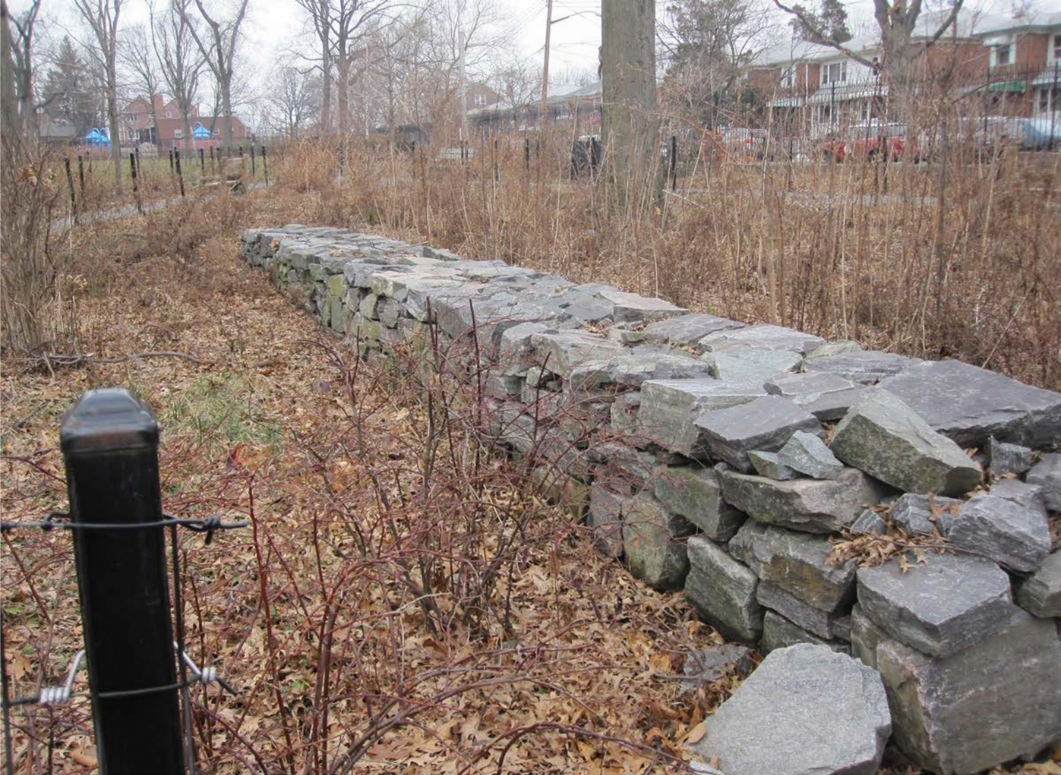
Olde Towne of Flushing Burial Ground, Queens, NY. Photo 9 of 17
