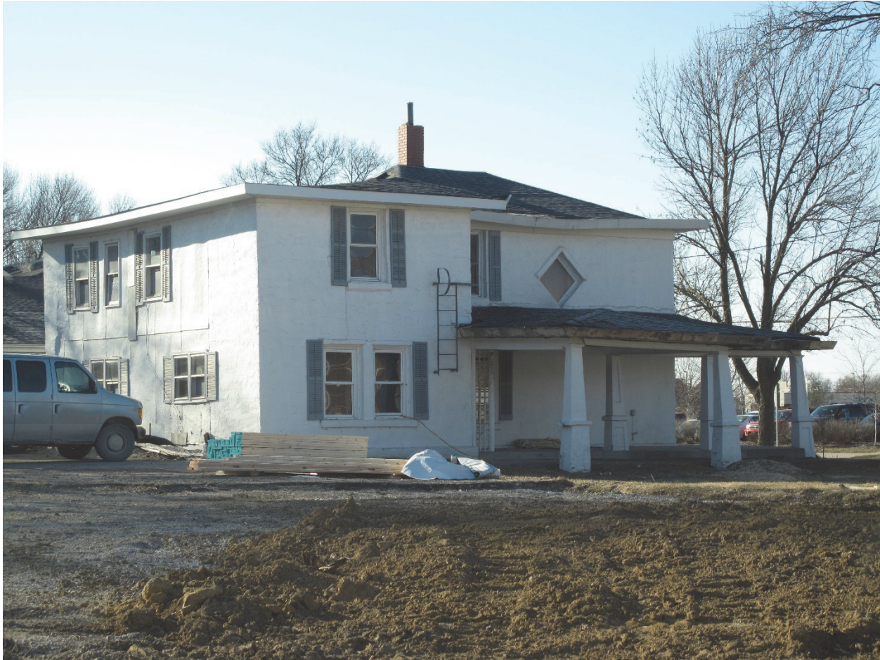
Figure 6. View of the Tate Arms in December 2014, facing southwest. This photograph shows the house before its most recent renovation. The second story had been stuccoed by this time. Older features that have been replaced since 2014 include the roof, which is similar but not identical to the hipped roof shown here, and the fenestration on the rear wall, shown at the left side of this photograph. Photograph by Marlin Ingalls, Office of the State Archaeologist, Iowa City, December 31, 2014. Included in electronic files associated with Carlson and Ingalls, Phase I Intensive Historic Architectural Survey of the Sabin School and Southside Iowa City Neighborhood, Johnson County, Iowa; on file, Office of the State Archaeologist, University of Iowa, Iowa City.
