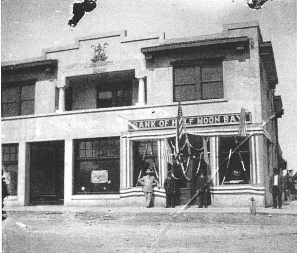
Figure 8: Joseph Debenedetti Block, constructed with leftover materials from bridge construction after the 1906 earthquake and fire
