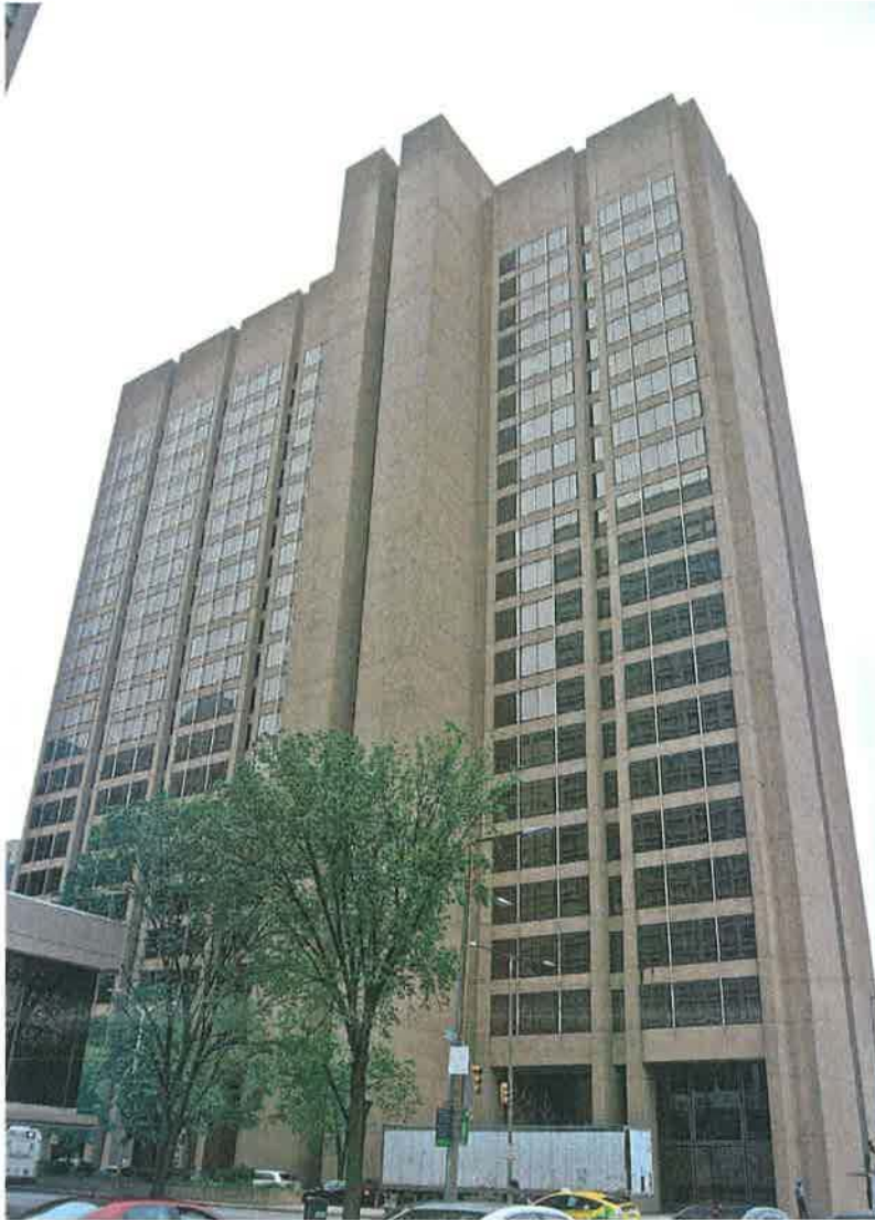
MD_BaltimoreCity_MercantileDeposit&Trust_0001.tif North Facade
