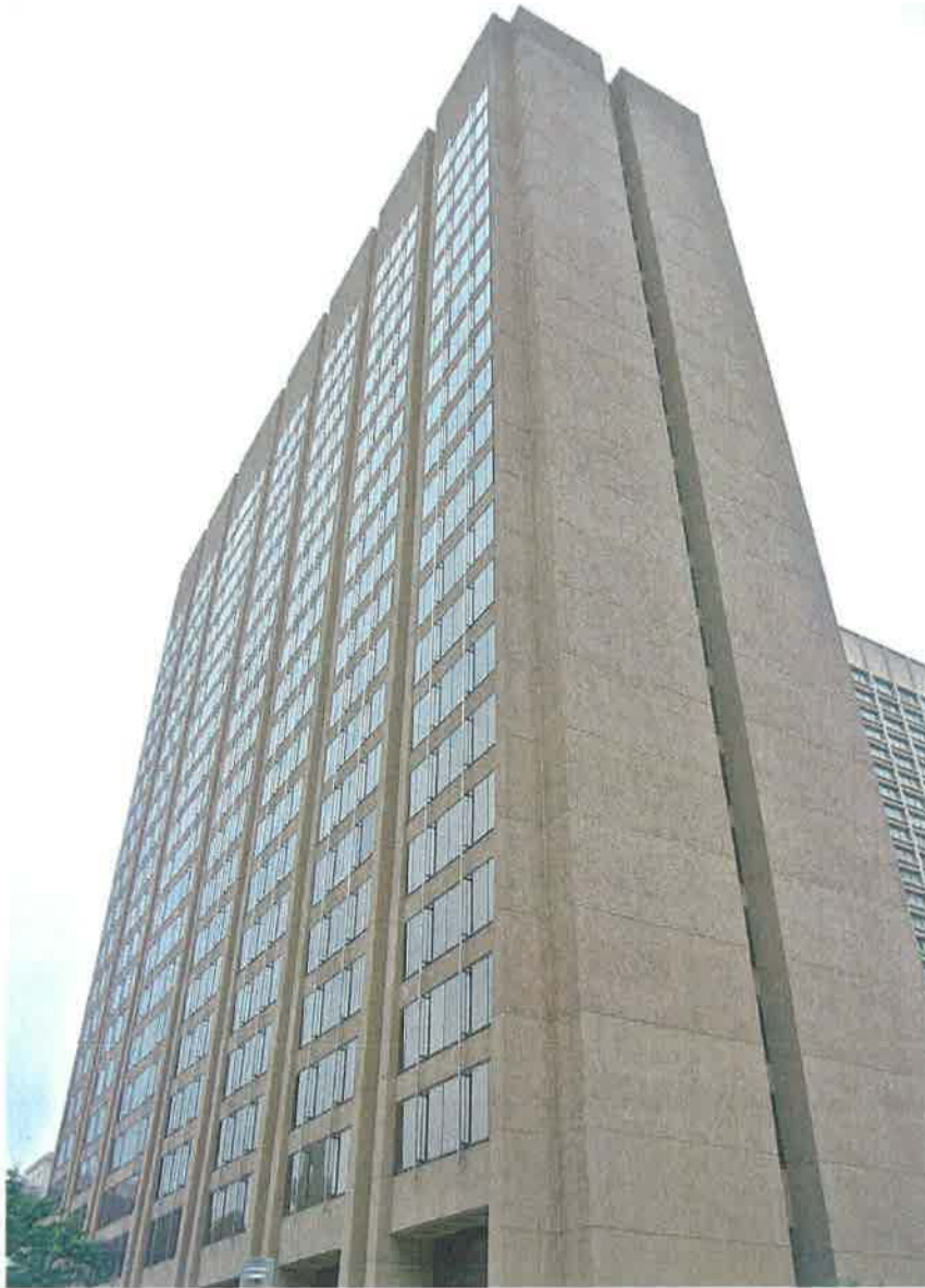
MD_BaltimoreCity_MercantileDeposit&Trust_0005.tif View from southeast
