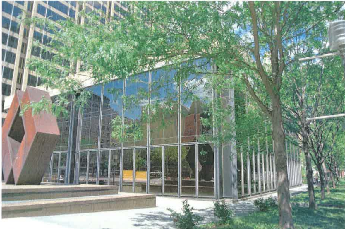
MD_BaltimoreCity_MercantileDeposit&Trust_0014.tif Pavilion from southwest
