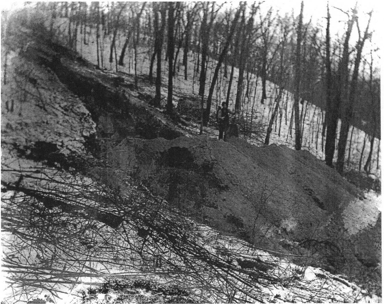
Mindoro Cut construction, Spring 1908, collection of John and Joan Dolbier, La Crosse County, WI
