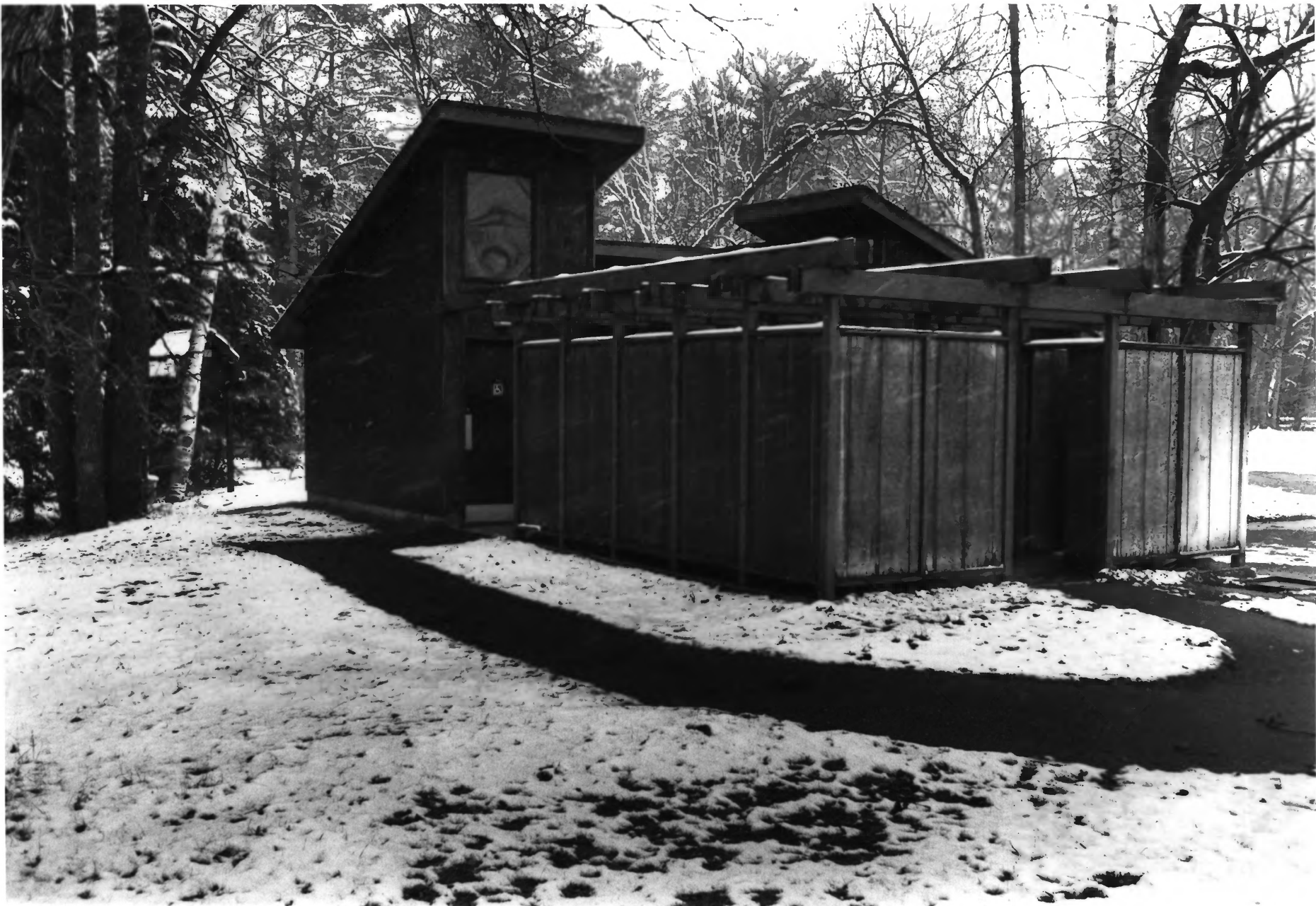
LAKE BEWIDJI STATE PARK BELTRAMI CO., MN BLDG #3 PHOTO I.D. 09119# 11 (NON-CONTRIBUTING)
