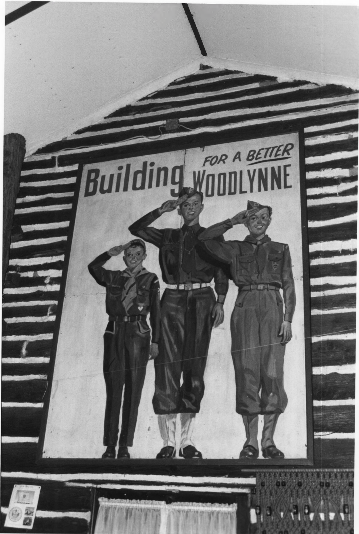
WOODLYNNE LOG CABIN CAMDEN COUNTY, NEW JERSEY PHOTOGRAPH #6 of 6
