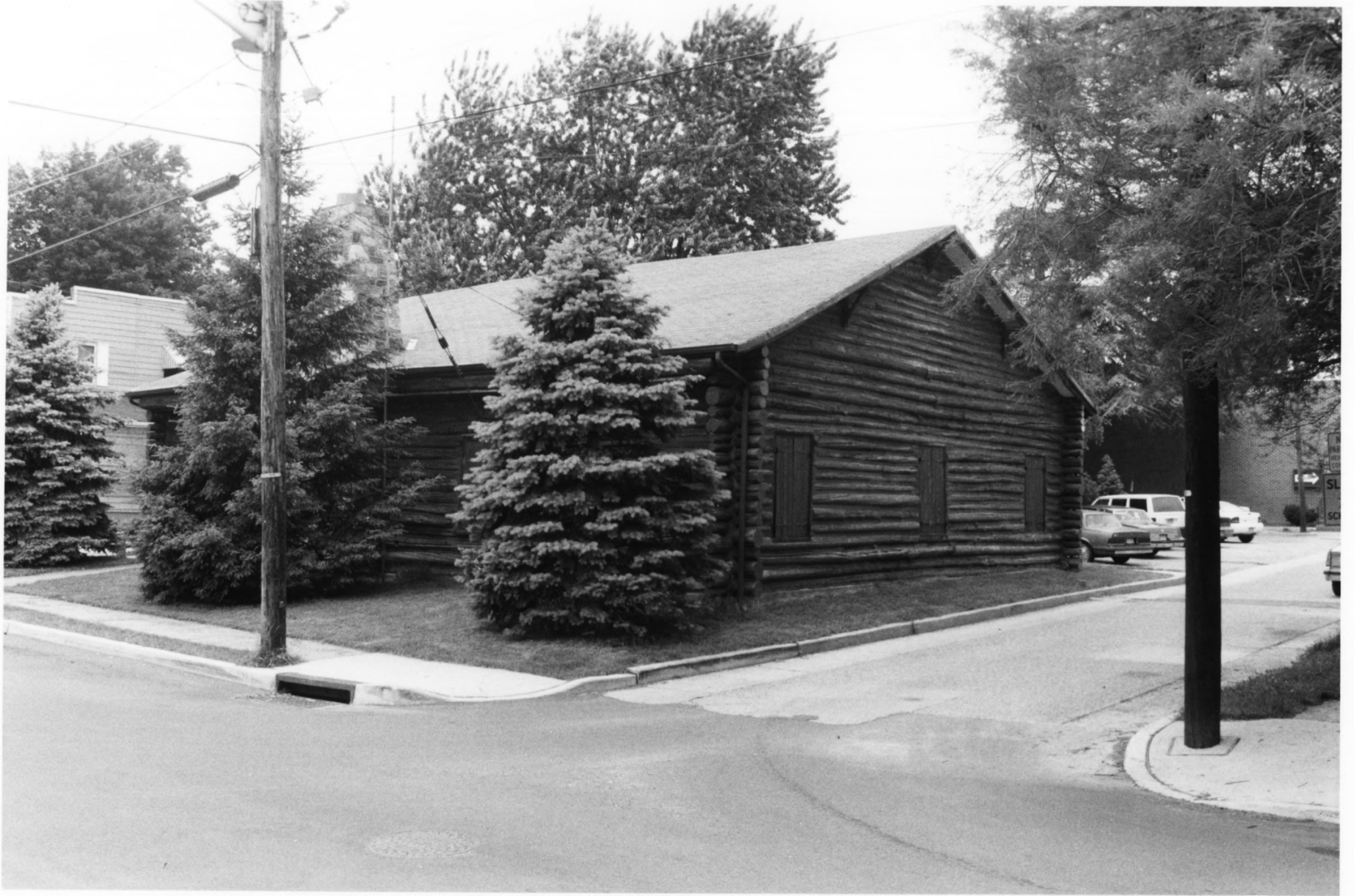
WOODLYNNE LOG CABIN CAMDEN COUNTY, NEW JERSEY PHOTOGRAPH #2 of 6
