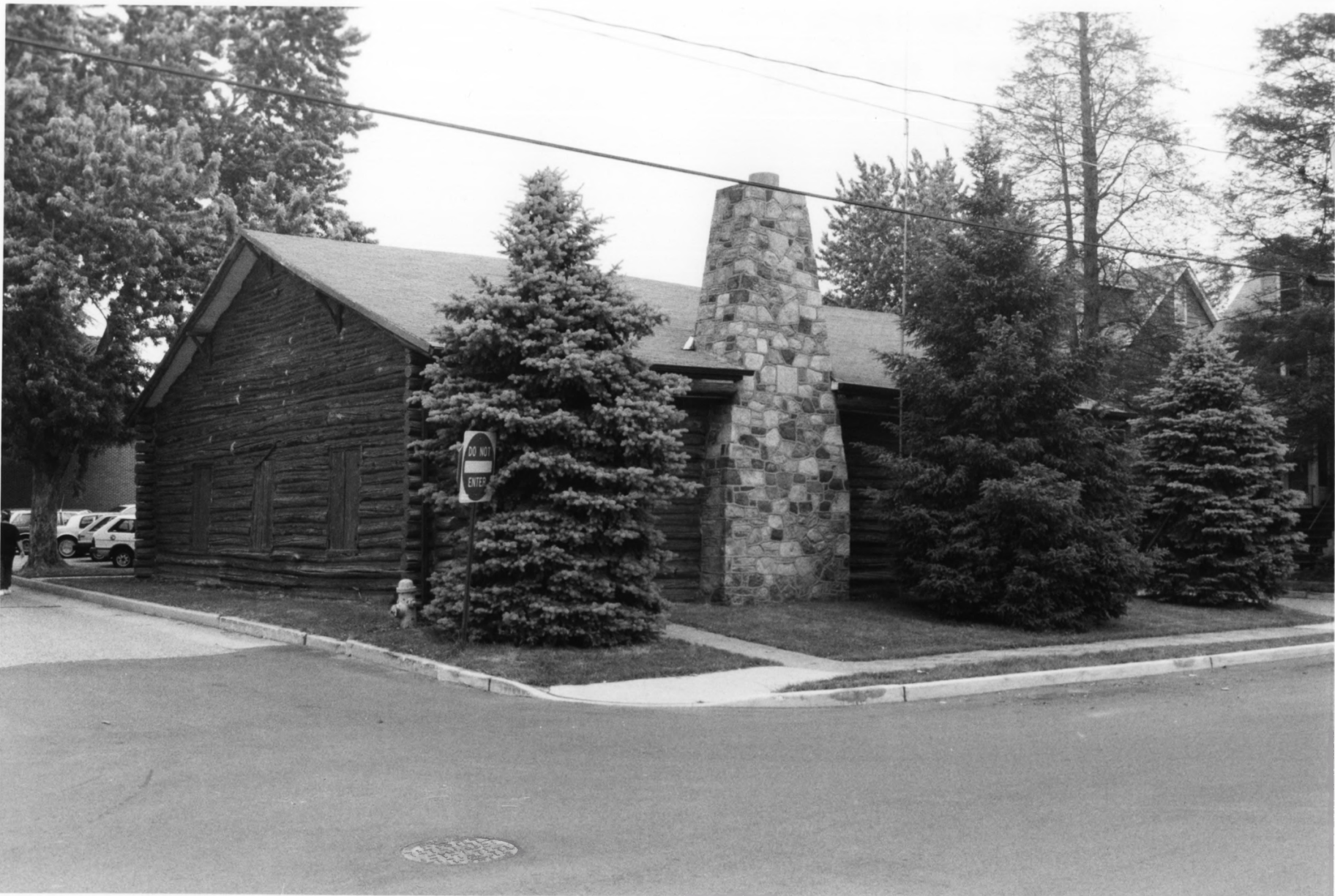
WOODLYNNE LOG CABIN CAMDEN COUNTY, NEW JERSEY PHOTOGRAPH #3 of 6
