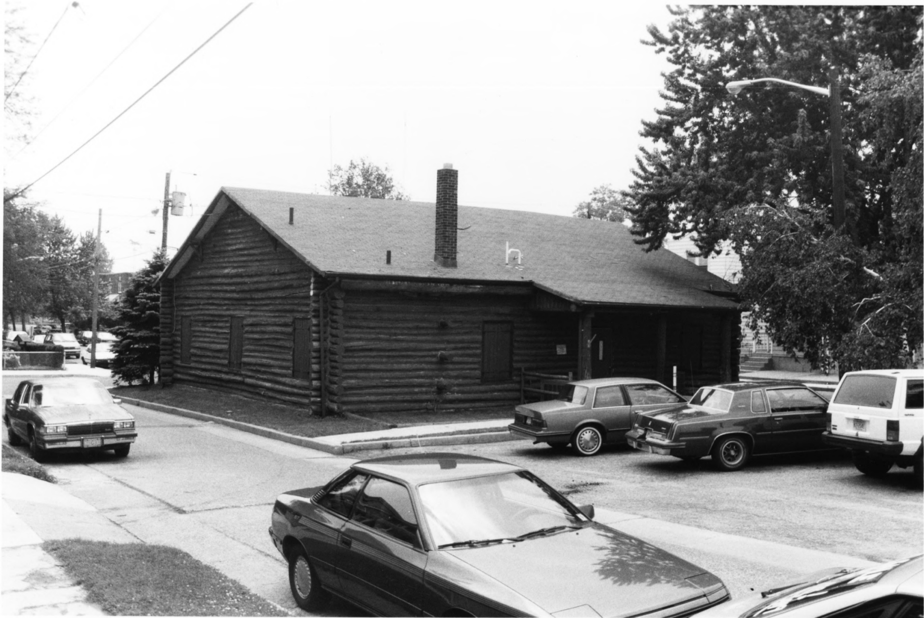
WOODLYNNE LOG CABIN CAMDEN COUNTY, NEW JERSEY PHOTOGRAPH # 1 of 6
