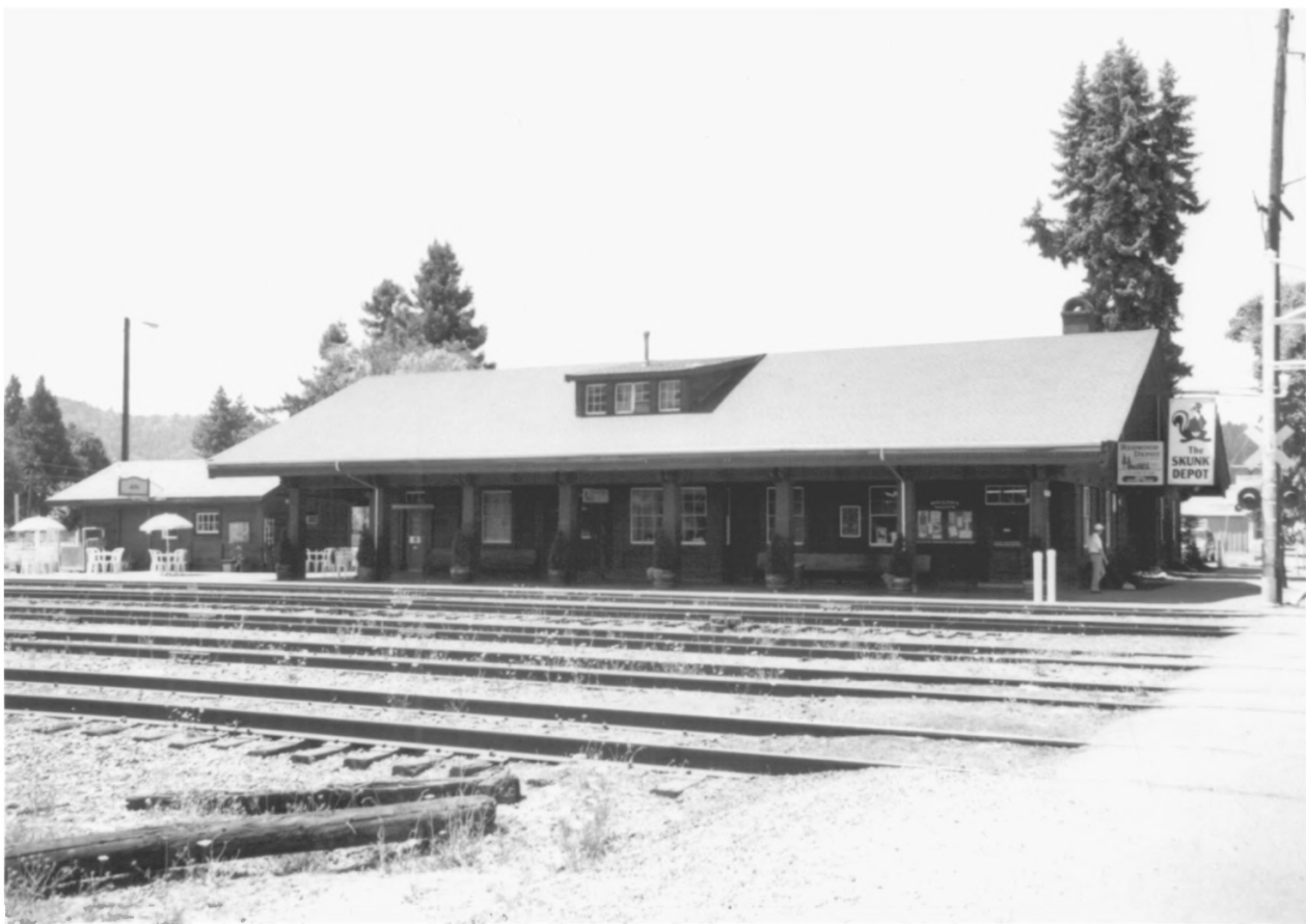
WILLITS DEPOT, MENDOCINO CO. CA PHOTO 1
