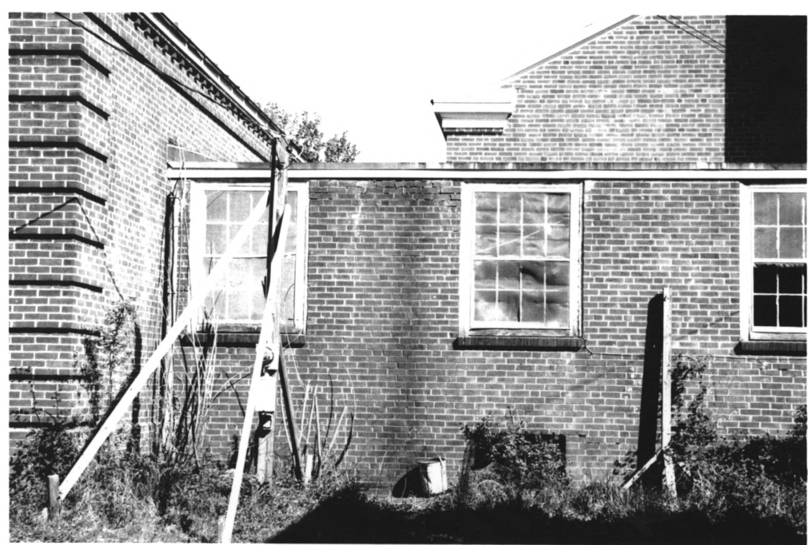
RIVERSIDE SCHOOL KNOX COUNTY TN
