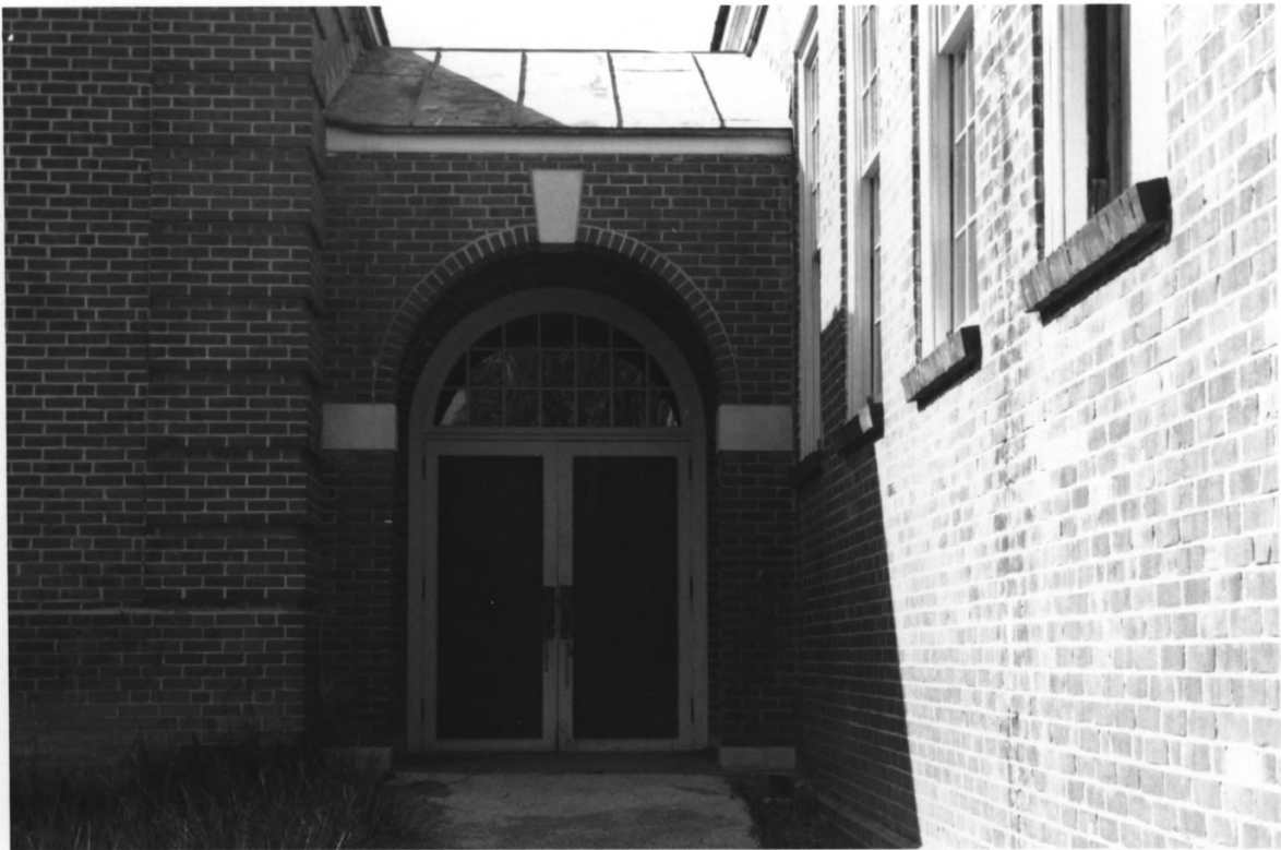
RIVERSIDE SCHOOL KNOX COUNTY TN
