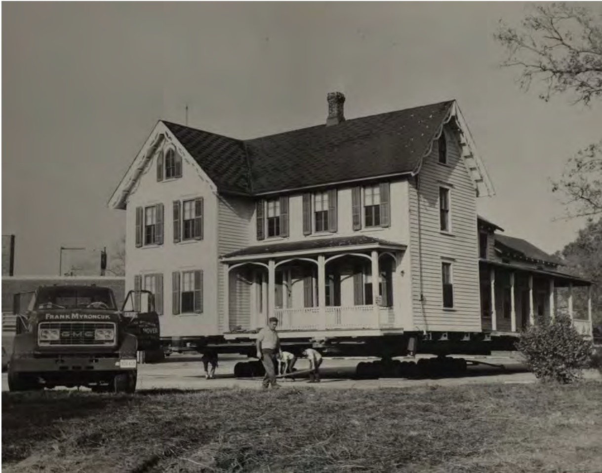
Historic Photograph 2: The Elizabeth Sculthorp Force House in transit during its move in 1971. The primary/east and north elevations are shown. Courtesy of Ocean County Historical Society.
