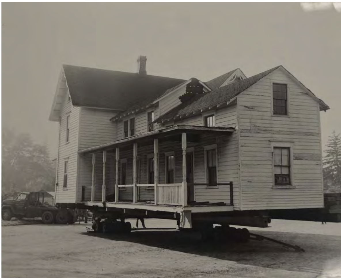
Historic Photograph 3: The Elizabeth Sculthorp Force House in transit during its move in 1971. The current north and west elevations are shown, illustrating the three volumes that make up the historic main house. Courtesy of Ocean County Historical Society.
