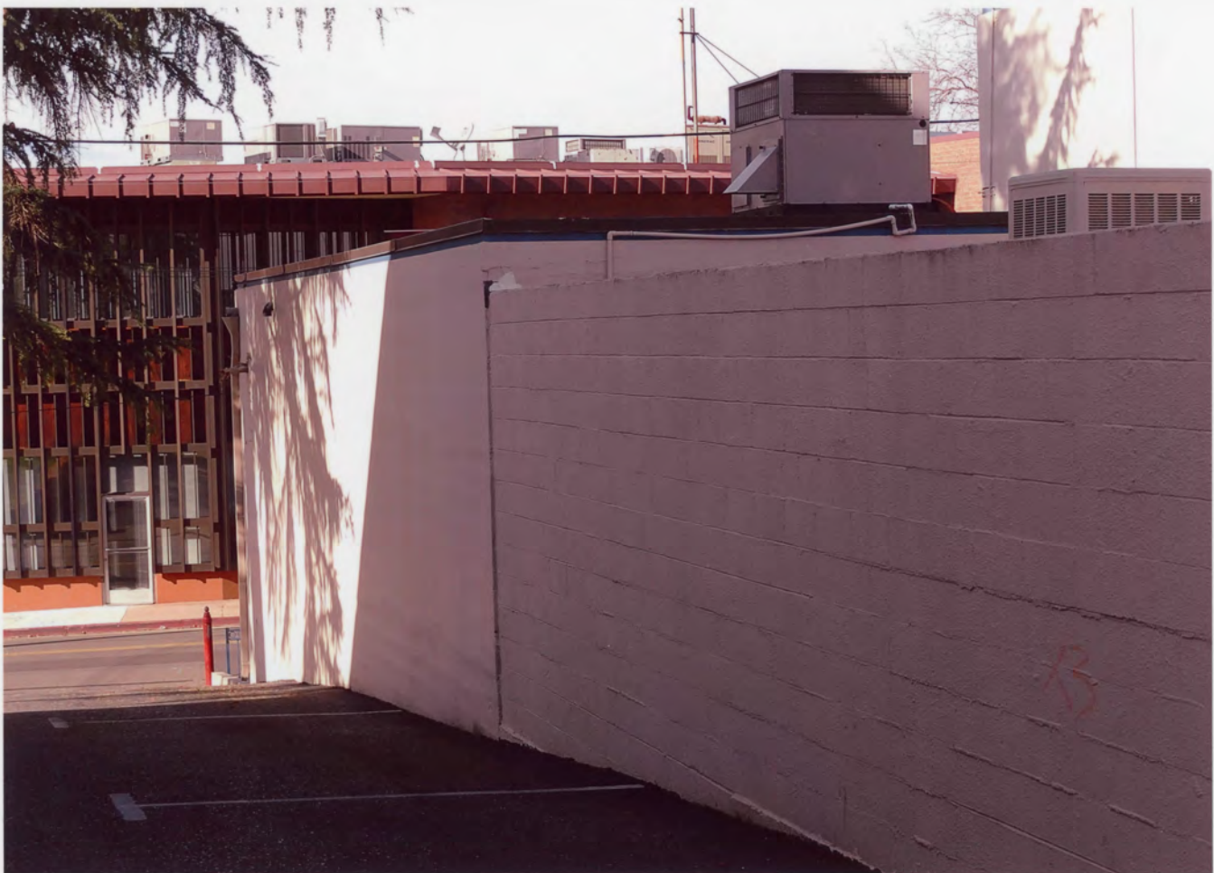
5. AUBURN CITY HALL AND FIREHOUSE PLACER COUNTY, CA
