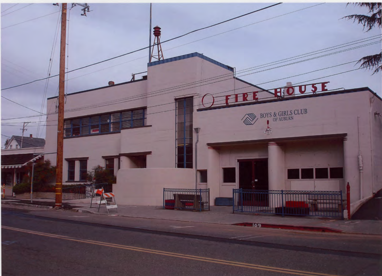
2. AUBURN CITY HALL AND FIREHOUSE PLACER COUNTY, CA
