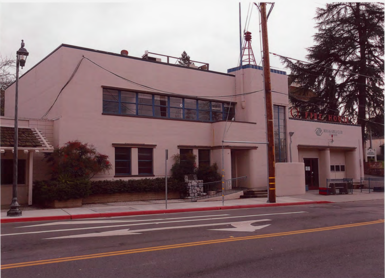
1. AUBURN CITY HALL AND FIREHOUSE PLACER COUNTY, CA
