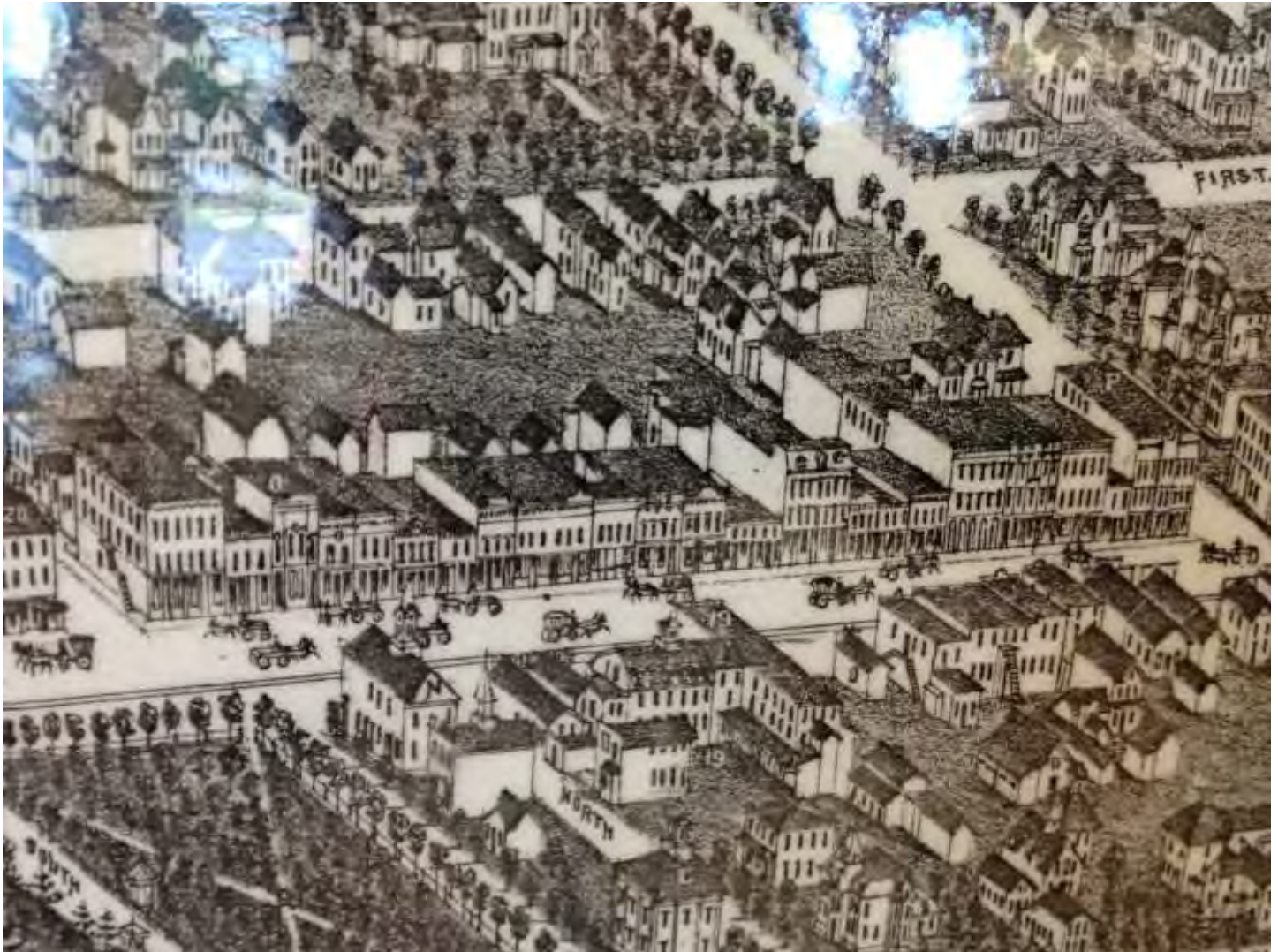
Figure 5. Birdseye View, looking at the west side of North Union Street (1882) Entire block rebuilt by this time.
