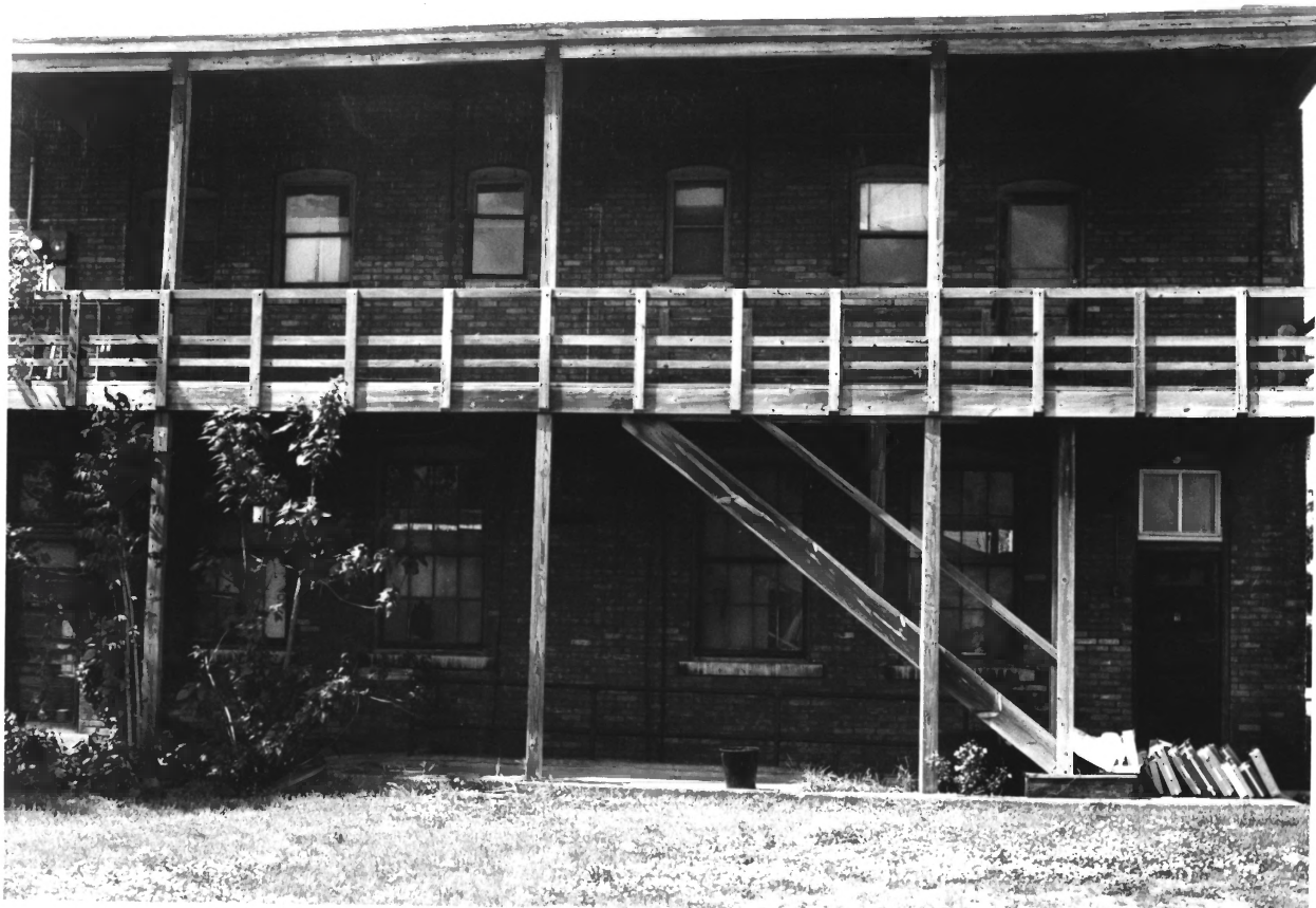
③ C. MCCORMICK BLDG, E. BANK M.P.L, SO. BEND, IN
