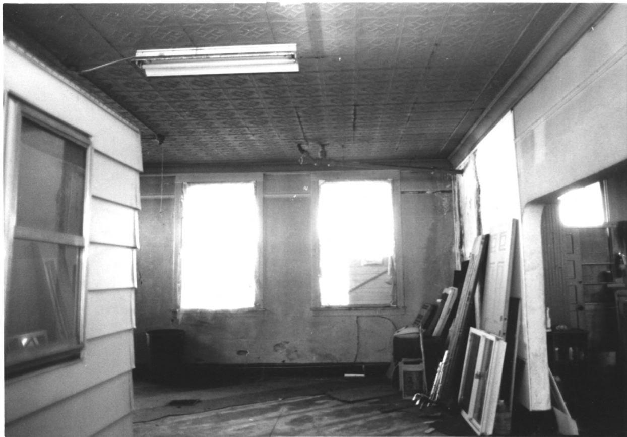
5 C. MCCORMICK BLDG, E. BANK H.P.L., SO. BEND, IN
