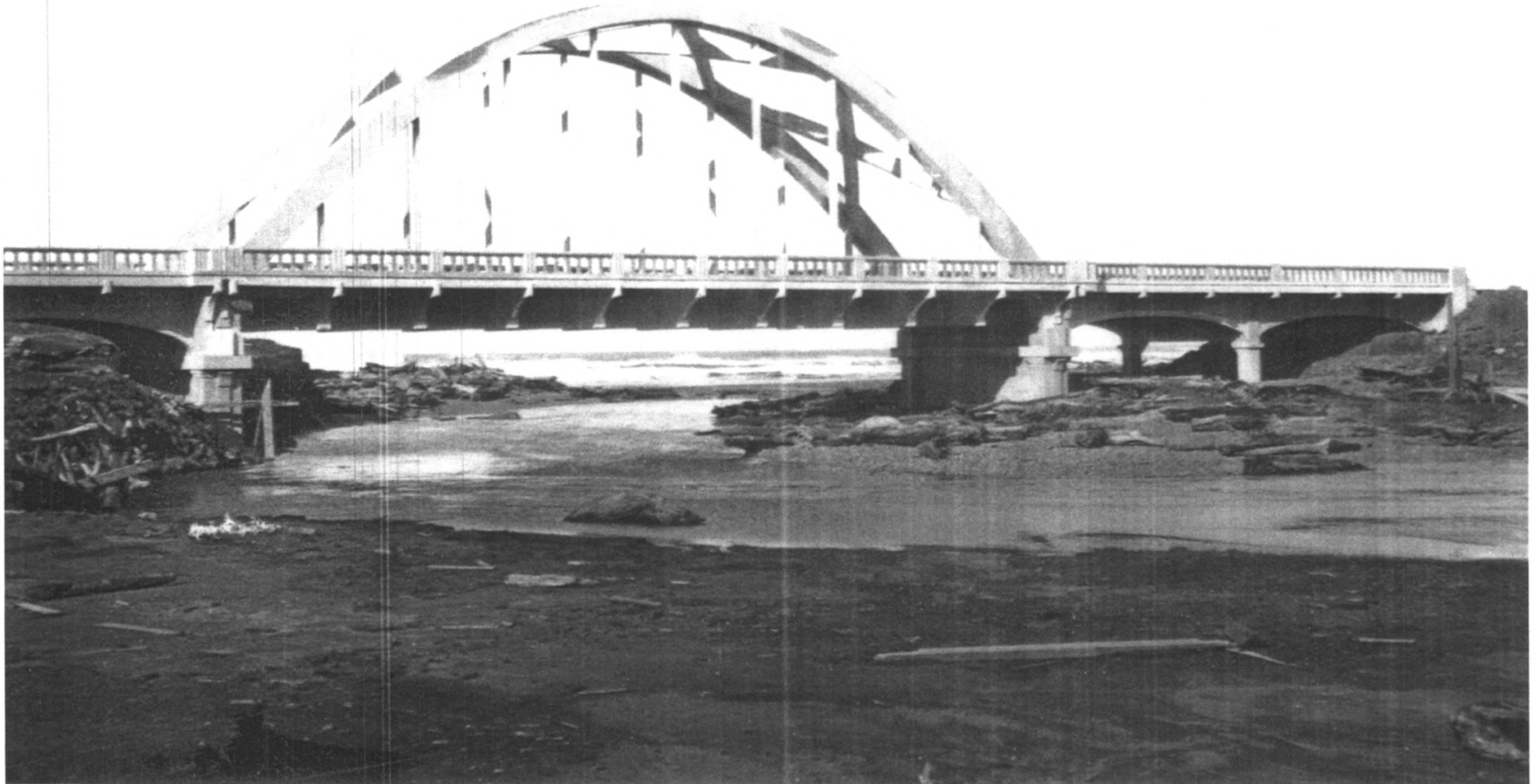
Big Creek #01180 US-101 MP 175.02 Lane County Near Yachats
