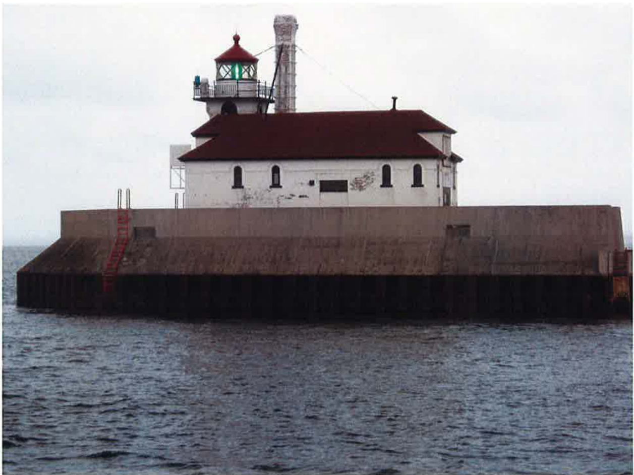
Photo 1. Lighthouse northern elevation, camera facing south.
