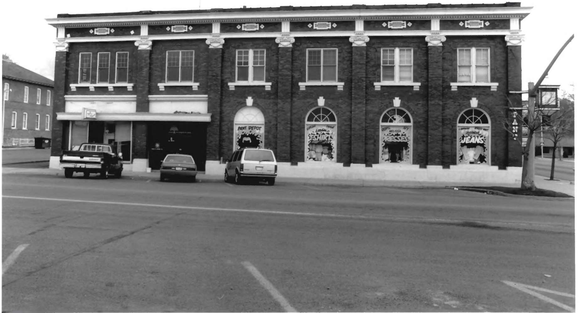
BANK OF AMERICAN Fork AMERICAN Fork, UTAH CO., UT PHOTO #2
