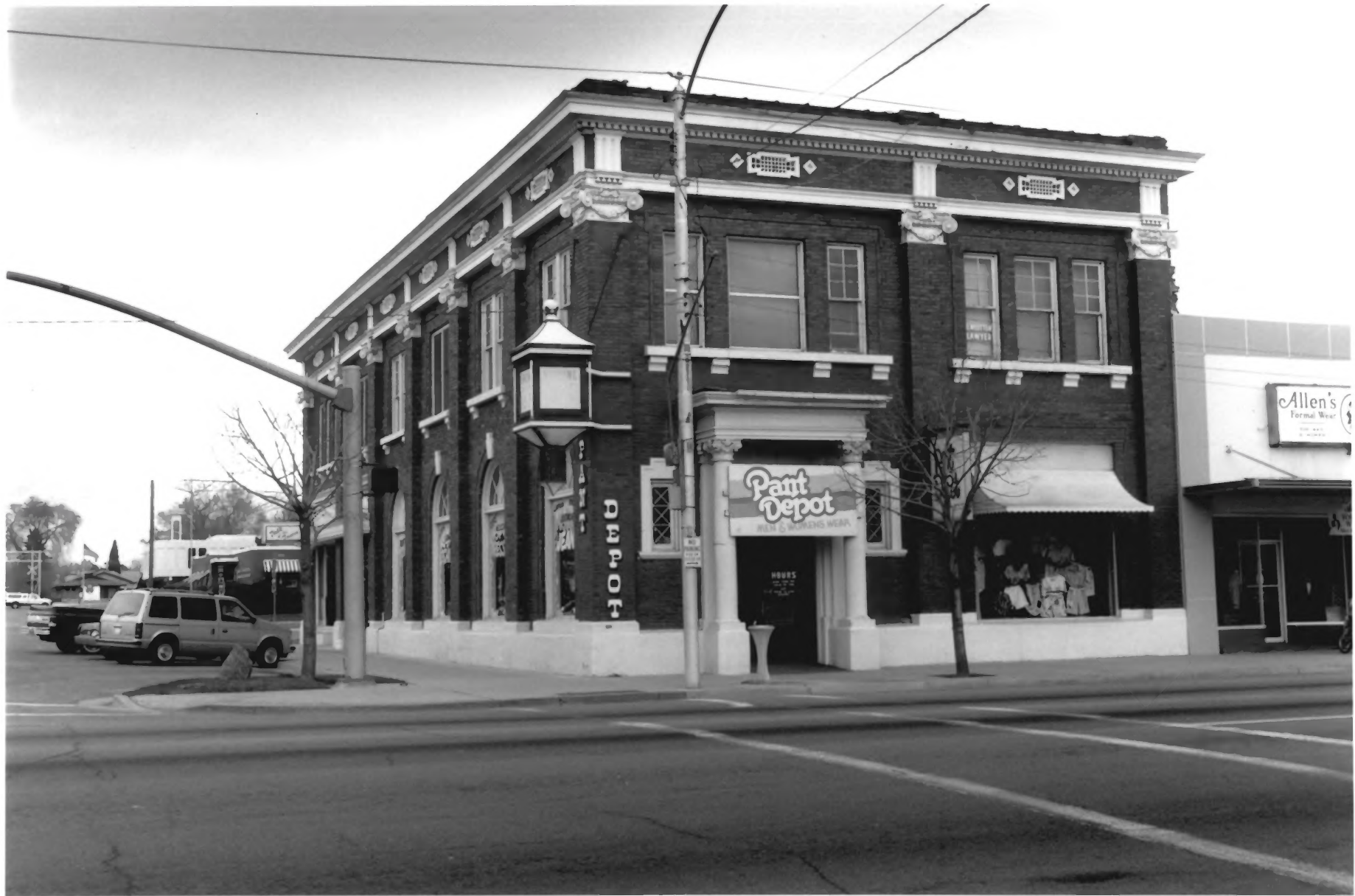
BANK OF AMERICAN FORK AMERICAN FORK, UTAH CO., UT PHOTO #1
