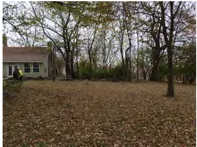
Photo 4 - Craig-Peak House - Ruins of Detached Structure
