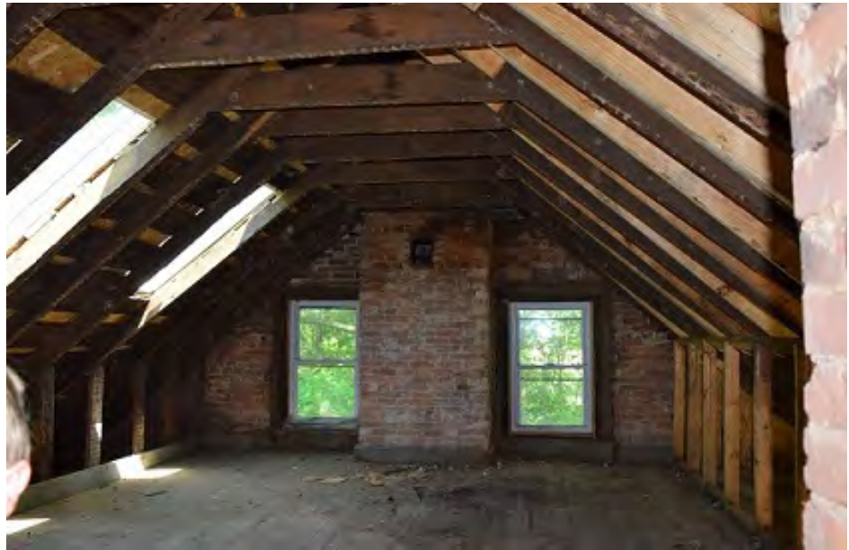
Rear Addition, Second Floor
