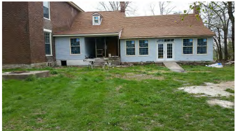
Rear Addition, South façade
