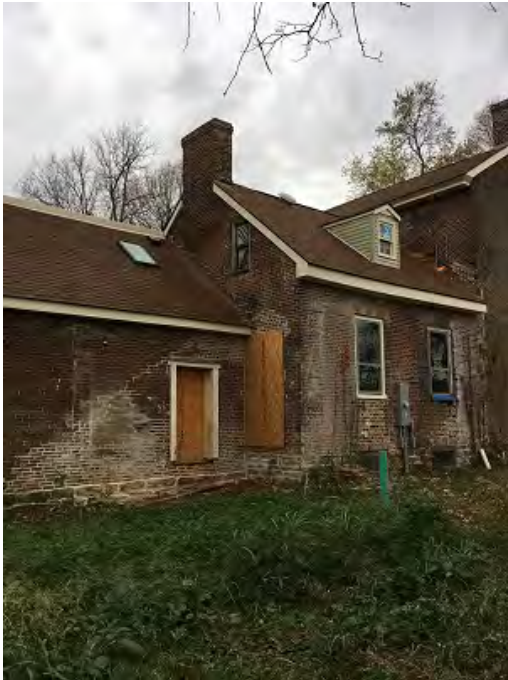
Rear Addition and Original Dwelling, North Façade
