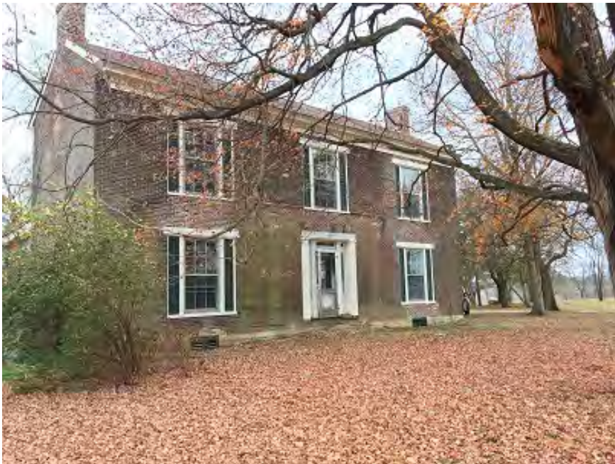
Greek Revival Addition, West façade
