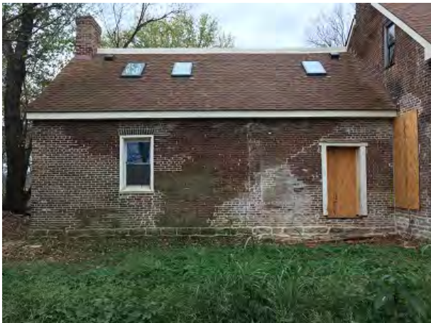
Rear Addition, North façade
