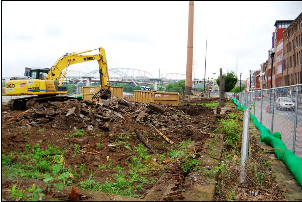
Figure 25: June 20, 2015 photograph showing clean-up after demolition of Fort Nashborough.
