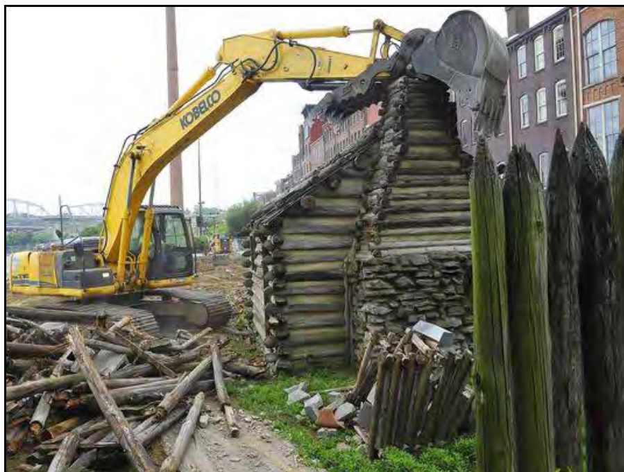
Figure 21: June 20, 2015 photograph of Fort Nashborough with demolition underway.
