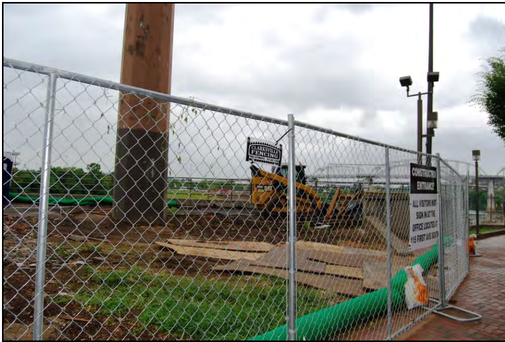
Figure 29: June 20, 2015 photograph showing clean-up after demolition of Fort Nashborough.
