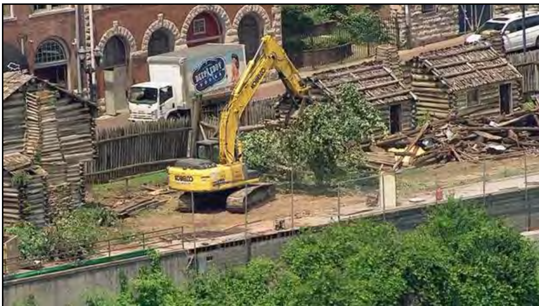
Figure 23: June 20, 2015 photograph of Fort Nashborough during demolition.
