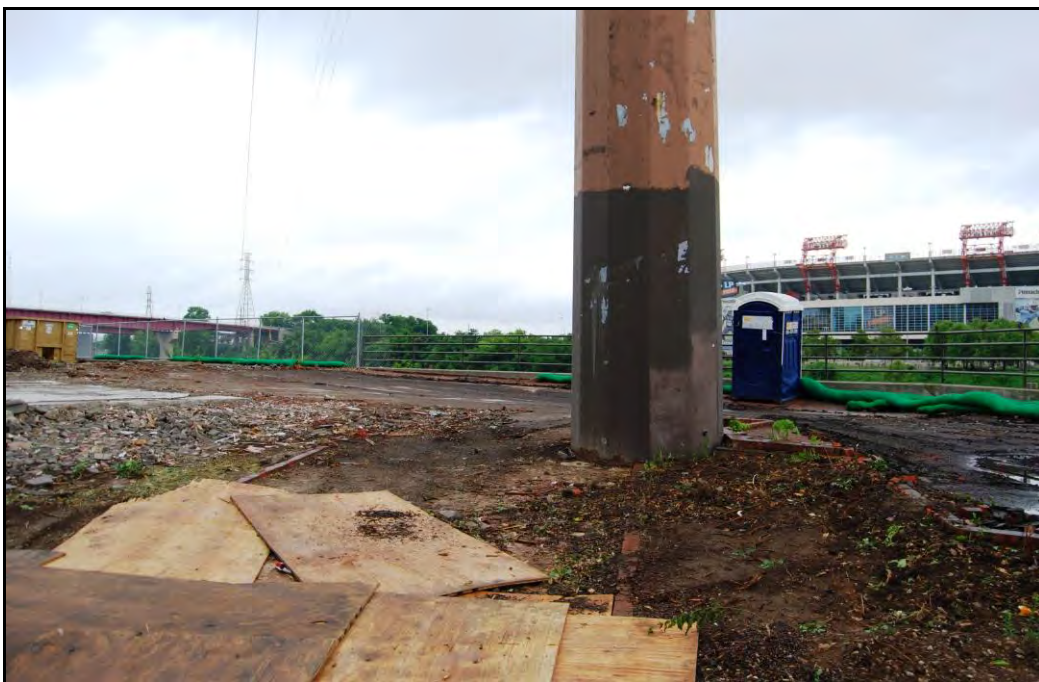
Figure 28: June 20, 2015 photograph showing clean-up after demolition of Fort Nashborough.
