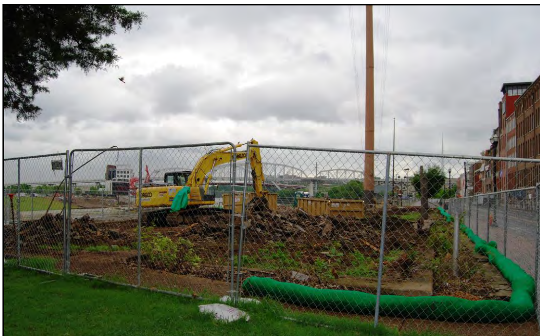
Figure 26: June 20, 2015 photograph showing clean-up after demolition of Fort Nashborough.
