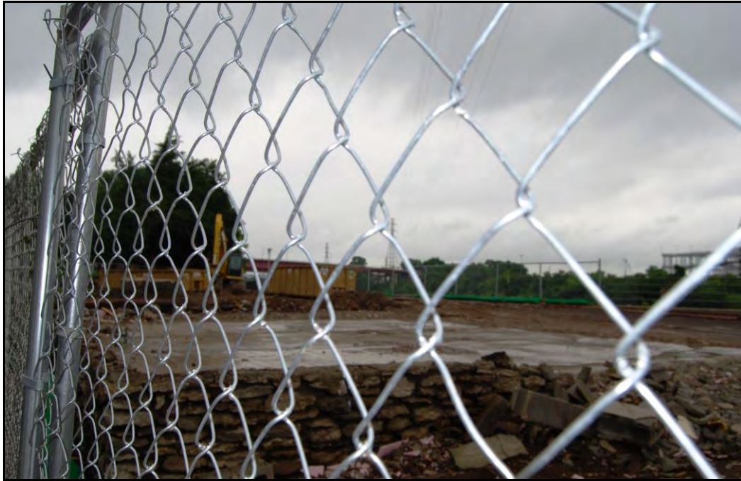
Figure 27: June 20, 2015 photograph showing clean-up after demolition of Fort Nashborough.
