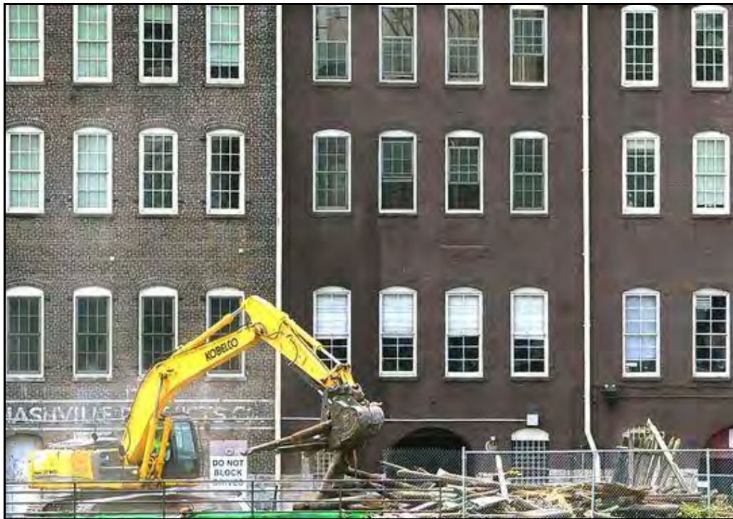
Figure 22: June 20, 2015 photograph of Fort Nashborough during demolition.
