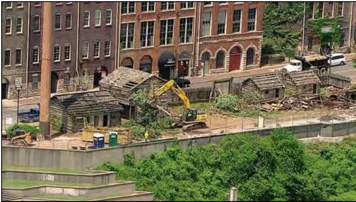
Figure 20: June 19, 2015 photograph of Fort Nashborough with demolition underway.
