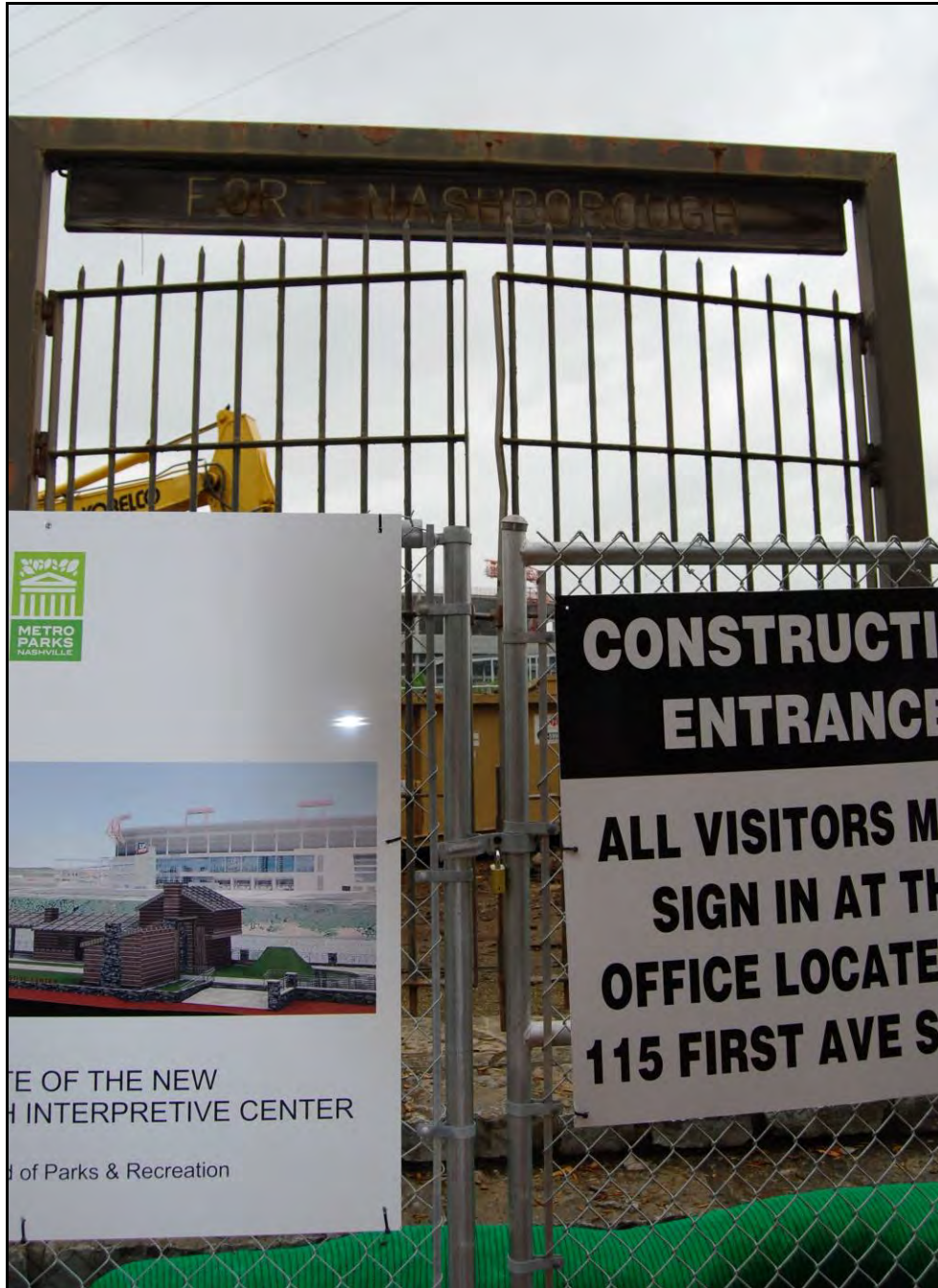
Figure 24: June 20, 2015 photograph showing clean-up after demolition of Fort Nashborough.
