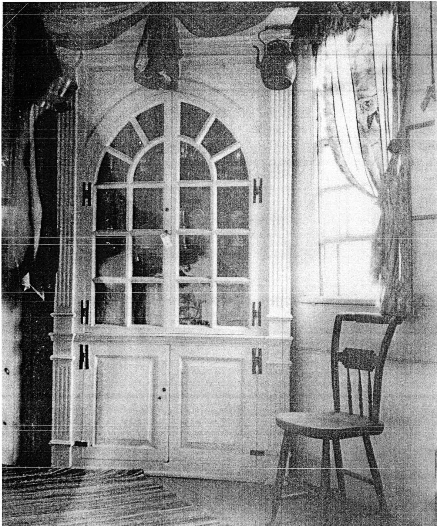
Figure 86. Corner cupboard in Room 101. Photo ca. 1920, from the WHA files. This corner cupboard is not original to Rockingham, and is currently in room 102. The paint has been stripped. This photo appears to show the original board partition still in place at Room 101.
