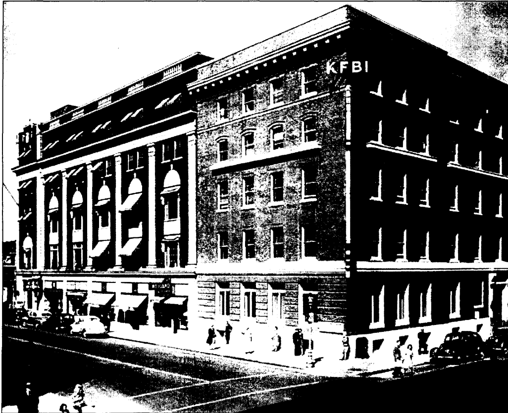
The Elks Club (left) and the Wichita Club (right) buildings circa 1943. (Wichita-Sedgwick County Metropolitan Area Planning Department)
