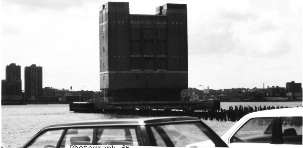
Photograph #5 Holland Tunnel New York County, NY & Hudson County, NJ New York River Ventilation Building, Looking West Robie Lange, 1992
