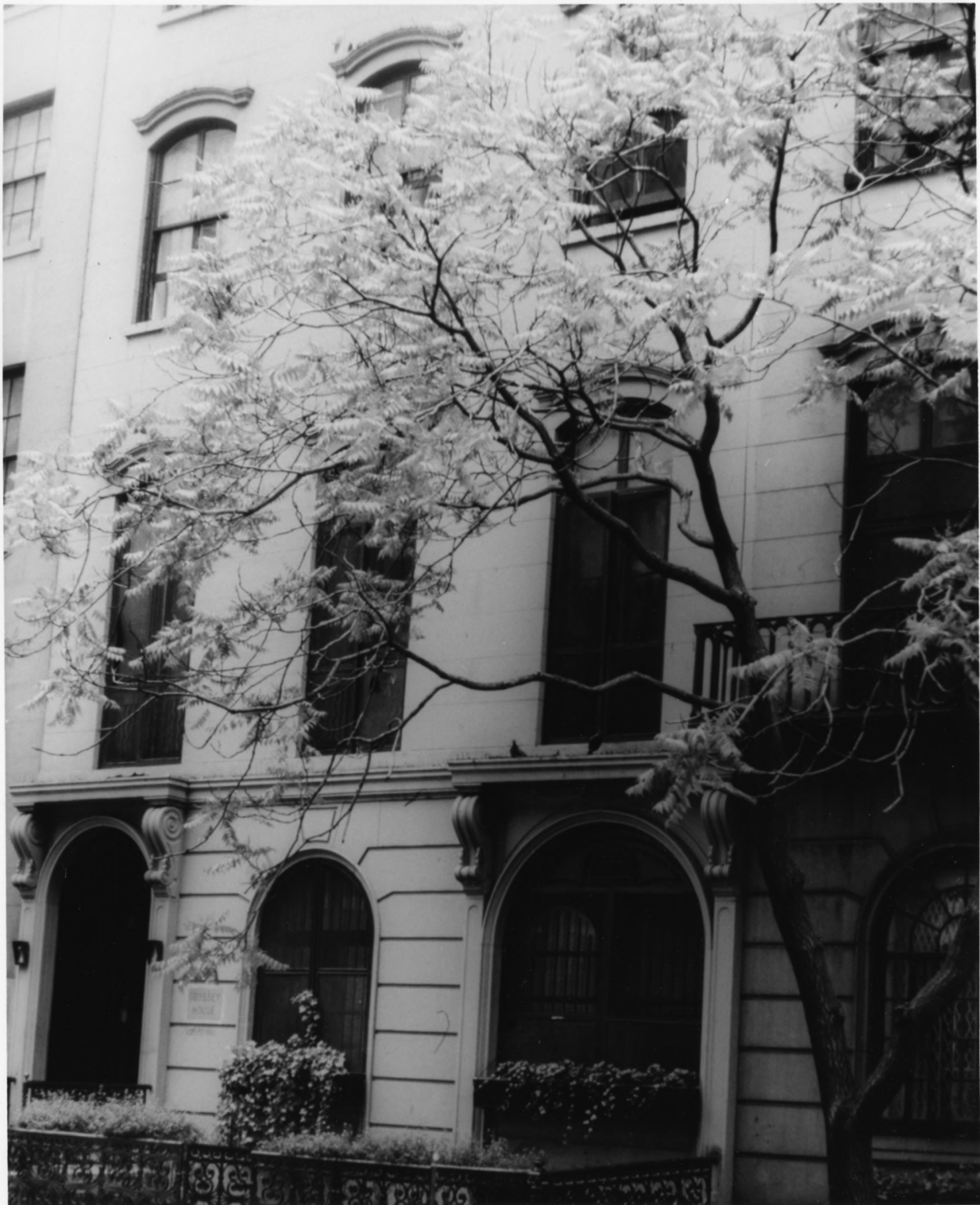
General Winfield Scott House, 24 West 12th St., N. Y., N. Y.
