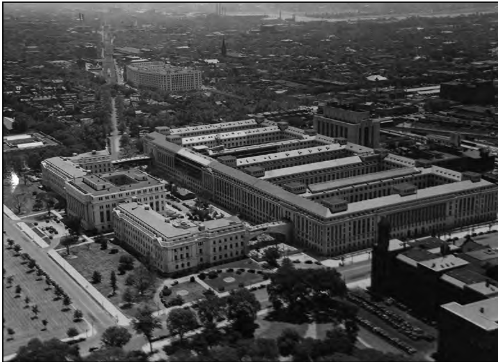
Figure 31: South Building and bridges under construction, June 1936 Source: National Agriculture Library, USDA Construction Photos
