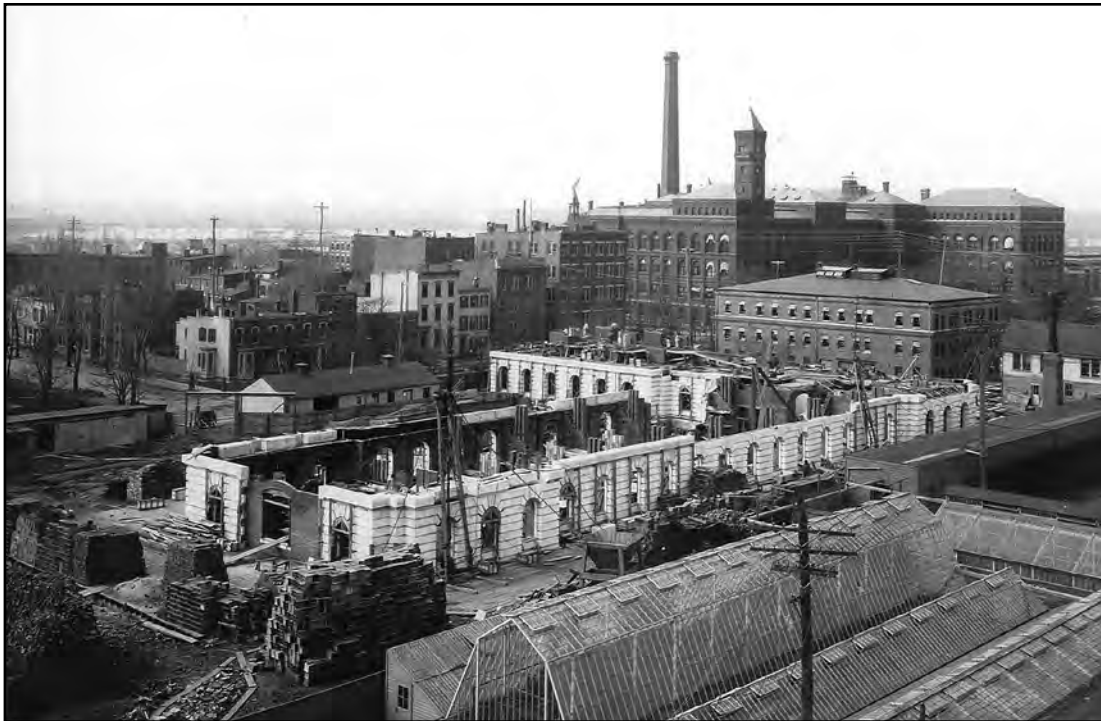
Figure 11: West Wing under construction, with surrounding buildings before demolition, March 1906 Source: National Archives Record Group 16, Records of the Office of the Secretary of Agriculture
