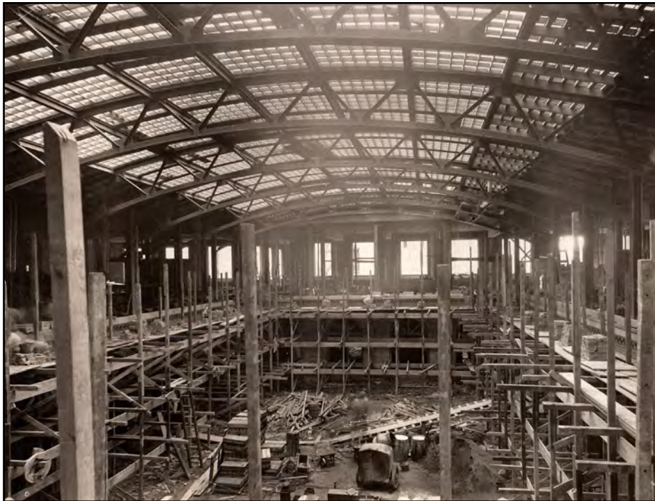
Figure 18: Courtyard under construction, July 1929. Source: National Agriculture Library, USDA Construction Photos
