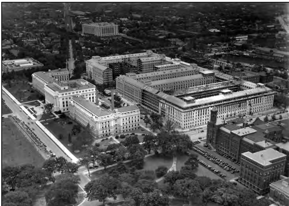
Figure 30: South Building under construction, January 1933 (note changes in Mall landscaping) Source: National Agriculture Library, USDA Construction Photos
