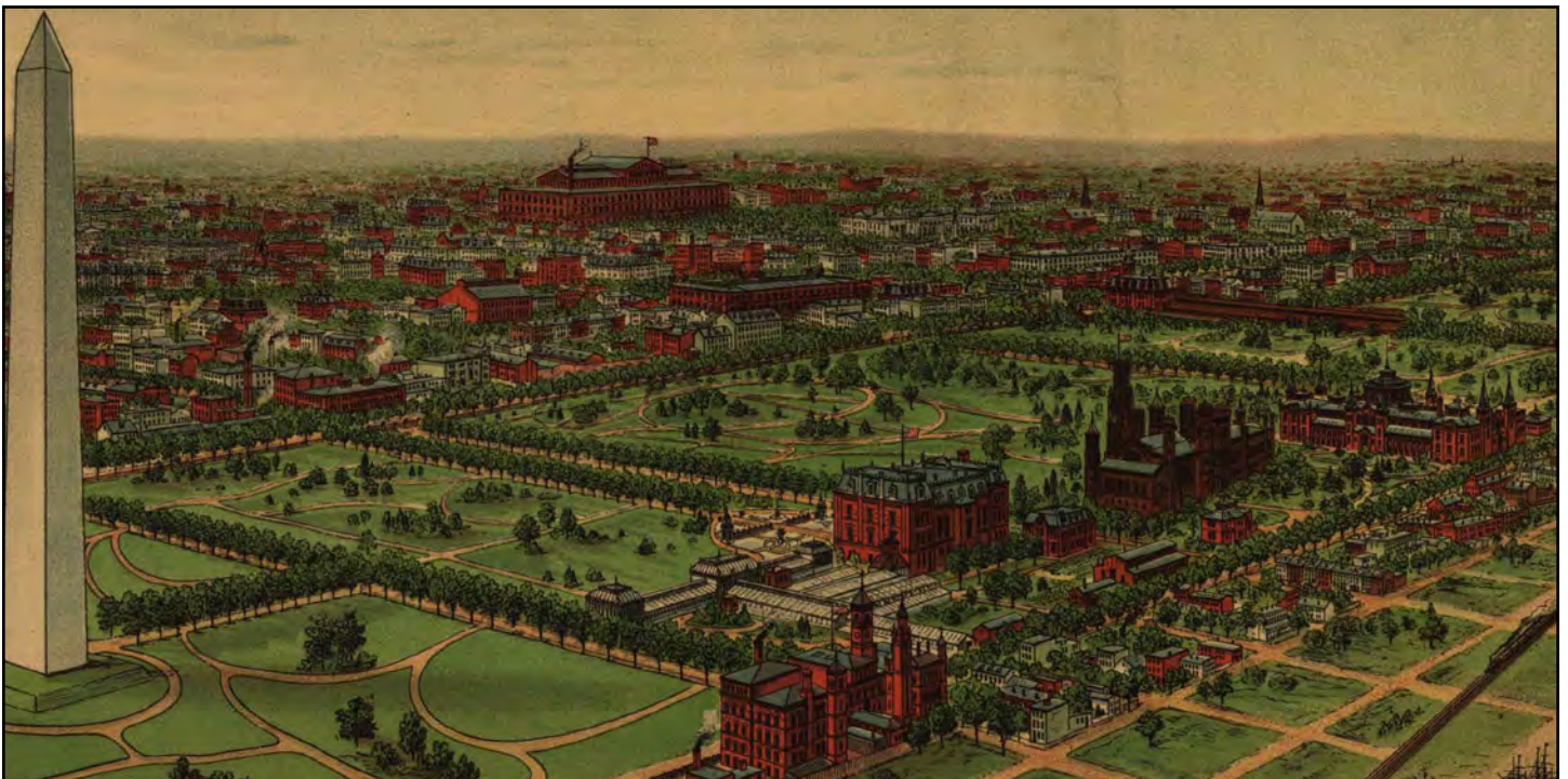
Figure 7: Panoramic view showing buildings on Agriculture Grounds, circa 1888.
