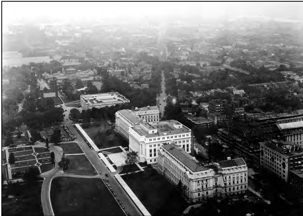
Figure 29: South Building under construction, June 1931 Source: National Agriculture Library, USDA Construction Photos
