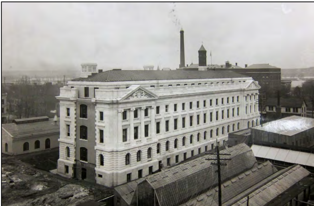
Figure 12: West Wing under construction, with surrounding buildings before demolition, circa 1907 Source: National Agriculture Library, USDA History Collection
