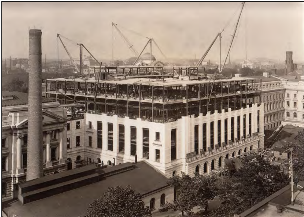
Figure 22: Center block under construction, south court, May 1929 Source: National Agriculture Library, USDA Construction Photos
