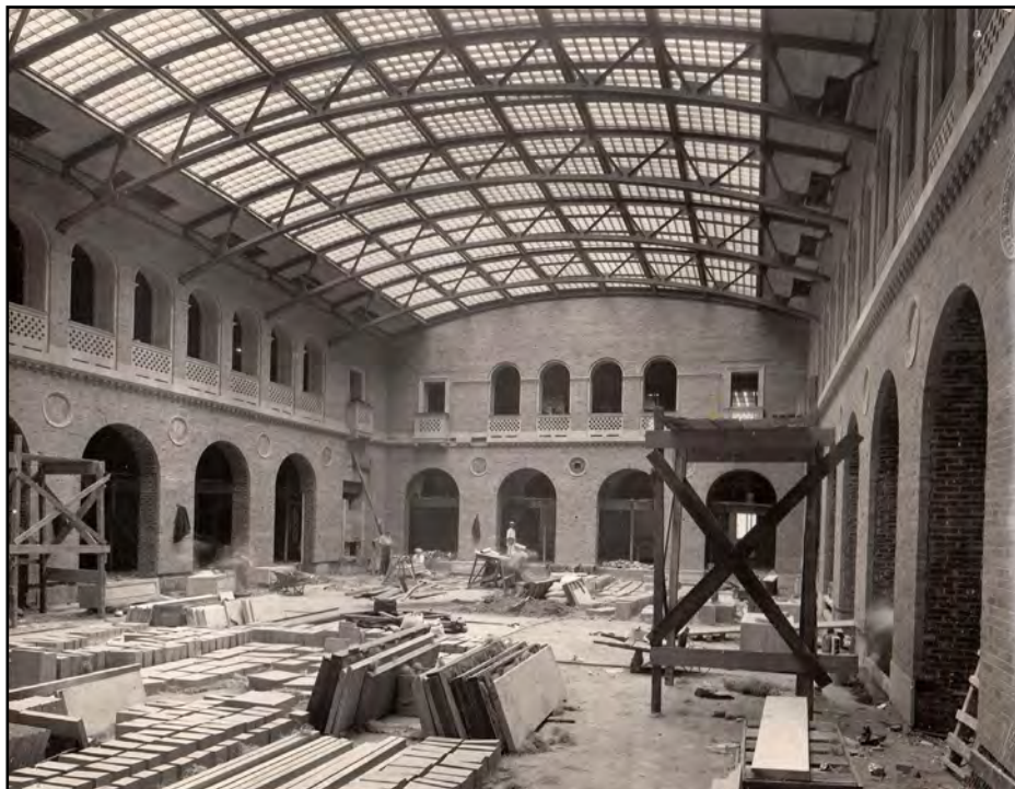
Figure 19: Courtyard under construction, September 1929. Source: National Agriculture Library, USDA Construction Photos
