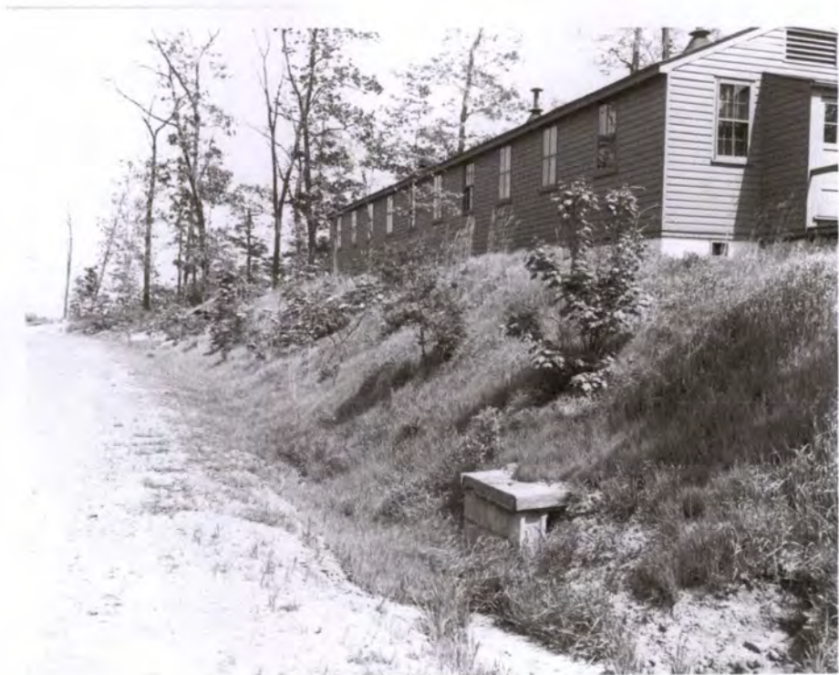
NJ_Monmouth County_Navesink Military Reservation_H62. Eastern Cantonment Barracks T-804 for 42 men, view south, c1944, GATE
