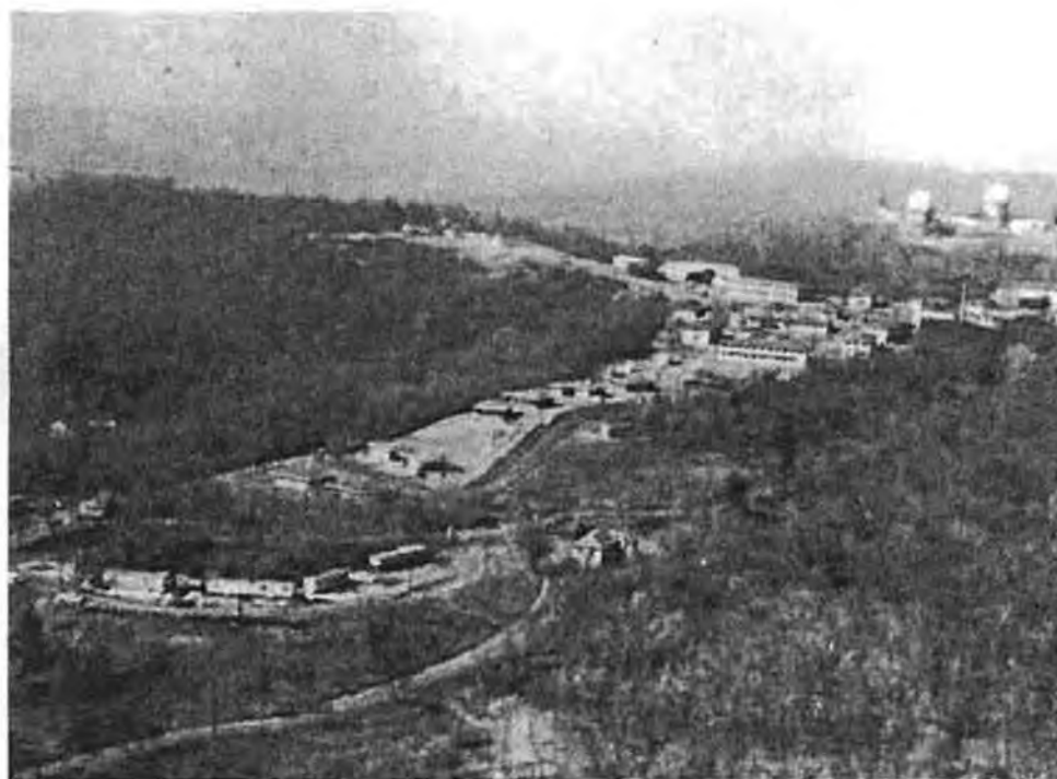
NJ_Monmouth County_Navesink Military Reservation_H82. Highlands Air Force Station, c1962, MCPS
