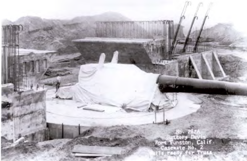
20. Construction of central traverse magazine in 1938, at Battery Richmond P. Davis. NARA Photo
