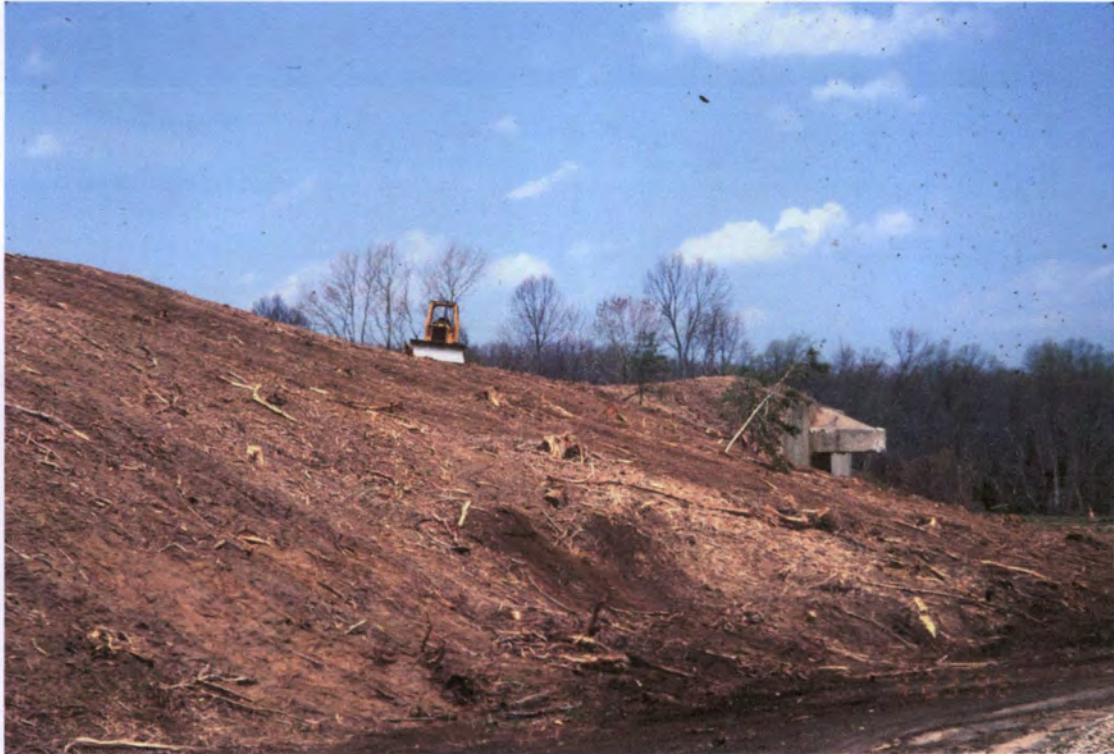
NJ_Monmouth County_Navesink Military Reservation_H89. Battery Lewis vegetation removal, 1996, MCPS
