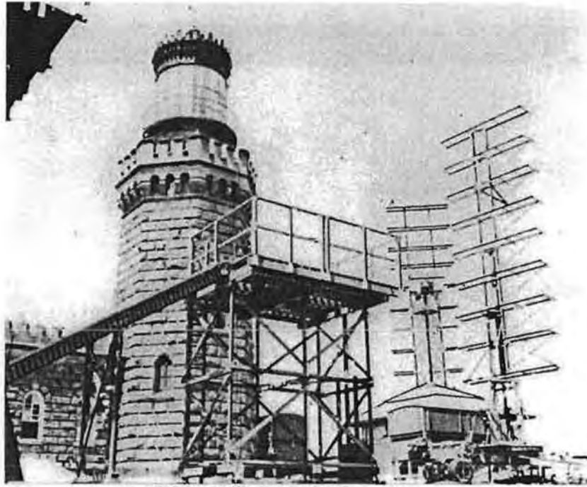
Early models of both the SCR-270 and SCR-271 installed at Twin Lights, N.J.
