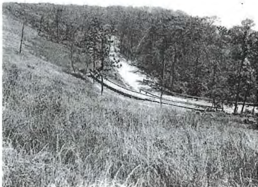
NJ_Monmouth County_Navesink Military Reservation_H64. Access Road A, Retaining Wall, view east, c1944, GATE
