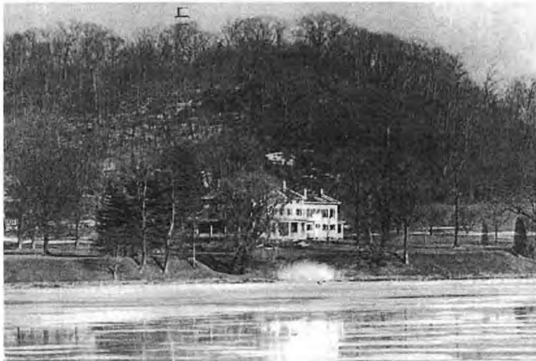
NJ_Monmouth County_Navesink Military Reservation_H60. Portland House with SCR-296 Tower, 1947-48, MCPS
