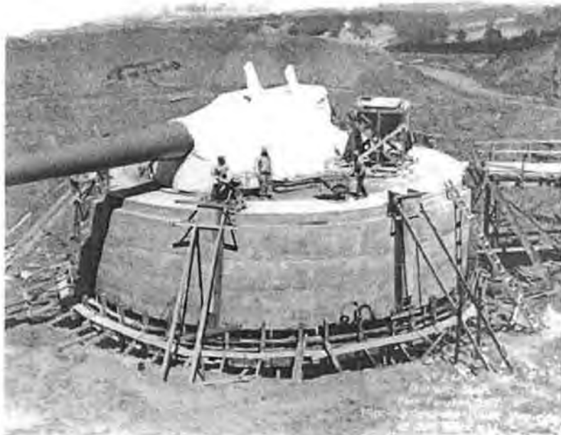
19. Gun block with 16-inch gun, Battery Richmond P. Davis, Fort Funston, HD of San Francisco. NARA Photo.
