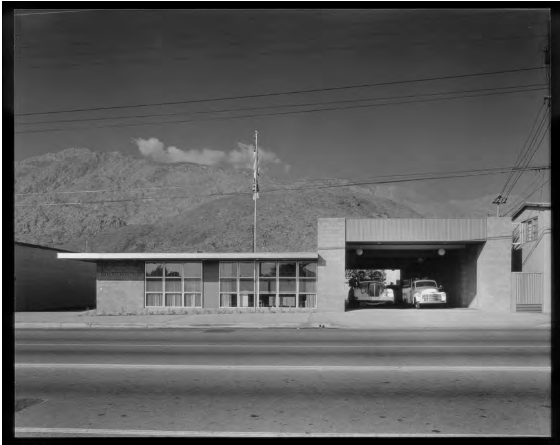
Figure 1. Primary (east) elevation, looking west, 1958.
