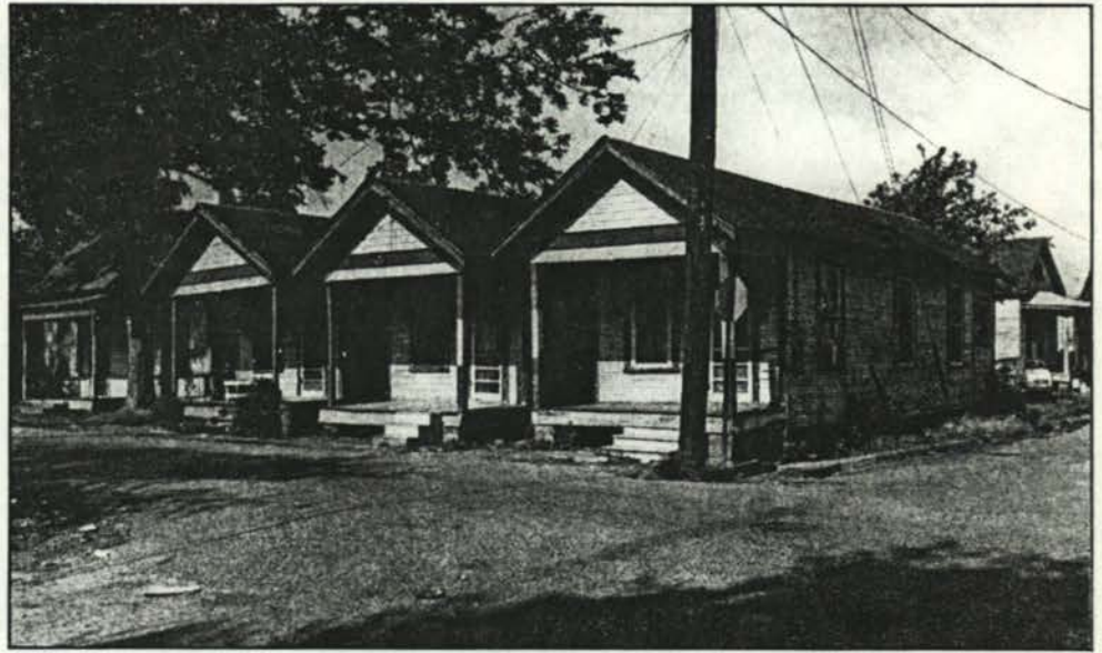
The shotgun house was a popular rental housing genre constructed in the Fourth Ward. The typical cottage has three rooms, one behind the other.
