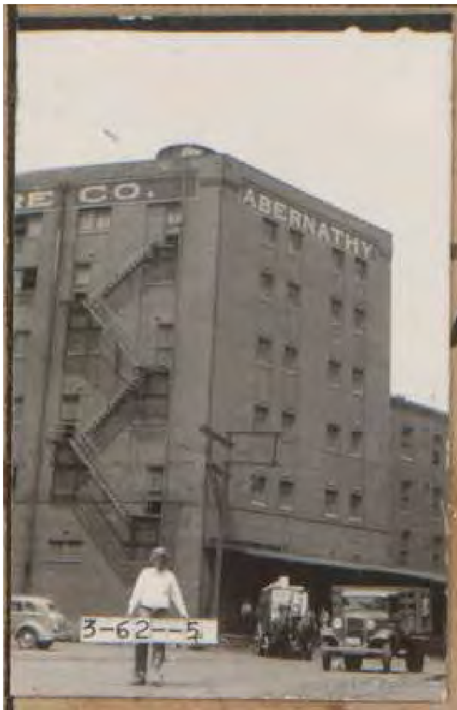
Figure 8: Abernathy Furniture Co., 910-12 Liberty St., south and east elevations, 1940. Source: Missouri Valley Special Collections, Kansas City Public Library, Kansas City, Missouri.
