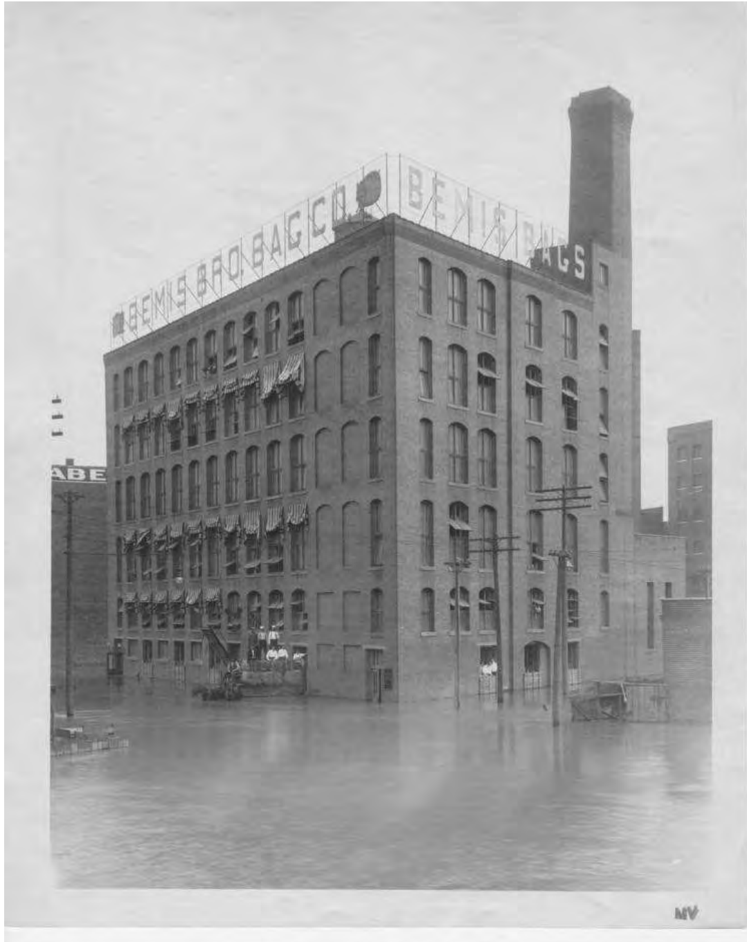
Figure 24: Bemis Bros. Bag Co., 921-29 Wyoming St., west and south elevations, 1908. Source: Missouri Valley Special Collections, Kansas City Public Library, Kansas City, Missouri.
