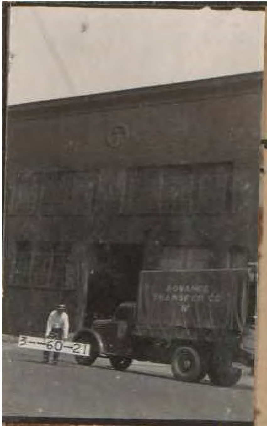
Figure 32: Advance Transfer Co. (former Samuel Freeman Livery), 1316-18 St. Louis Ave., south elevation, 1940. Source: Missouri Valley Special Collections, Kansas City Public Library, Kansas City, Missouri.
