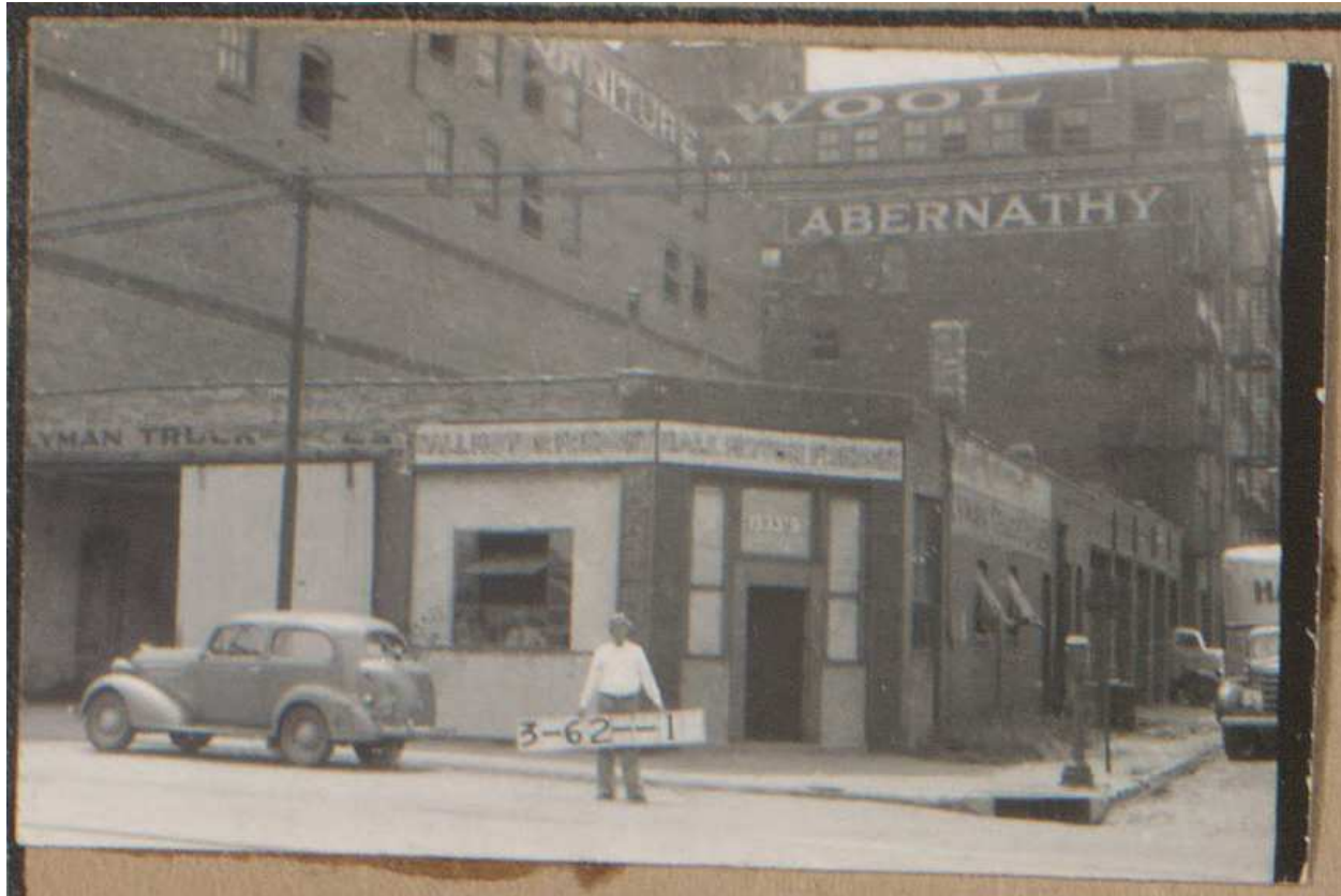
Figure 5: Abernathy Furniture Co. buildings, W. 9 th St. at Wyoming St., looking southeast, 1940. Source: Missouri Valley Special Collections, Kansas City Public Library, Kansas City, Missouri.
