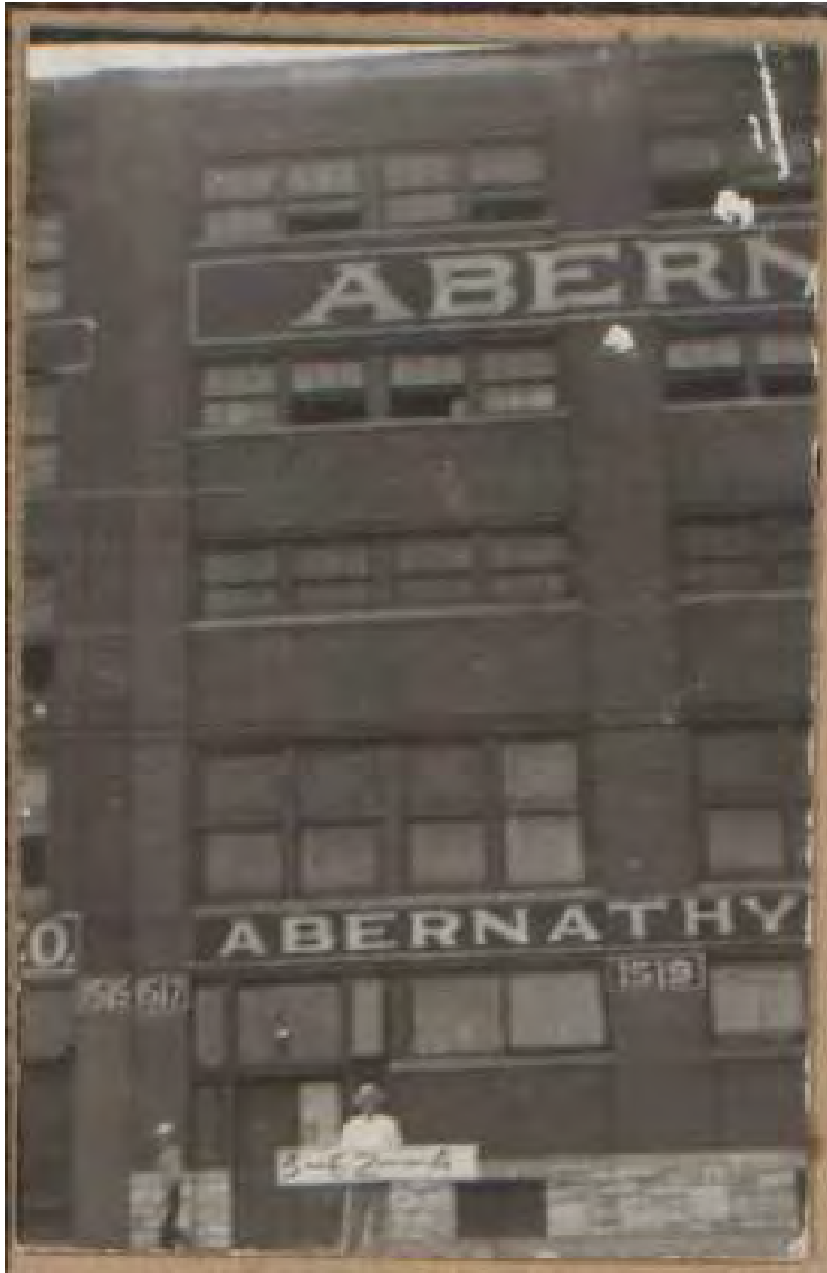
Figure 13: Abernathy Furniture Co., 1517-21 W. 9 th St., north elevation, 1940. Source: Missouri Valley Special Collections, Kansas City Public Library, Kansas City, Missouri.
