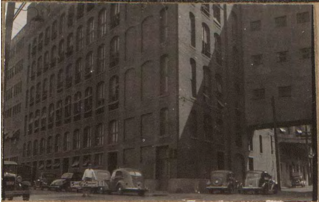
Figure 25: Bemis Bros. Bag Co., 921-29 Wyoming St., west and south elevations, 1940. Source: Missouri Valley Special Collections, Kansas City Public Library, Kansas City, Missouri.
