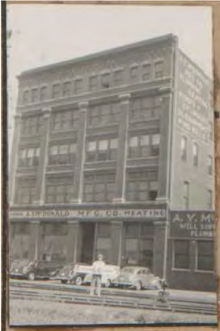
Figure 38: A. Y. McDonald Manufacturing Co. (former Geiser Manufacturing Co.), 1408-12 Union Ave., south and east elevations, 1940. Source: Missouri Valley Special Collections, Kansas City Public Library, Kansas City, Missouri.
