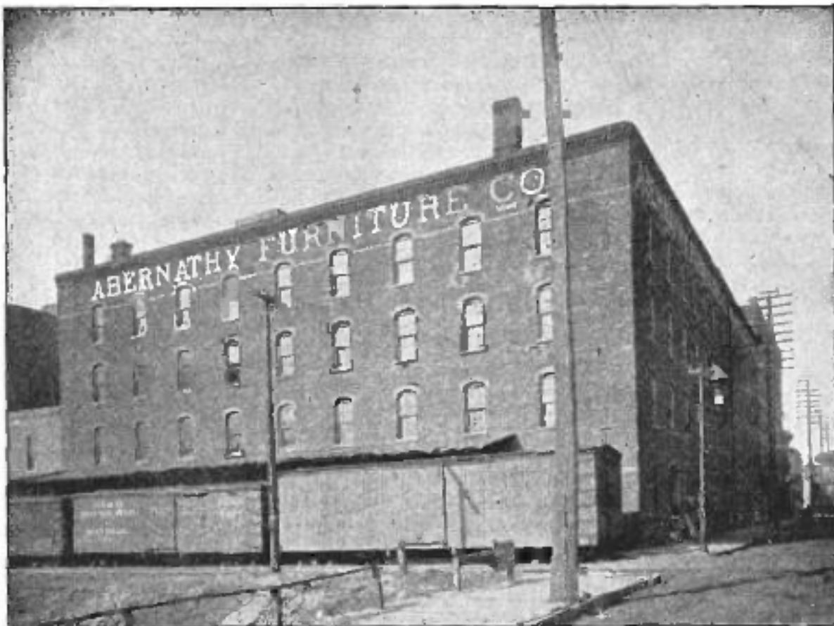
Figure 10: Abernathy Furniture Co., southwest corner of Liberty and W. 9 th Streets, east and north elevations. Source: Pen and Sunlight Sketches of Kansas City and Environs, 1892.
