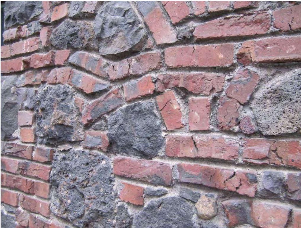
7 of 36 clinker brick and basalt rock rubblemix in 2013
