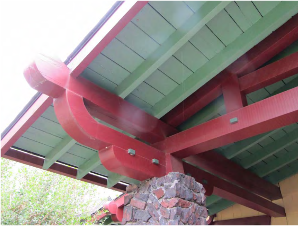
6 of 36 front porch mortise-and-tenon detail in 2013
