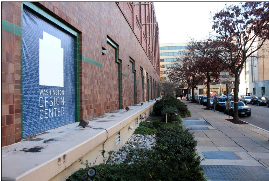
Photo #0006: DC_Terminal Refrigerating & Warehousing Co Bldg_0006.tif Exterior; detail of loading dock platform on north elevation, camera facing west
