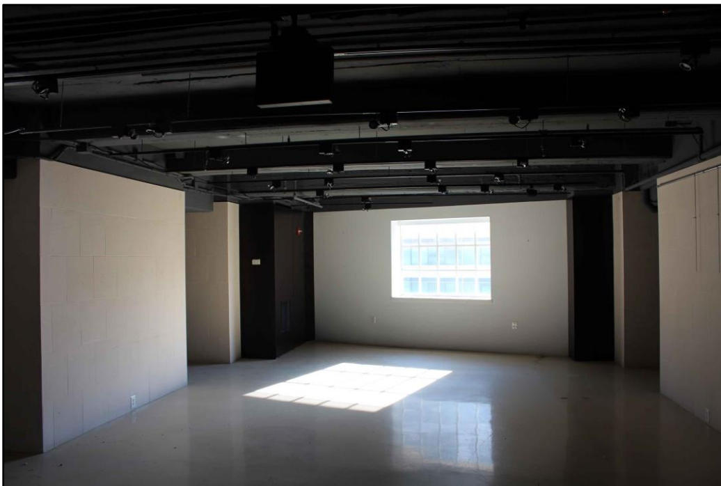
Photo #0010: DC_Terminal Refrigerating & Warehousing Co Bldg_0010.tif Interior; typical former dry storage room/design showroom, camera facing south
