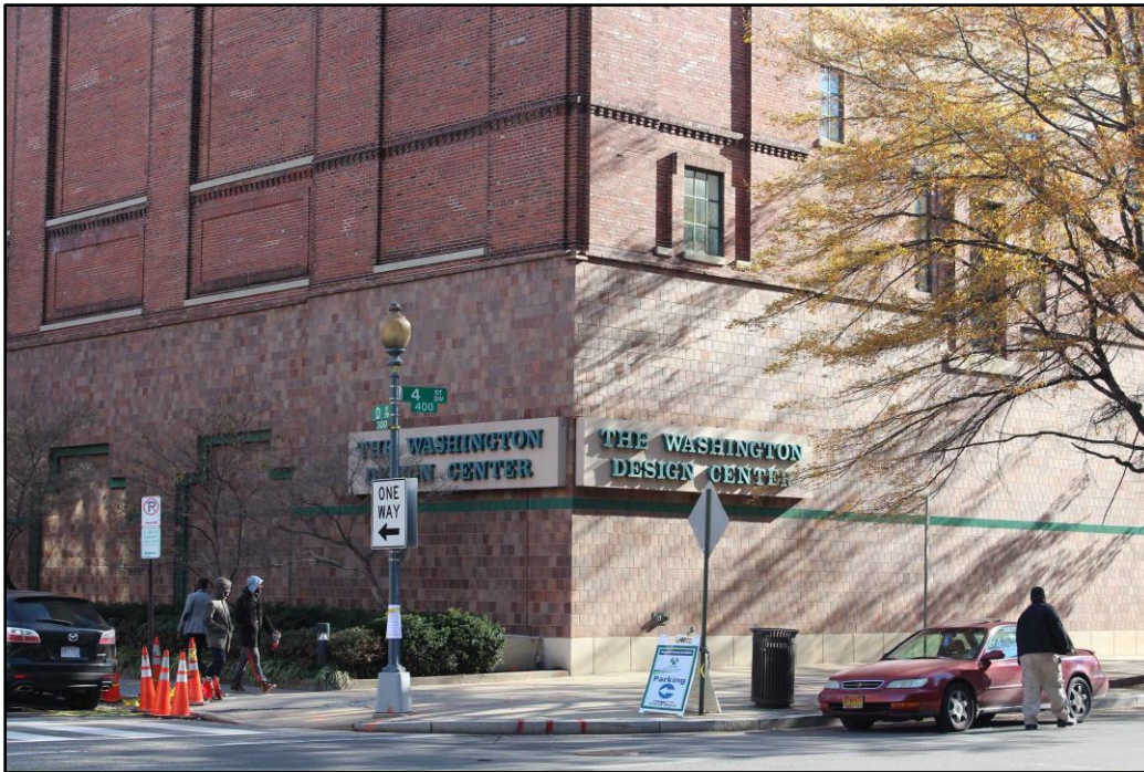
Photo #0007: DC_Terminal Refrigerating & Warehousing Co Bldg_0007.tif Exterior; detail of signage on northwest corner, camera facing southeast
