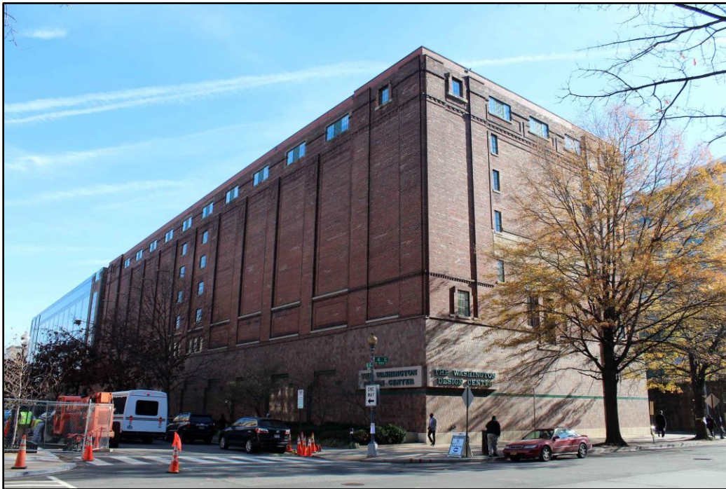
Photo #0001: DC_Terminal Refrigerating & Warehousing Co Bldg_0001.tif Exterior; north (left) and west (right) elevations, camera facing southeast
