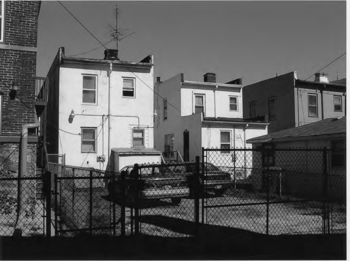
Polk Street Concrete Cottages H.D., Lake Co., IN #7
