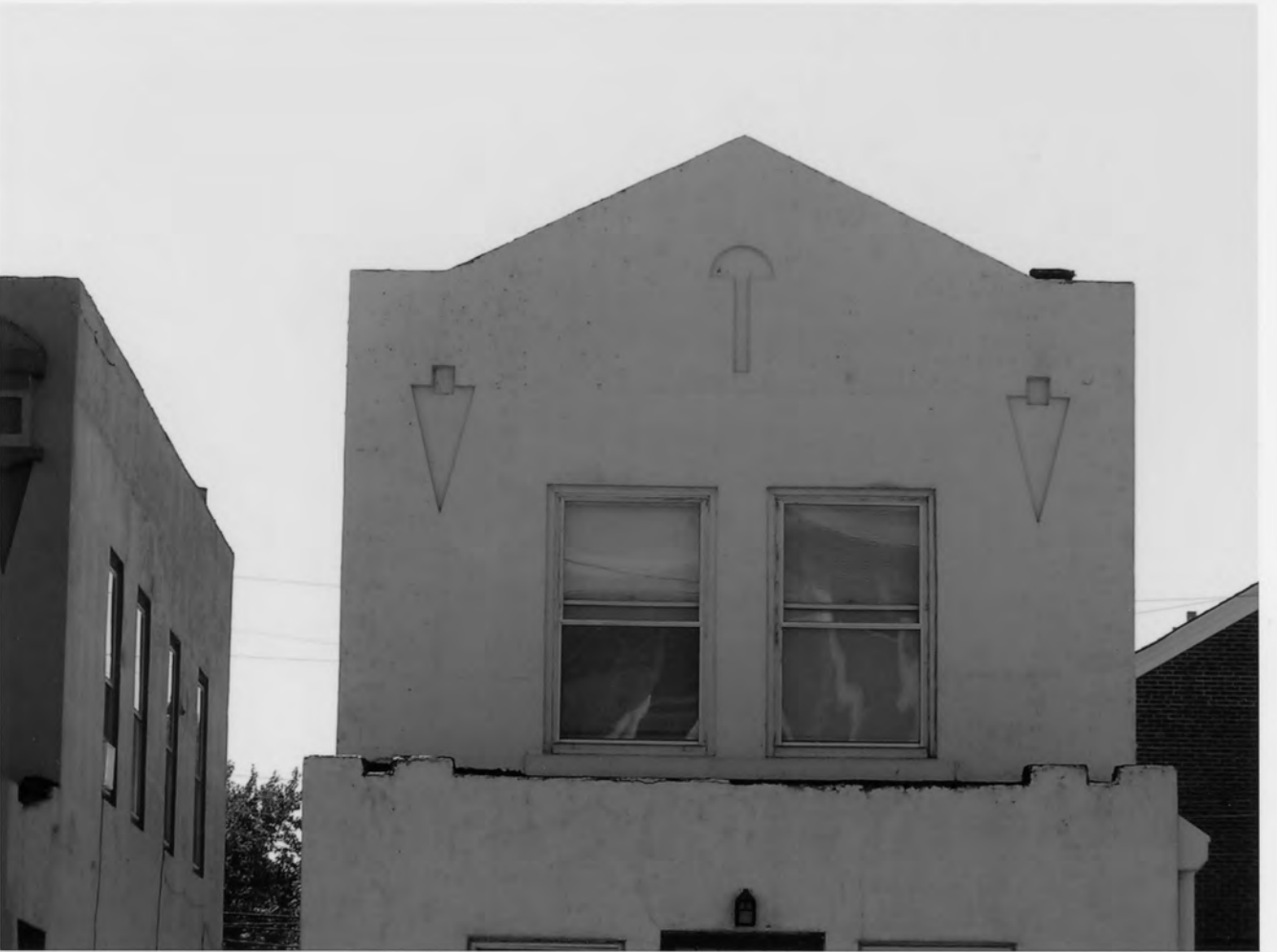
Polk Street Concrete Cottages H.D., Lake Co., IN #10
