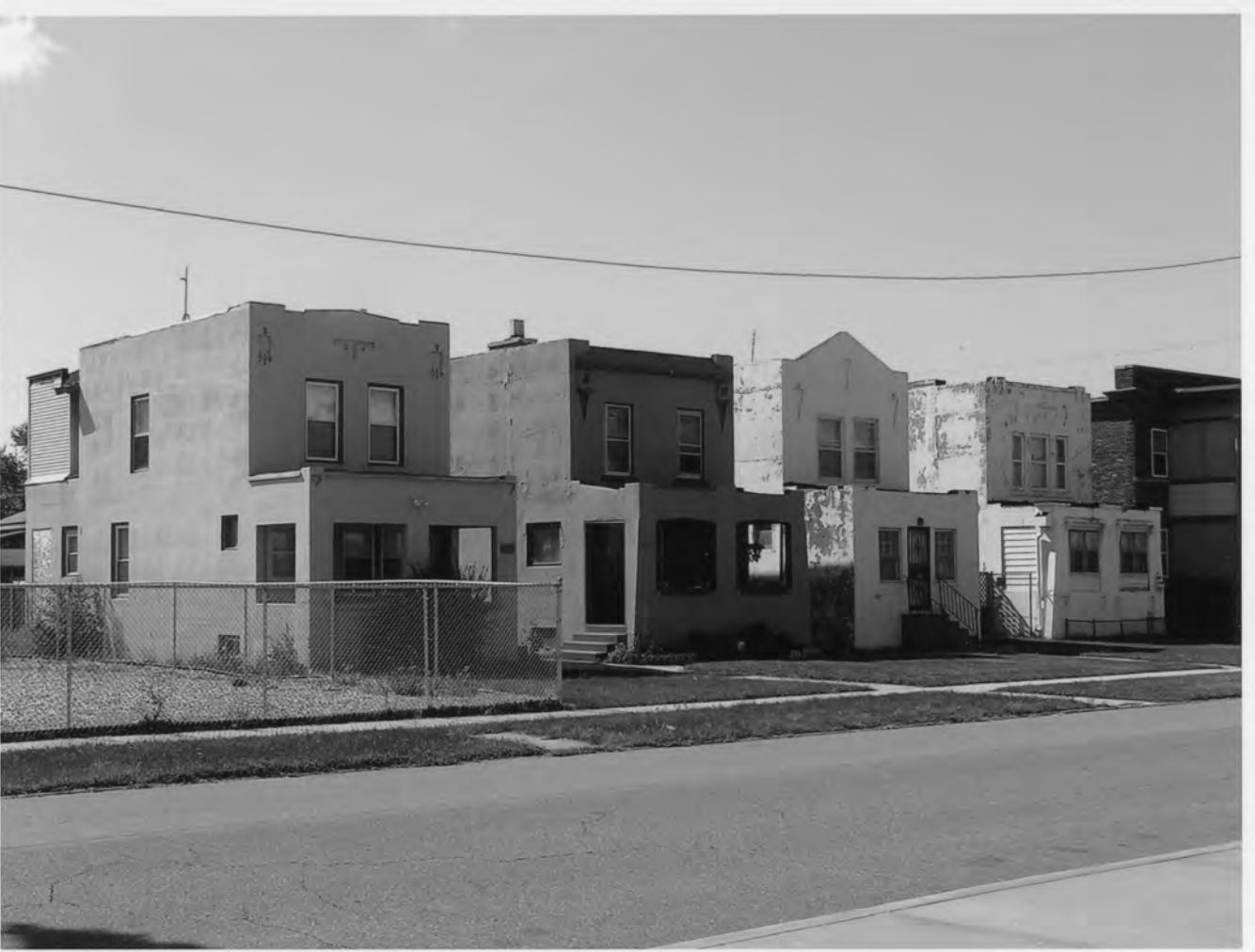
Polk Street Concrete Cottages H.D., Lake Co., IN #1
