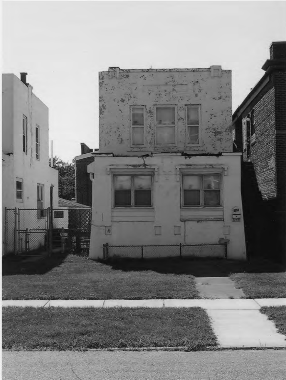
Polk Street Concrete Cottages H.D., Lake Co., IN #3
