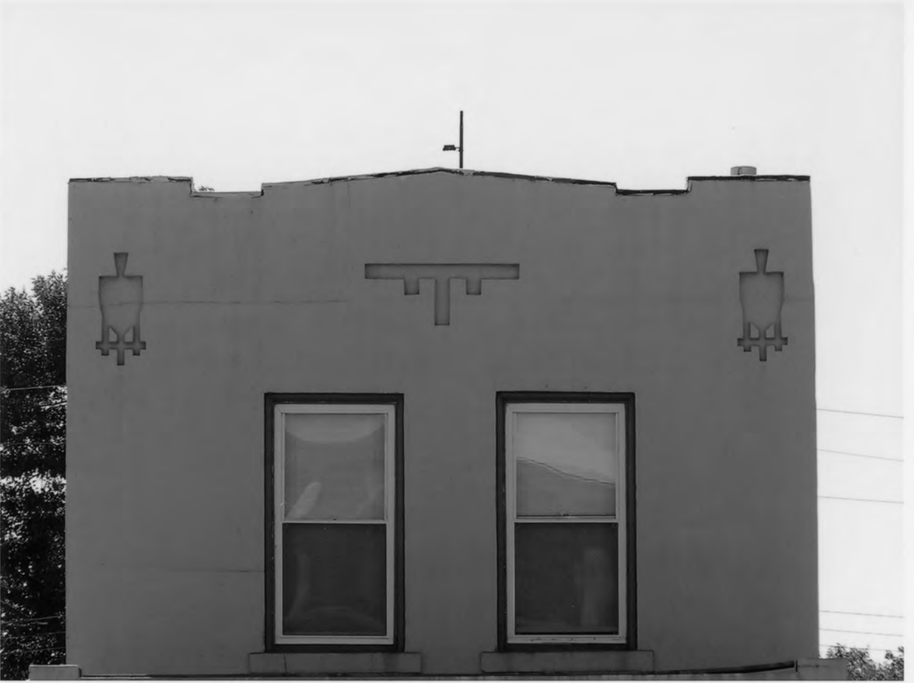
Polk Street Concrete Cottages H.D., Lake Co., IN #9
