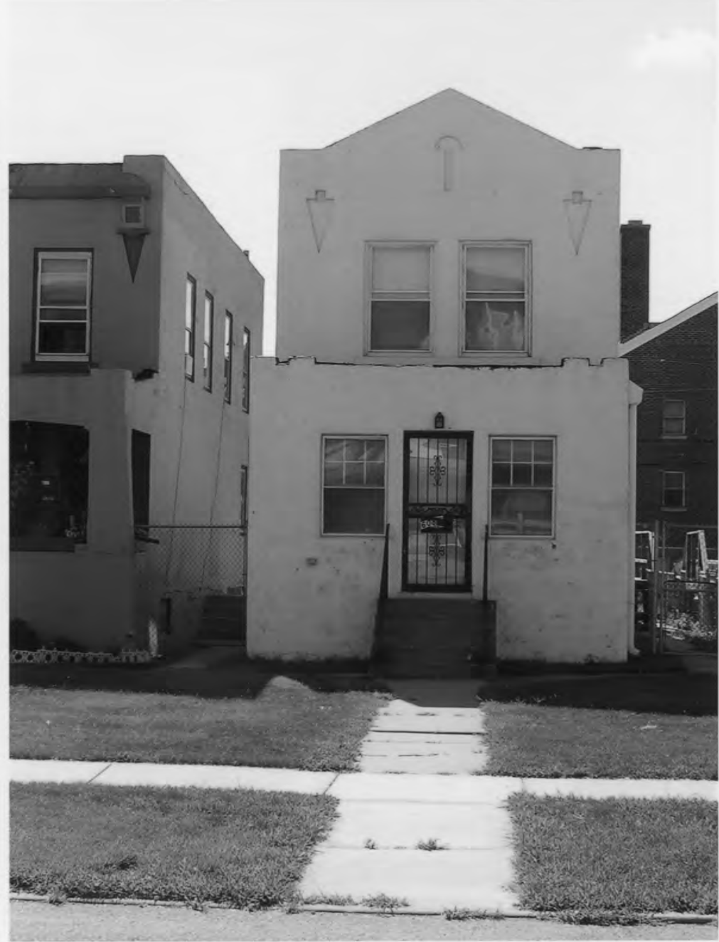
Polk Street Concrete Cottages H.D., Lake Co., IN #4
