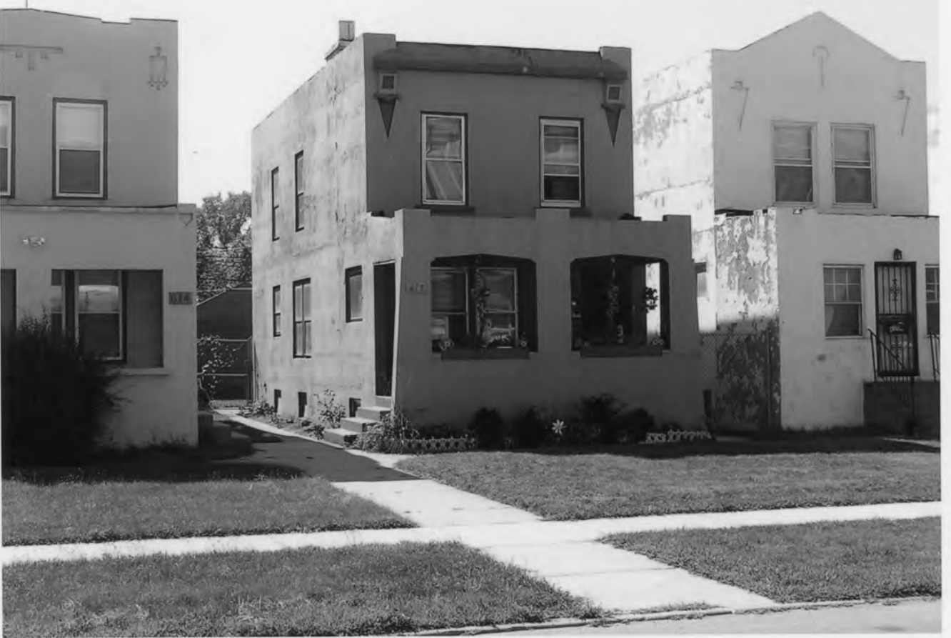
Polk Street Concrete Cottages H.D., Lake Co., IN #5
