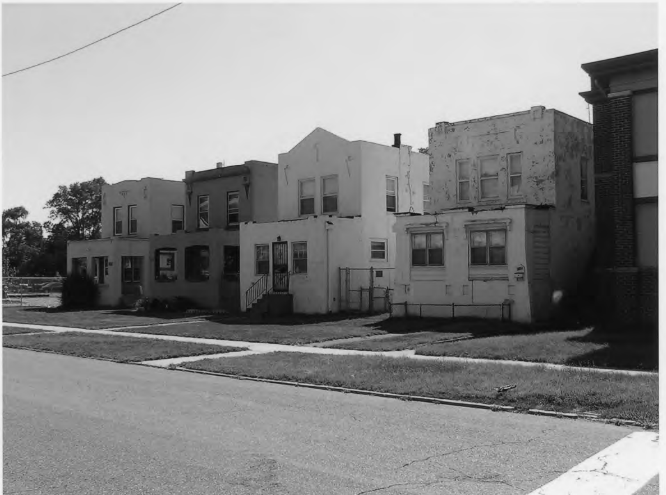
Polk Street Concrete Cottages H.D., Lake Co., IN #2
