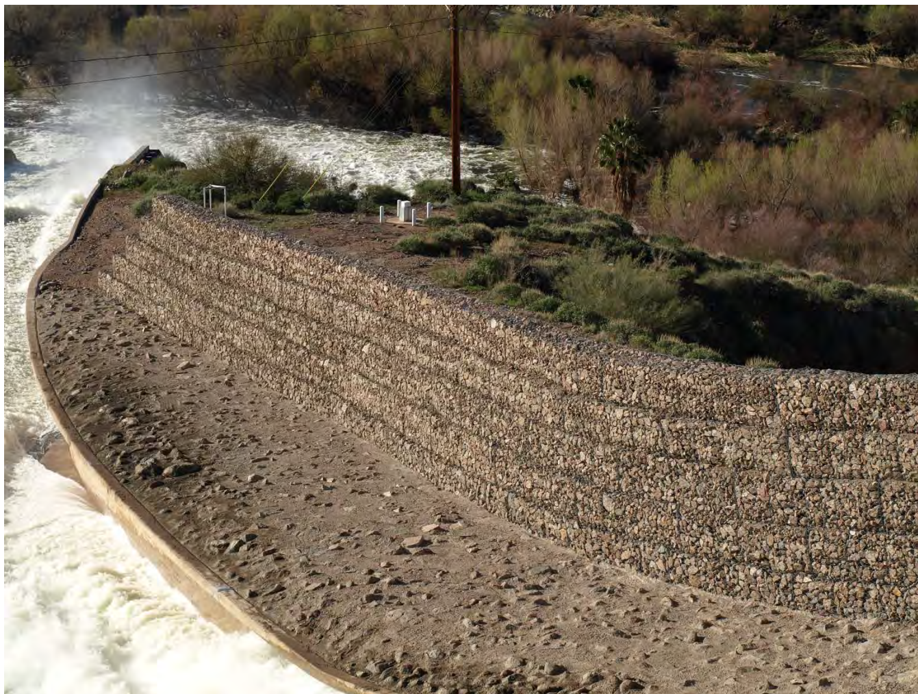
Photo 8. Stewart Mountain Dam spillway training wall looking south.
