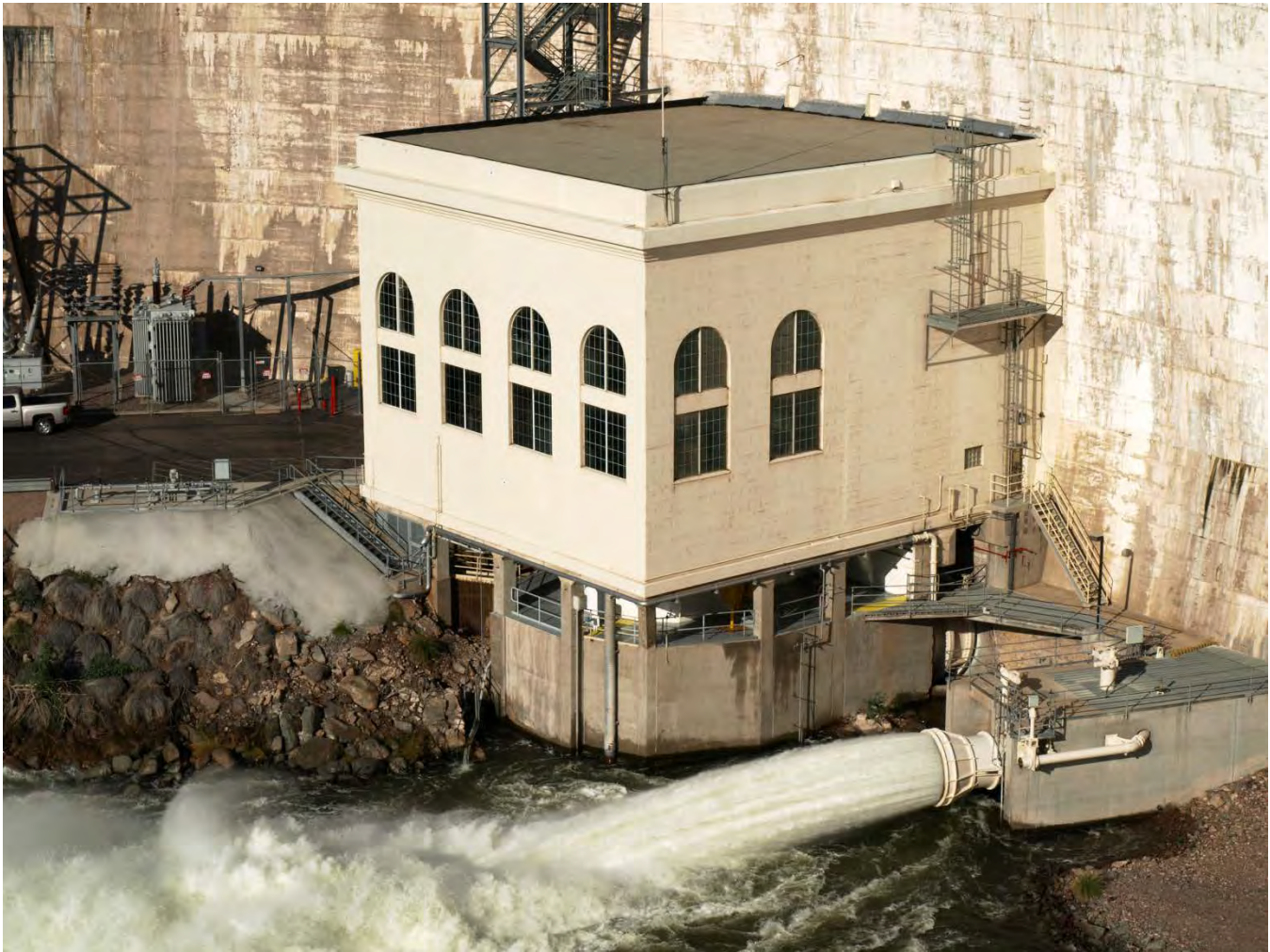
Photo 6. Stewart Mountain Dam powerhouse and river outlet looking west from the left abutment.
