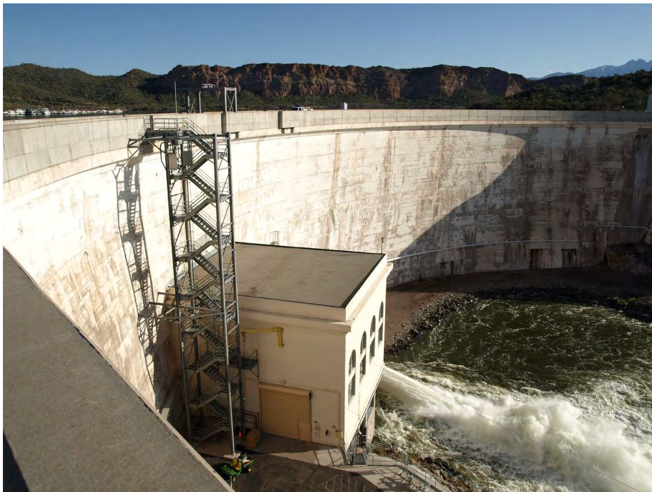
Photo 3. Stewart Mountain Dam arch section and powerhouse looking northeast.
