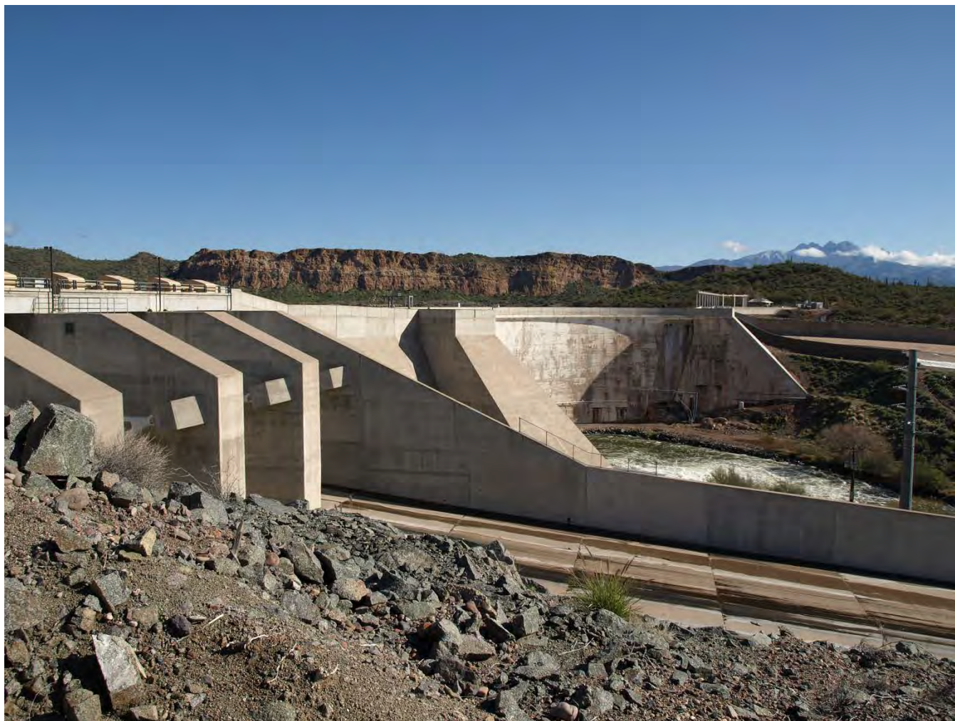
Photo 2. Stewart Mountain Dam looking northeast from the right abutment.
