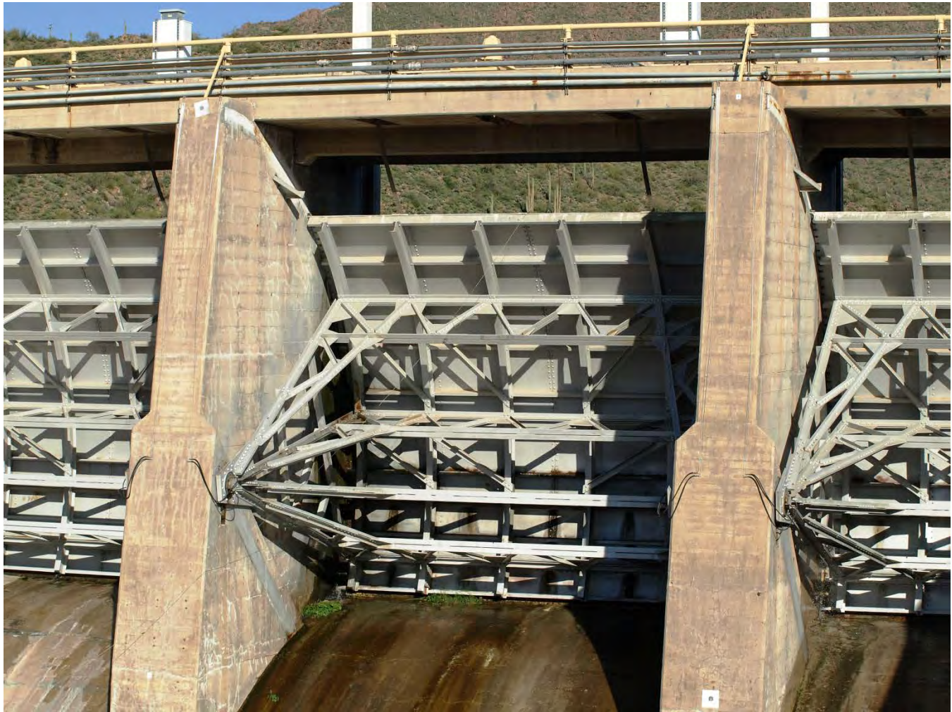
Photo 9. Stewart Mountain Dam spillway gate detail.
