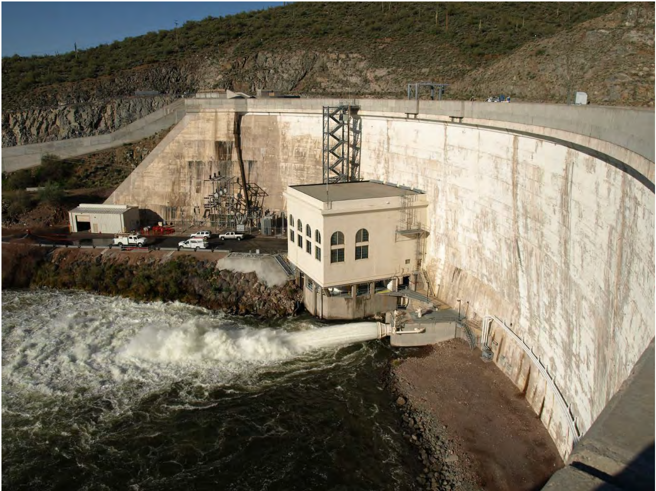
Photo 5. Stewart Mountain Dam looking west from the left abutment.
