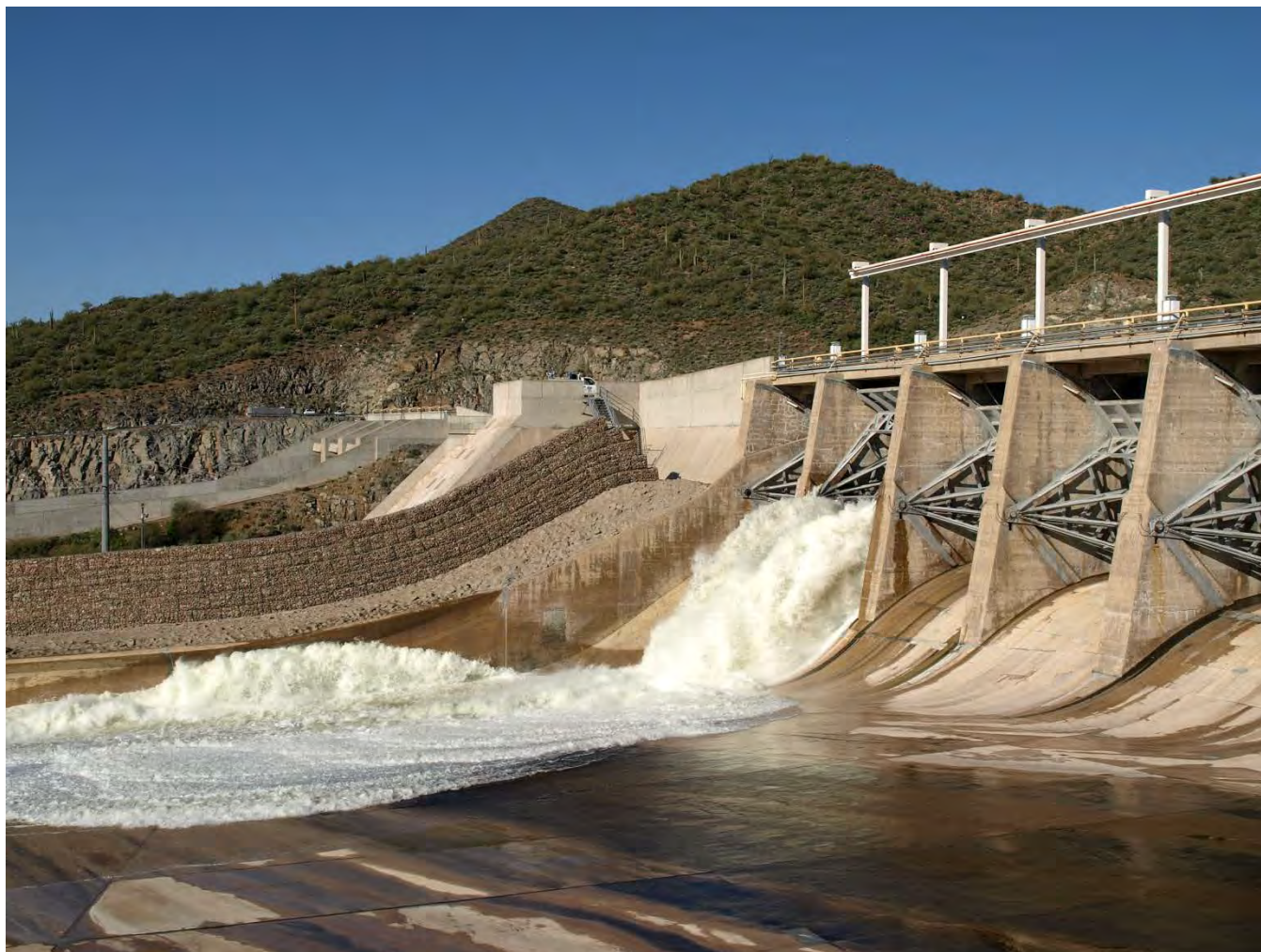
Photo 7. Stewart Mountain Dam historic spillway looking west from the left abutment.
