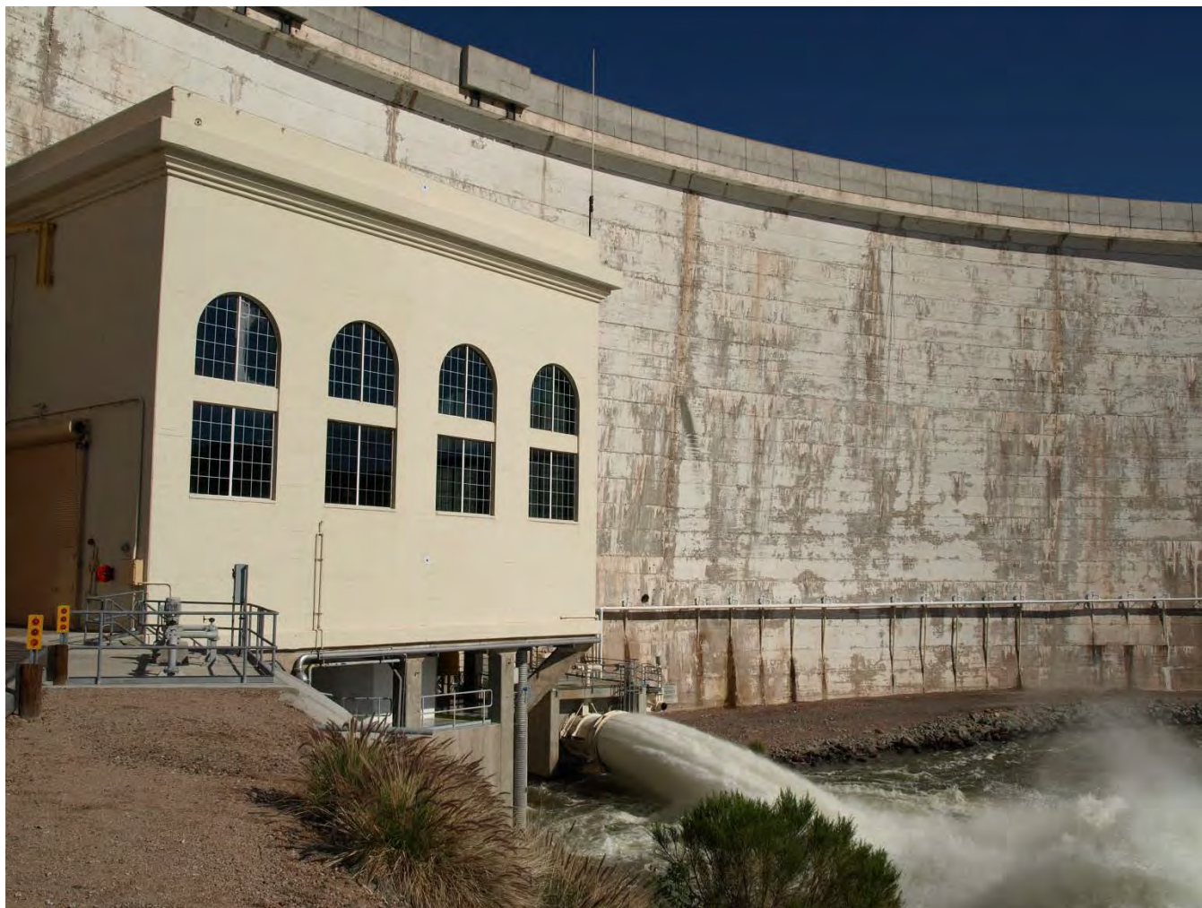
Photo 4. Stewart Mountain Dam powerhouse looking north-northeast.
