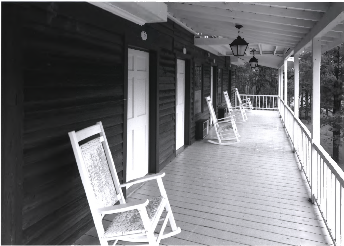
Glen-Ella Springs Hotel Clarksville, Habersham County, Georgia #10 of 13
