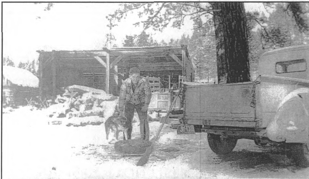
Looking north towards the combination blacksmith shop/woodshed. Note the log building adjacent to the left, which was removed in order to build the sauna.
